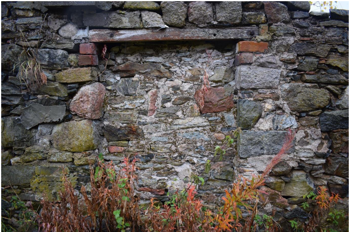
Illus 7 Room 5 blocked door D3; facing NNW
