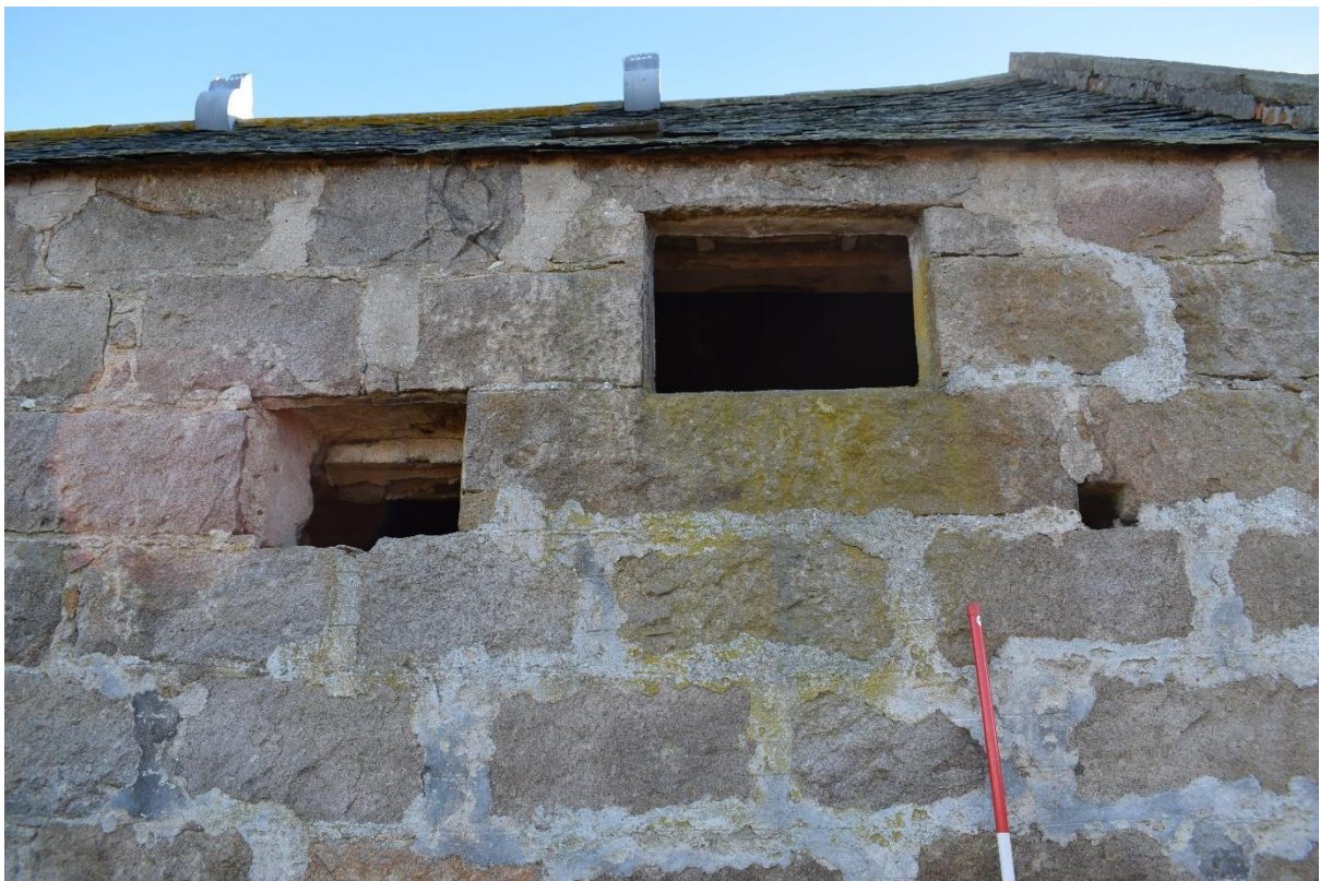
Illus 5 Building 1 W wall W2 (left) W1 (right); facing E
