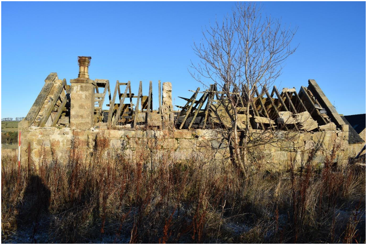
Illus 13 Building 2 S wall; facing N
