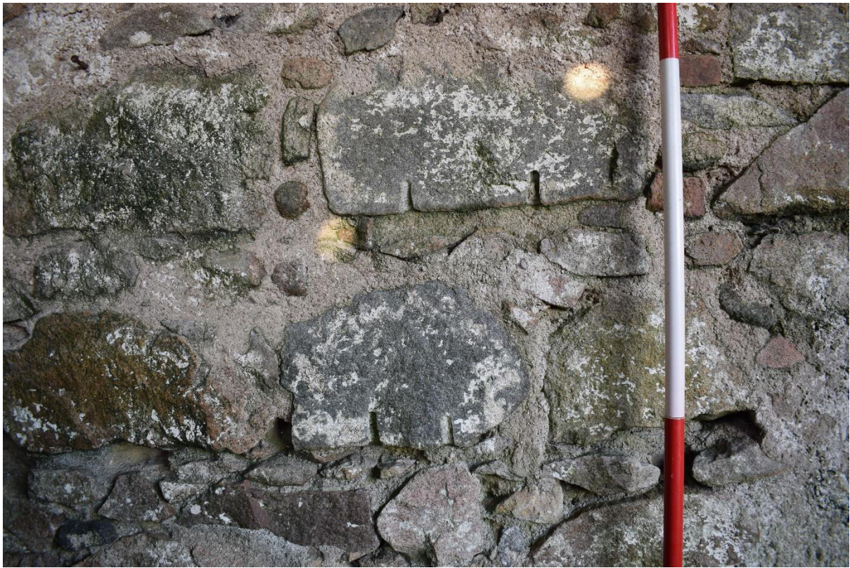
Illus 8 Building 1 N wall showing drilled granite blocks; facing N
