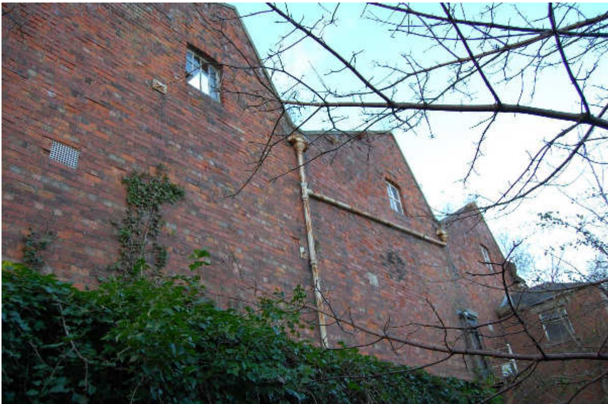
Illus 98 Building 83 E gable; facing NW
