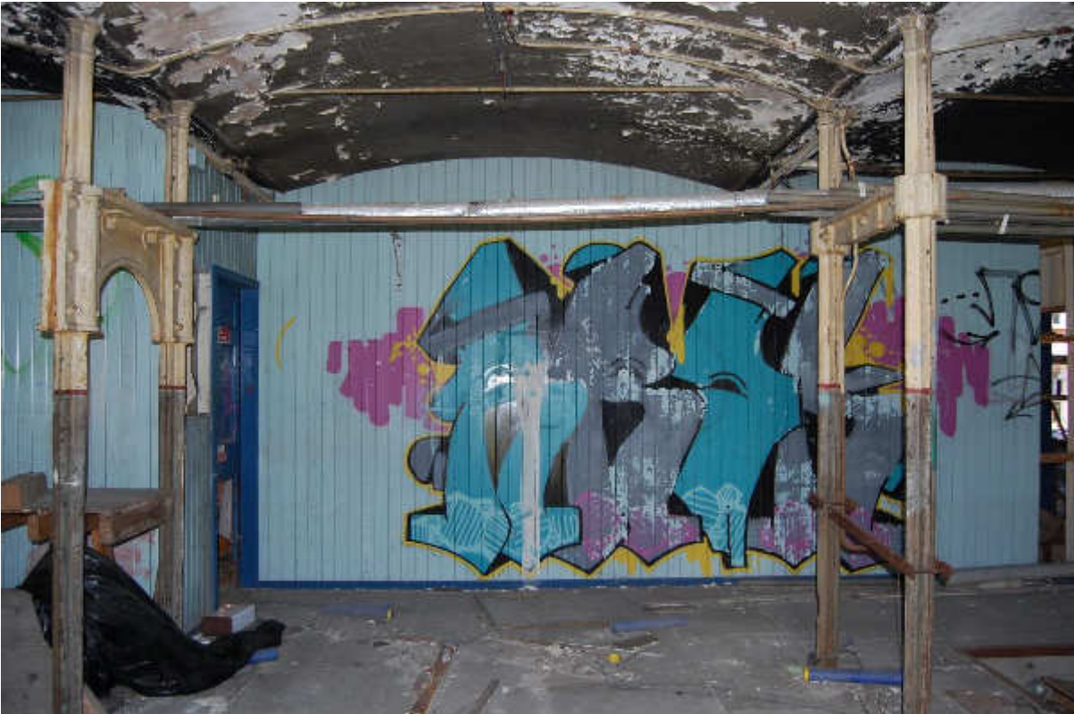
Illus 64 Building 45 cruciform cast iron pillars and arched brick ceiling
