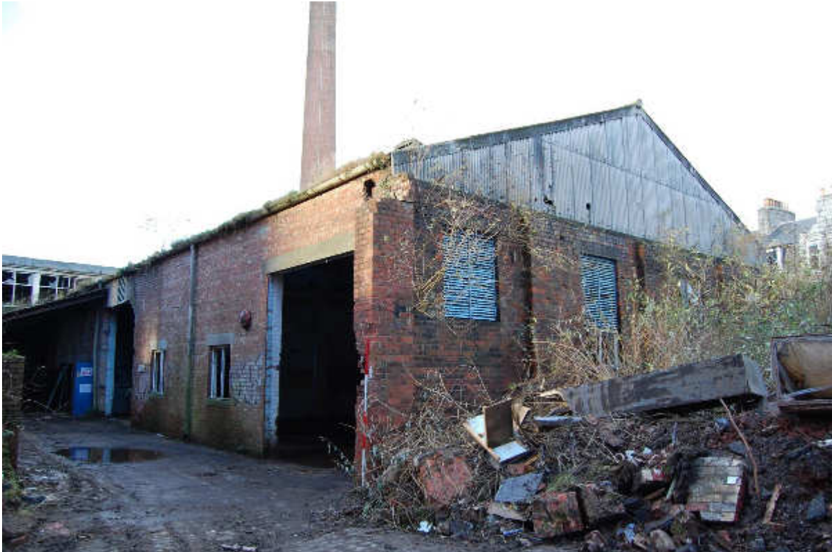
Illus 72 Building 52 SE corner showing area of demolished S wall (left); facing NW
