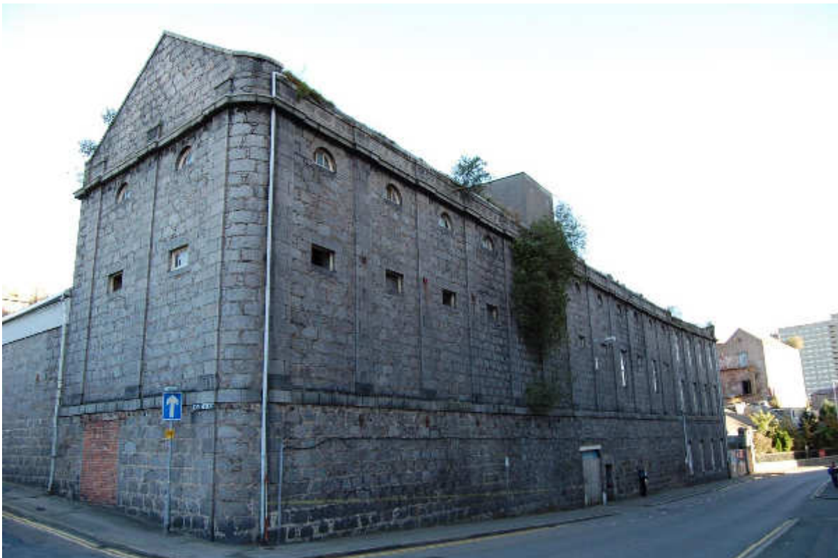
Illus 14 Ann St/Maberly St junction with Building 5 (left) Buildings 64, 4, 4A (right) showing brick-blocked door D5/1 (left); facing NE
