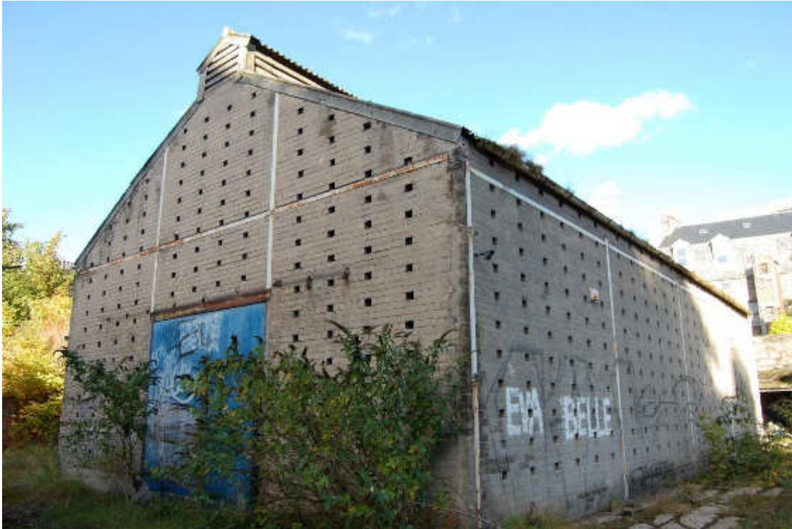
Illus 122 Building 92; facing NNE.
