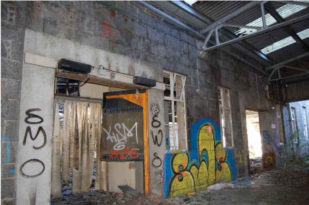
Illus 42 Building 30 E façade D30/1, W30/2, /3, D30/4 (L-R); facing NNW
