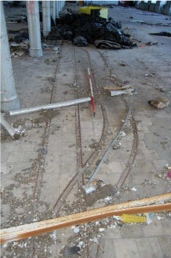
Illus 108 Building 84 first floor cart tracks passing place; facing NNW
