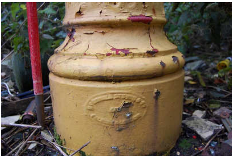
Illus 143 Detail of maker's mark, 'McDowall Steven & Co/Falkirk & ?', cast iron lamp stand F29; facing WSW
