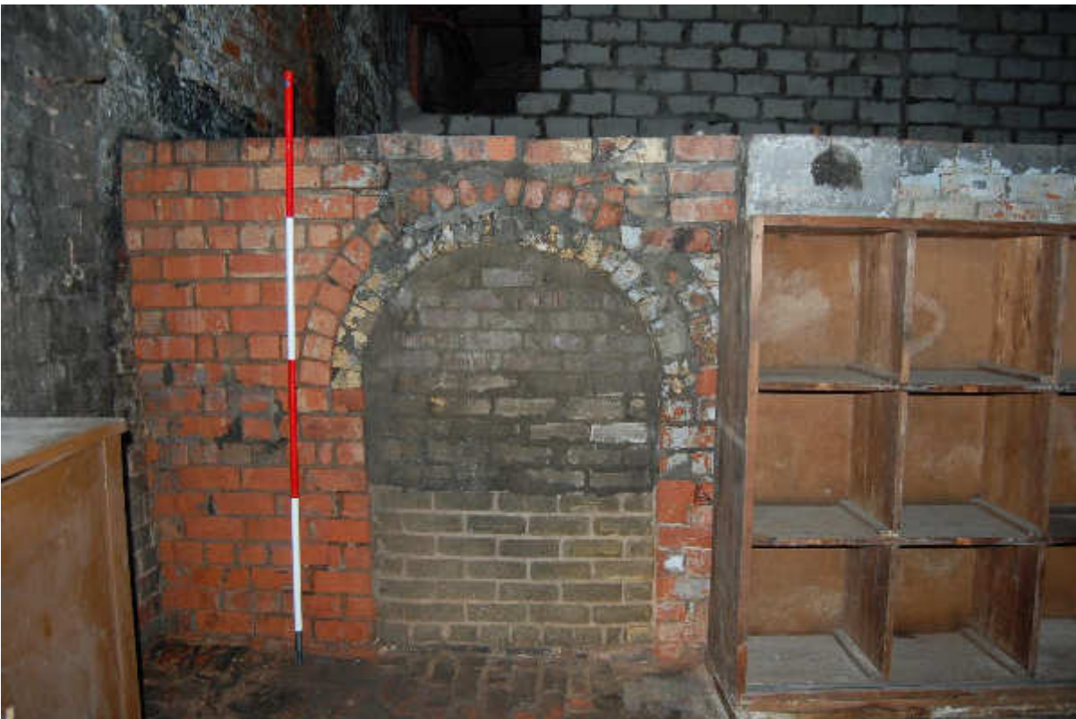
Illus 75 Building 52 wall 57 blocked door D52/11; facing E
