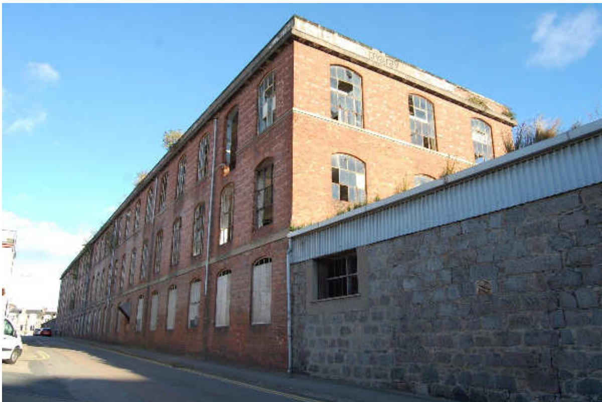
Illus 26 Ann Street façade, Building 19 (right), Building 20, 21, 22 (left); facing NNE
