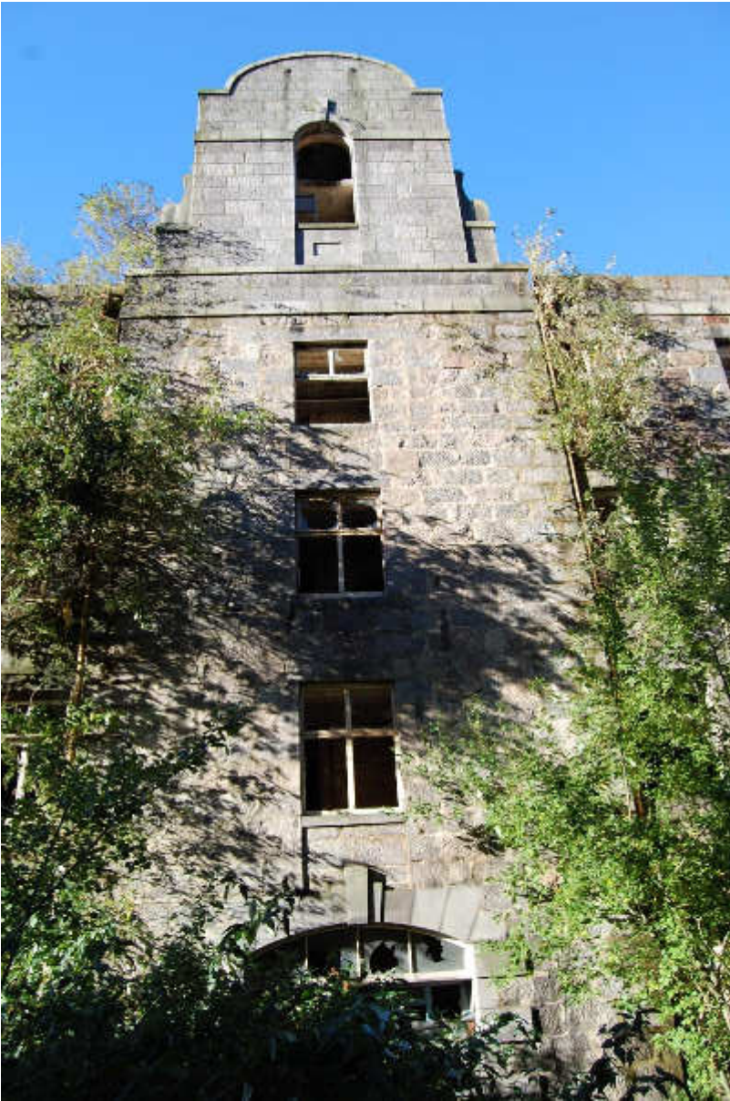
Illus 59 Building 48 stair tower; facing WSW
