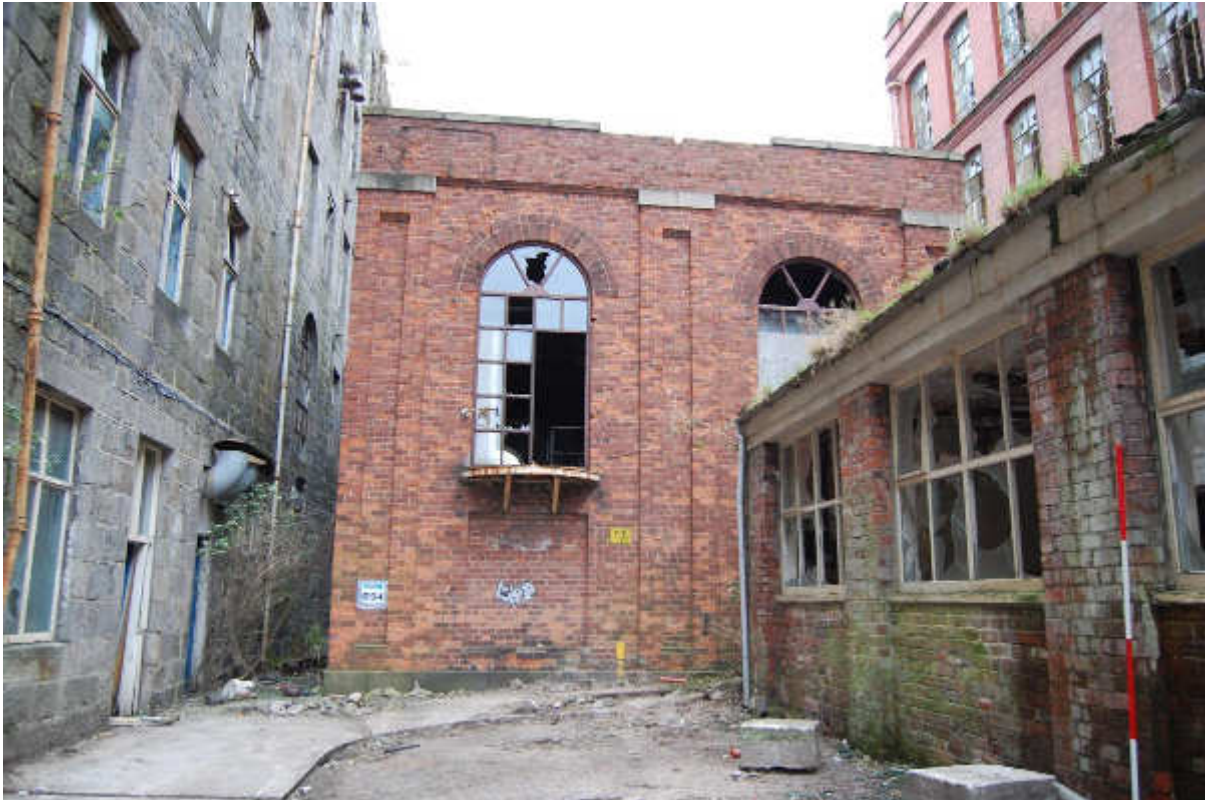
Illus 82 Building 54 S wall with Building 49/50 (left) Building 55 (right); facing NNW
