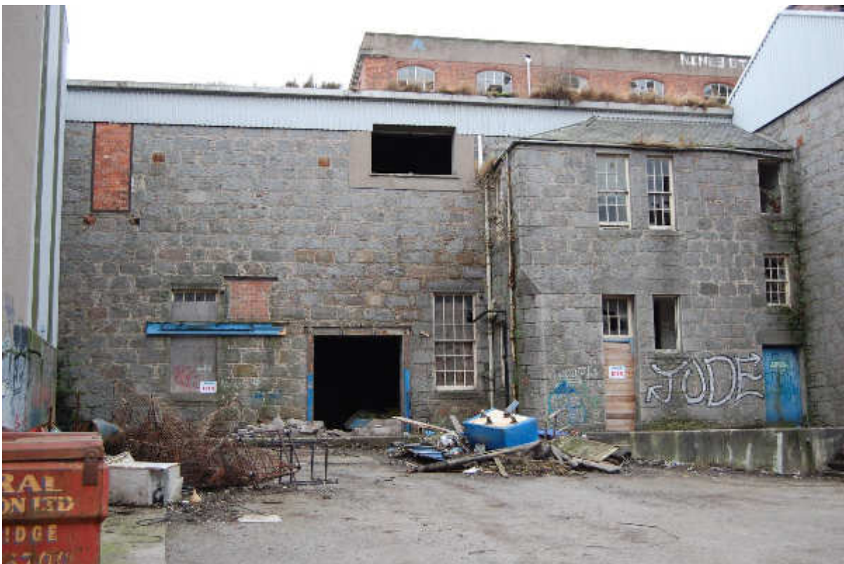
Illus 21 Building 19 (left) and 18 (right); facing WSW
