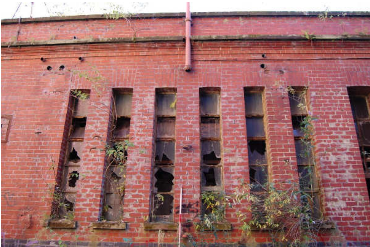
Illus 116 Building 90 W façade windows W90/11-/6 (L-R); facing ENE
