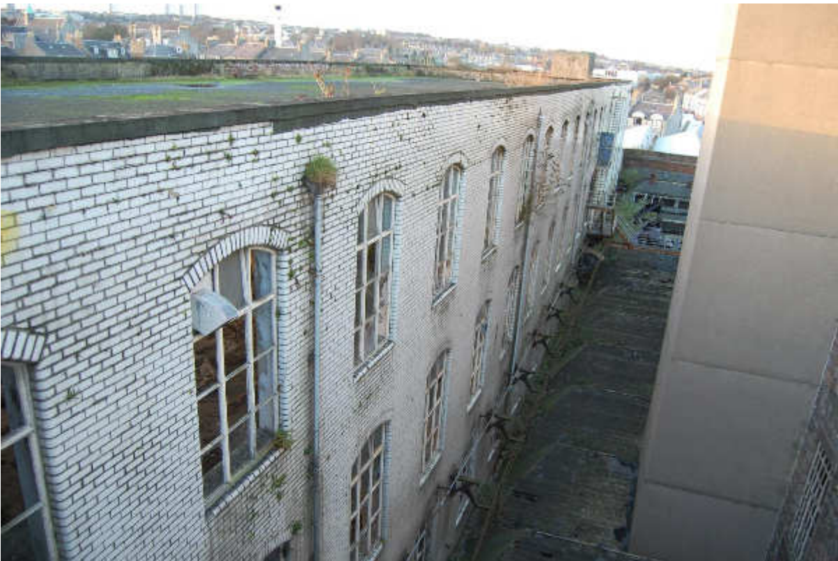
Illus 28 Building 21 N façade clad with white bricks; facing NNW
