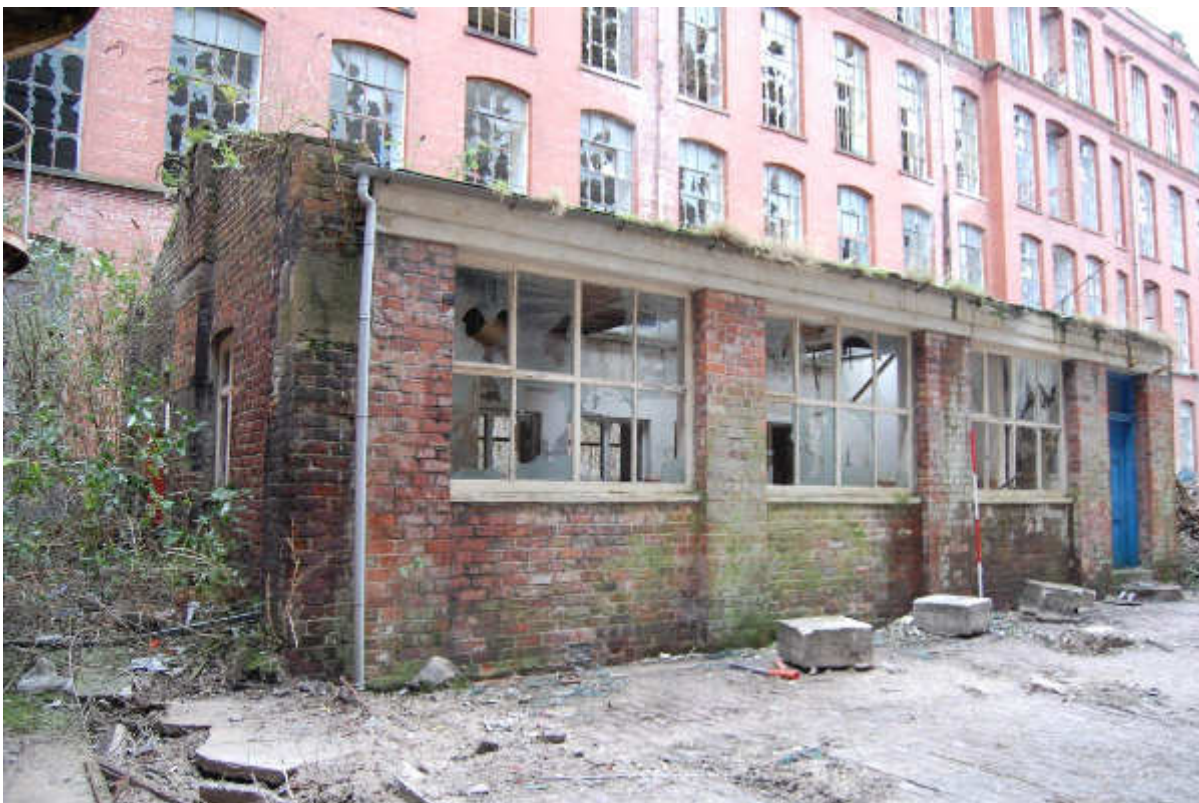
Illus 86 Building 55, W front façade, facing SE
