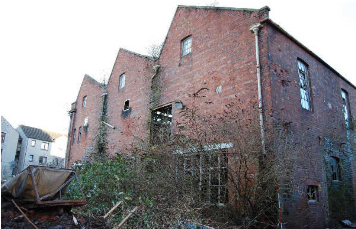
Illus 95 Building 83 W gable; facing NE
