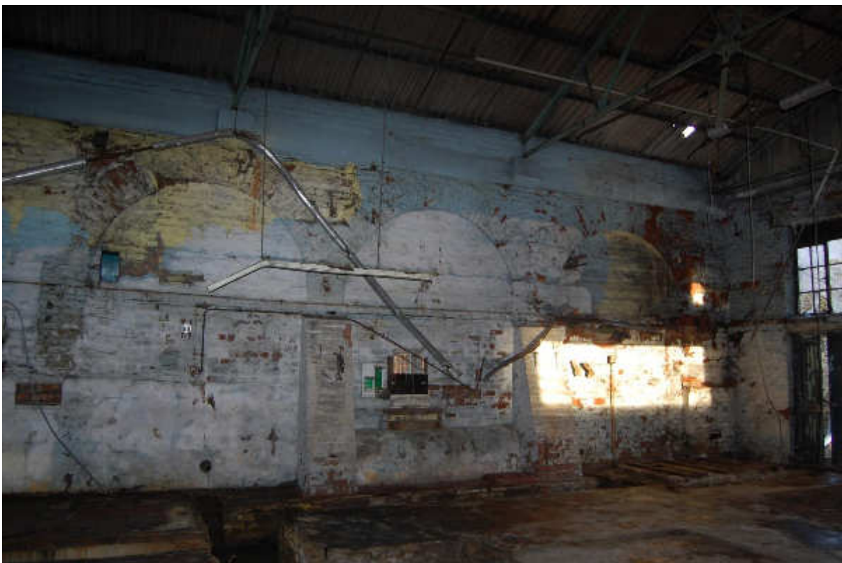
Illus 73 Building 52 interior N wall D52/7, 8, 9 (L-R); facing N
