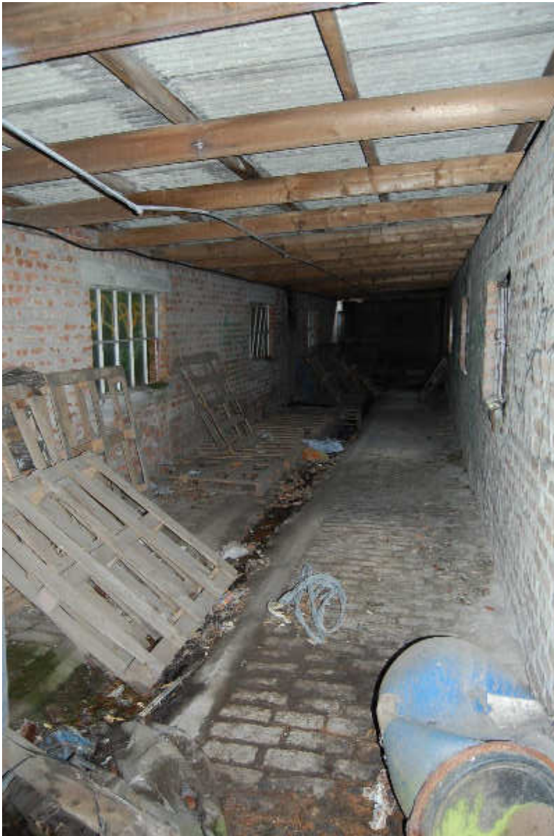
Illus 135 Building 102 hose pipe testing facility showing concrete gully (F39) with cobbled path either side (F38); facing SSE
