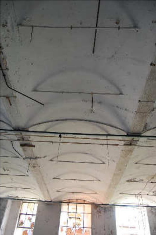
Illus 106 Building 86 cast iron and concrete ceiling, ground floor; facing ENE
