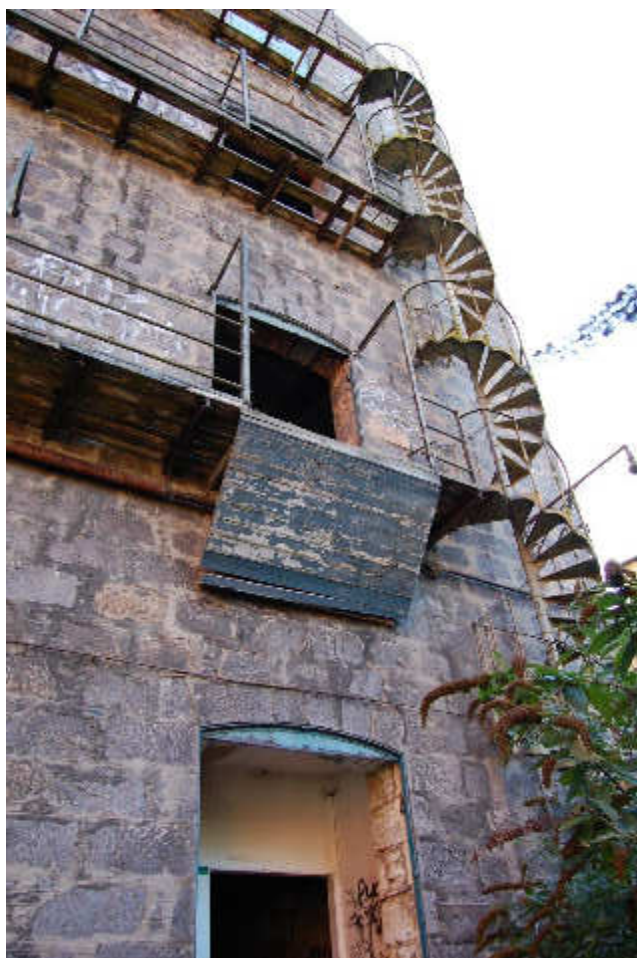
Illus 91 Building 68 W façade with cast iron spiral staircase; facing ESE
