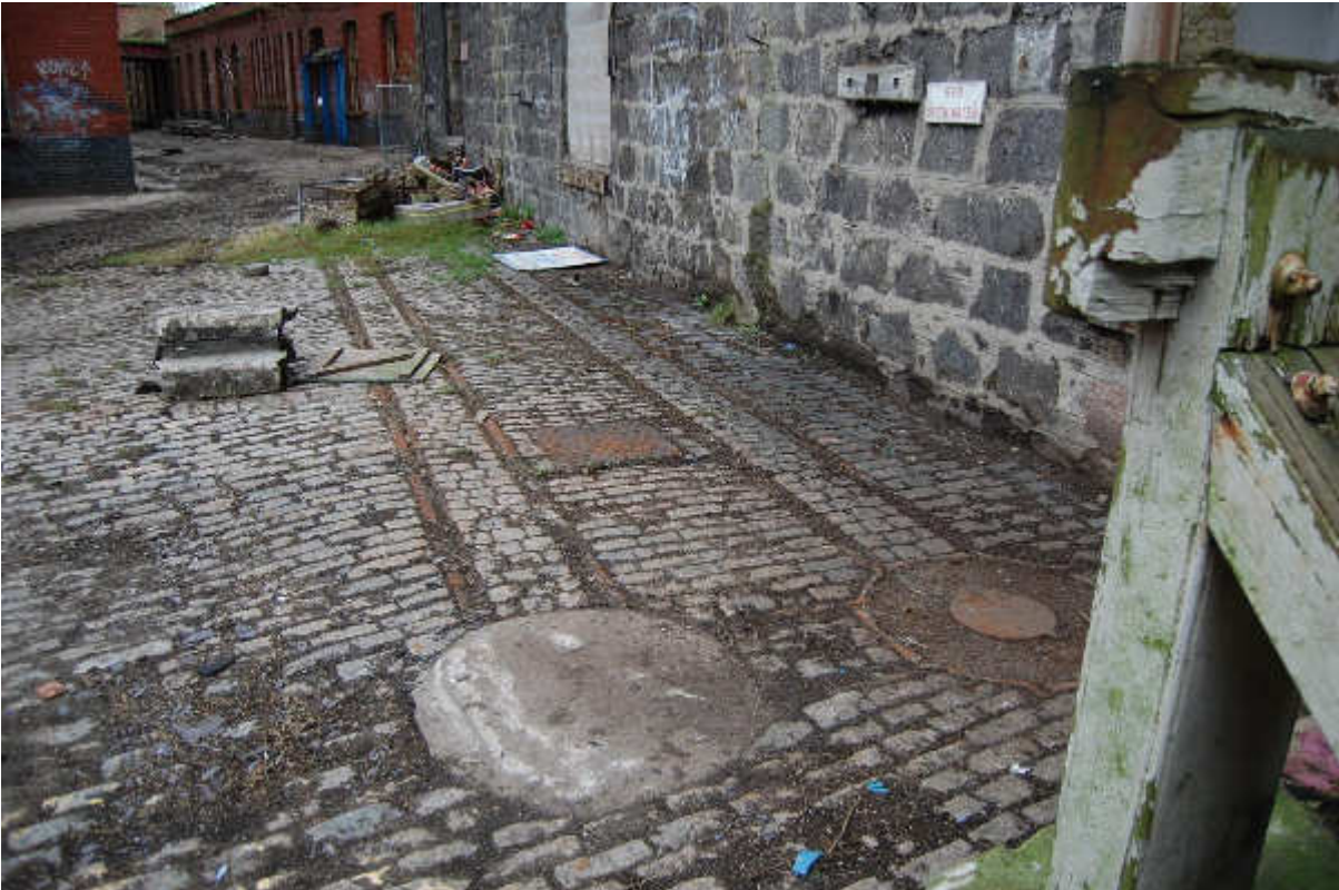
Illus 92 Cart tracks F14 on W side of Building 68 with wooden stop barriers (F50, right); facing N
