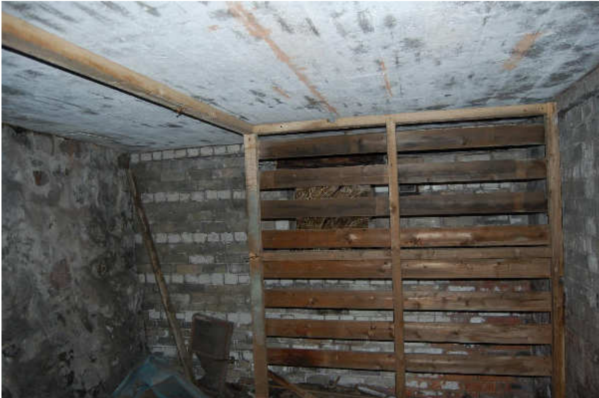
Illus 137 Building 103 interior showing stone boundary wall (left) and shuttered concrete roof; facing SSE
