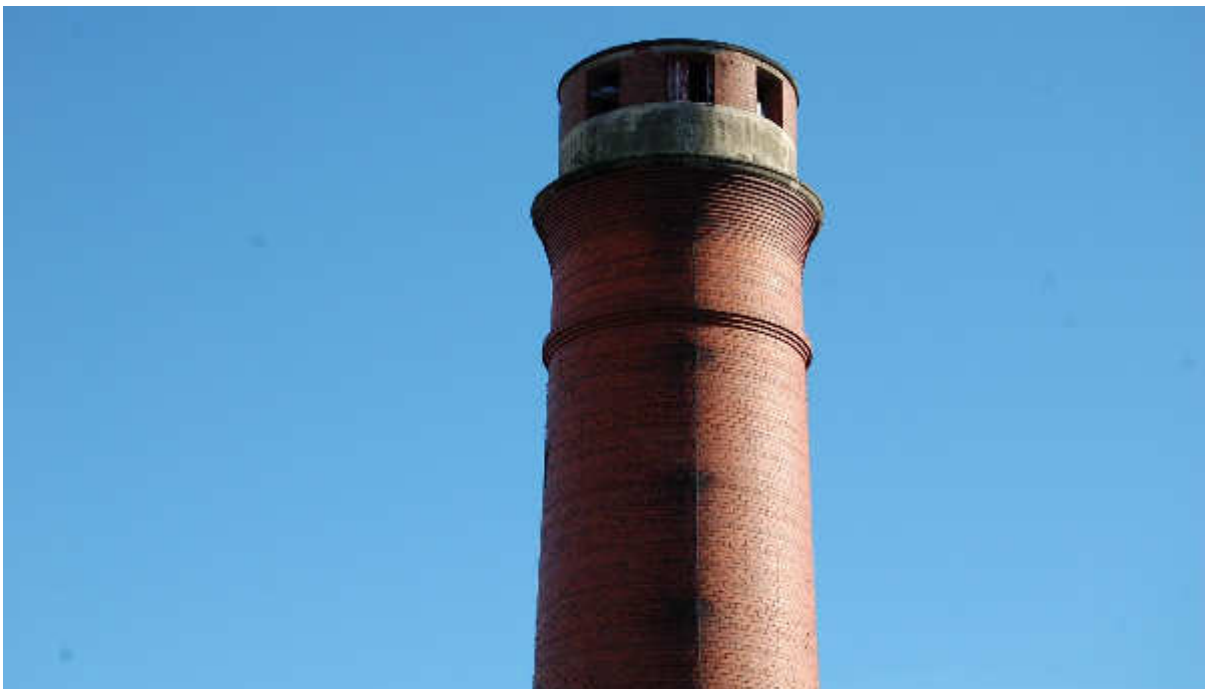
Illus 120 Top of round sectioned brick chimney 88A from Building 86 second floor
