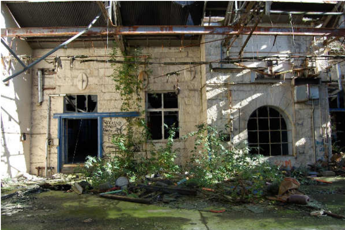
Illus 68 Building 50 SW façade with Building 47 attached (top); facing ENE
