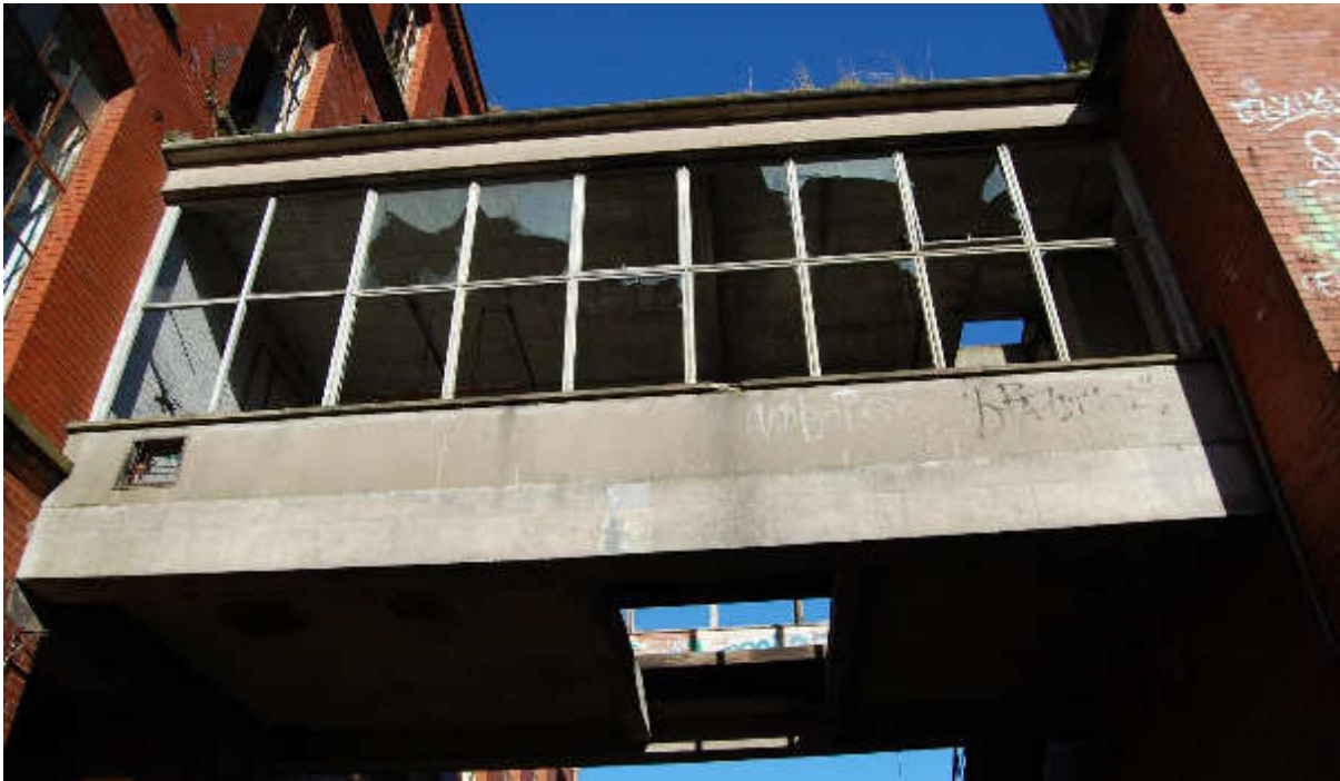
Illus 133 Building 86 (left) gantry 100, building 99 (right); facing NNE
