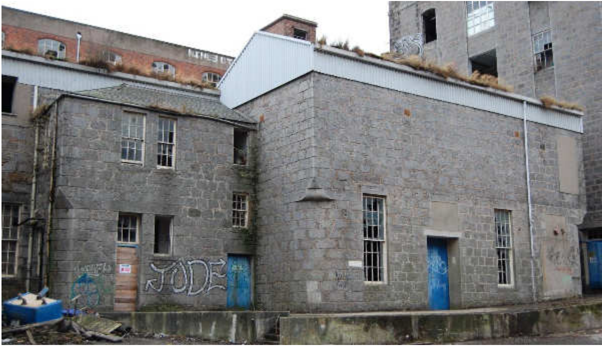
Illus 20 Building 18 E façade; facing WNW
