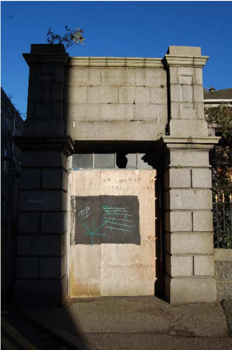
Illus 150 F46 granite pedestrian gate through Building 1 into complex; Facing NNW
