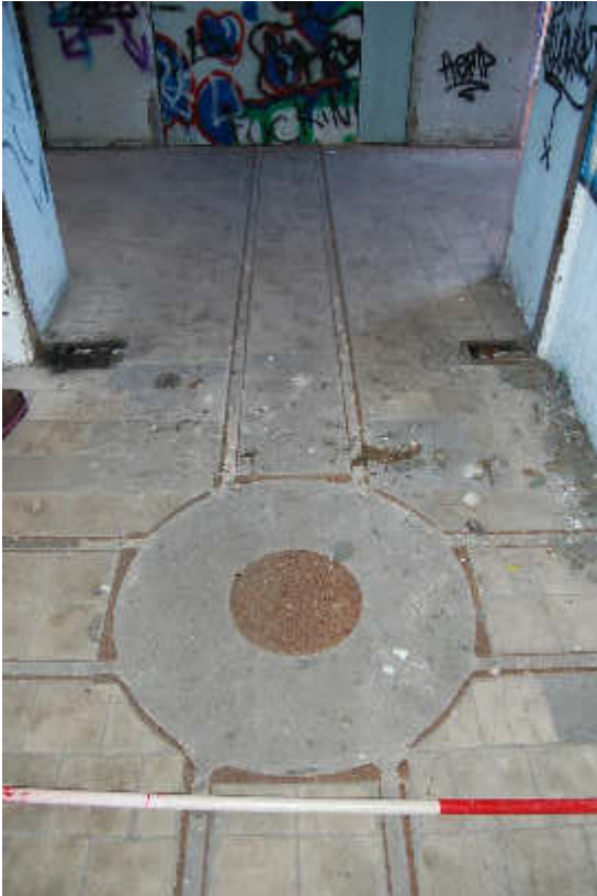
Illus 107 Building 84 first floor cart tracks leading to lift; facing SSE
