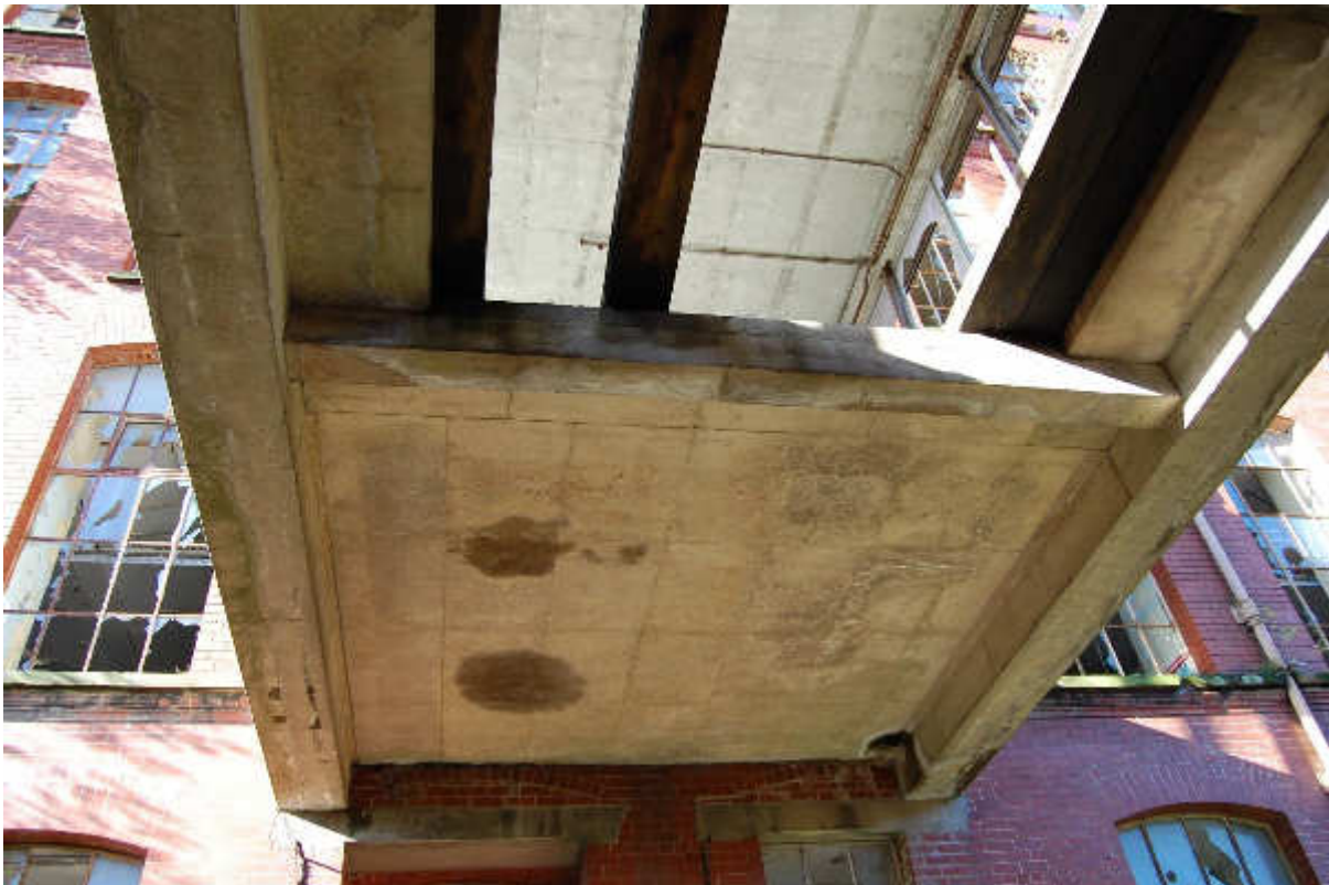
Illus 134 Underside of gantry Building 100 showing concrete block construction; facing ENE
