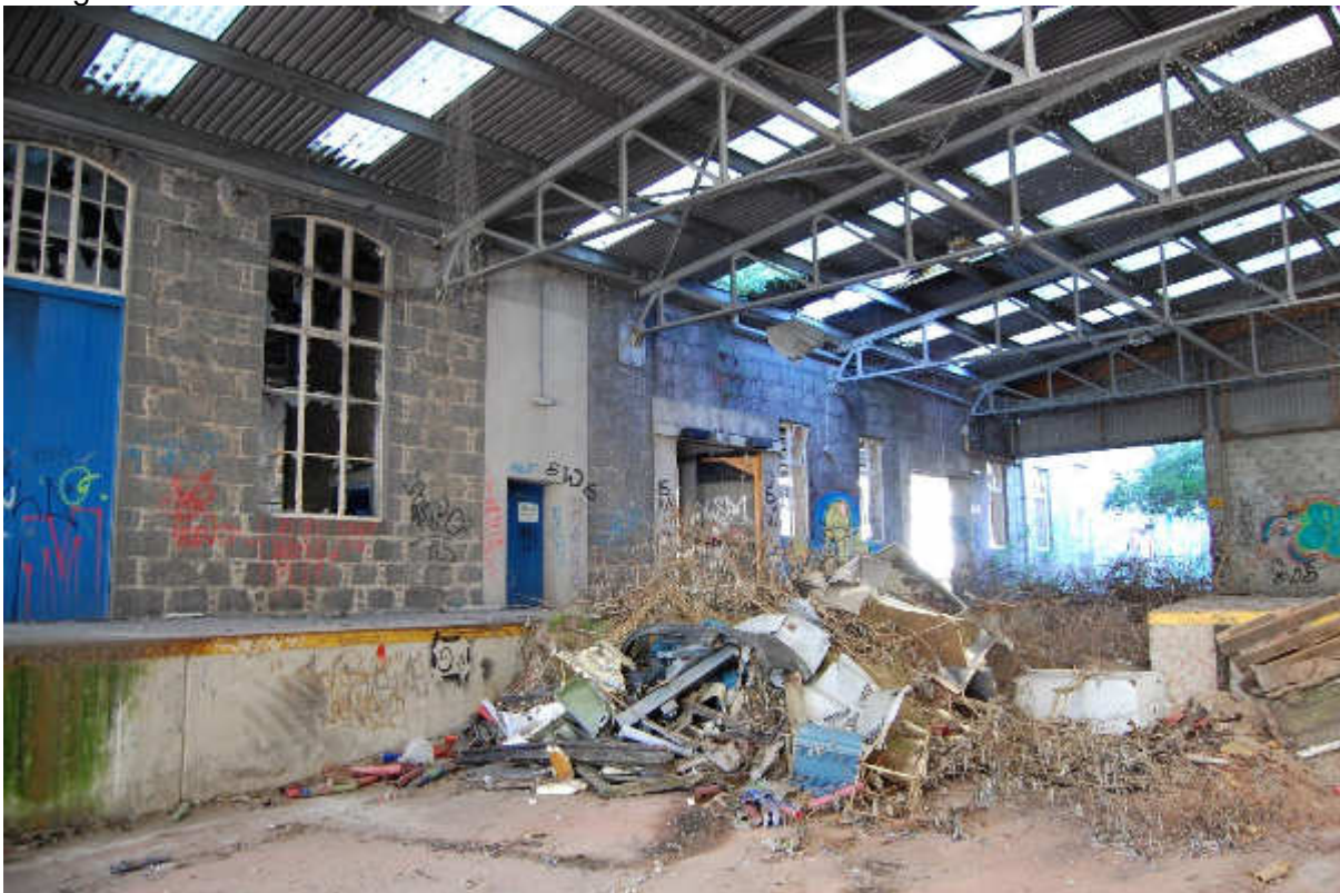
Illus 48 Building 32, 30 built into loading bay Building 29; facing NW
