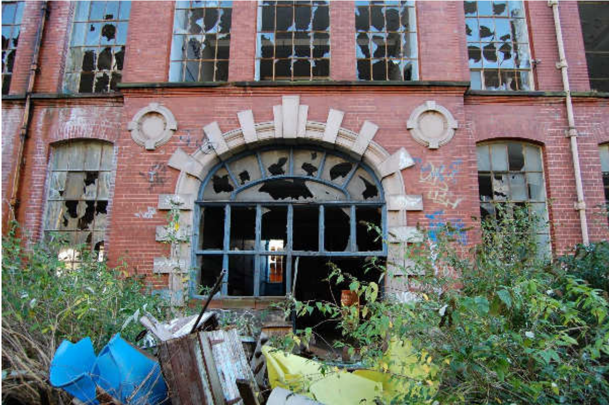
Illus 104 Building 85 Door D84/8 showing dressed granite mouldings and roundels above; facing ENE
