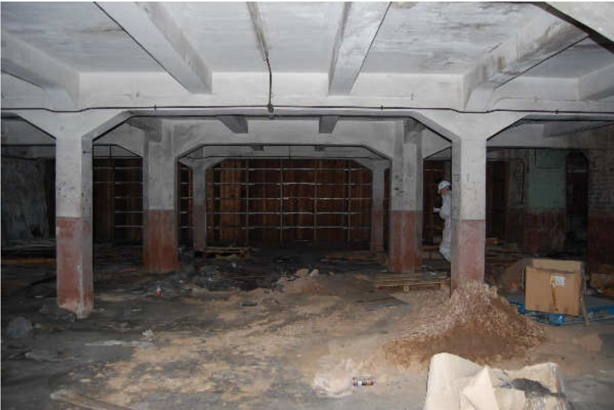
Illus 30 Building 21 basement showing octagonal concrete pillars and roof structure
