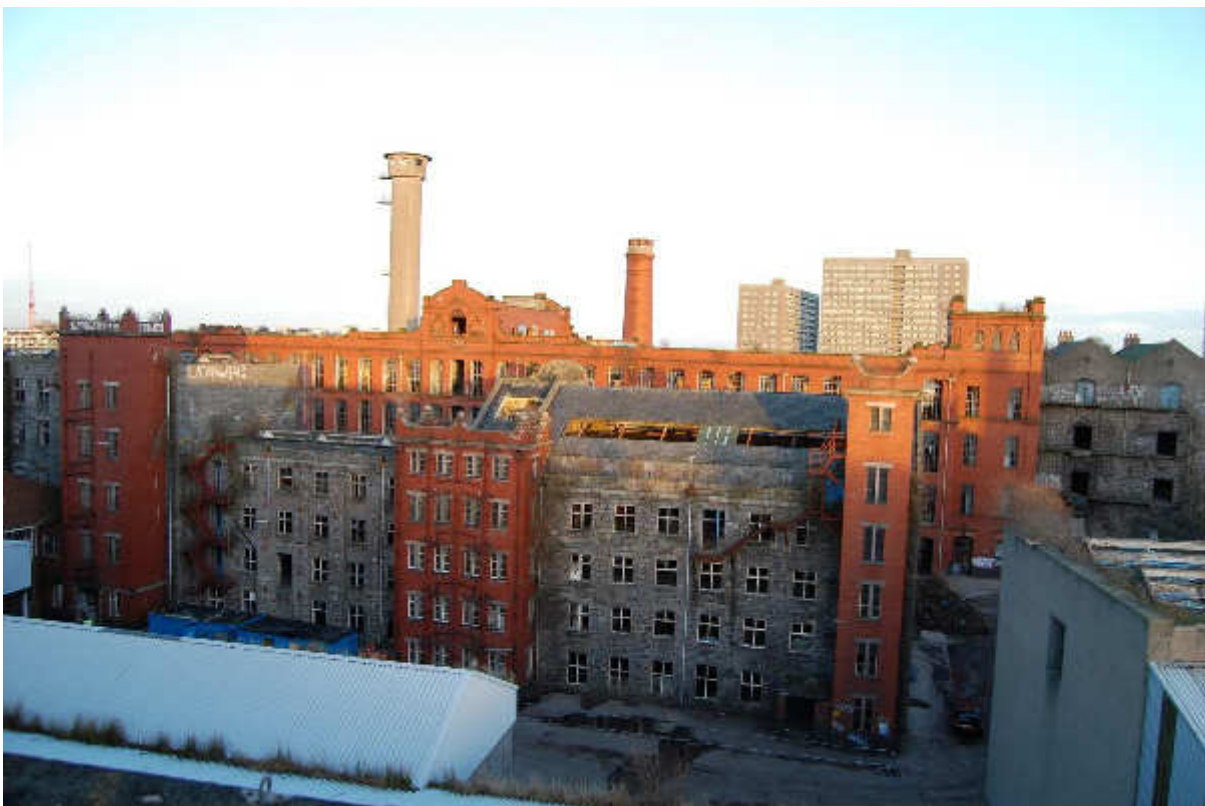
Illus 56 Buildings 43, 44, 45, 48 from roof Building 21; facing ENE
