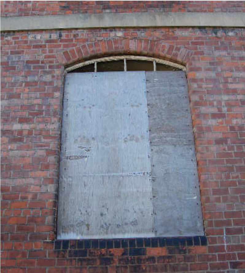
Illus 27 Building 20 W Ann Street façade window W20/1 showing arched window with grey brick sill and red brick arched lintel; facing ENE
