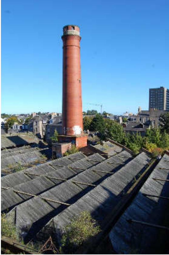
Illus 119 Chimney 88A from 3 rd floor Building 84 showing roofs of Buildings 88-90; facing NE
