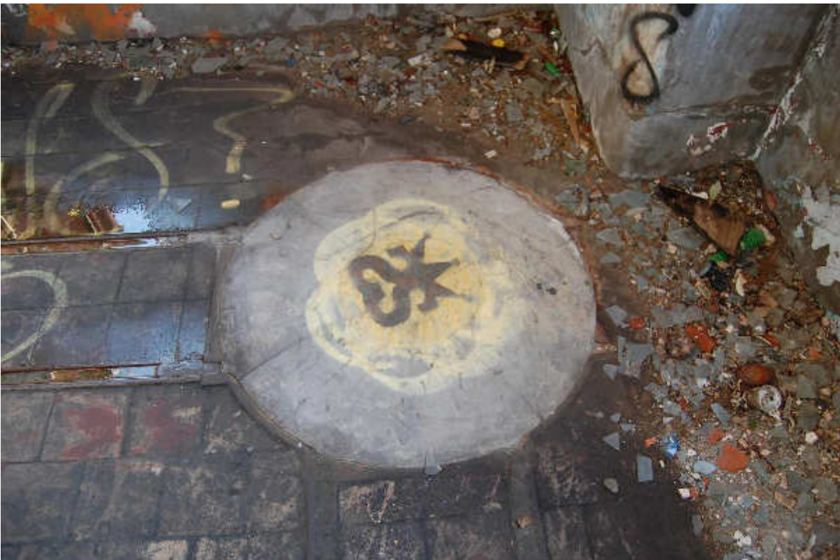
Illus 109 F31 terminal on corner of 3 rd floor Building 84; facing ENE
