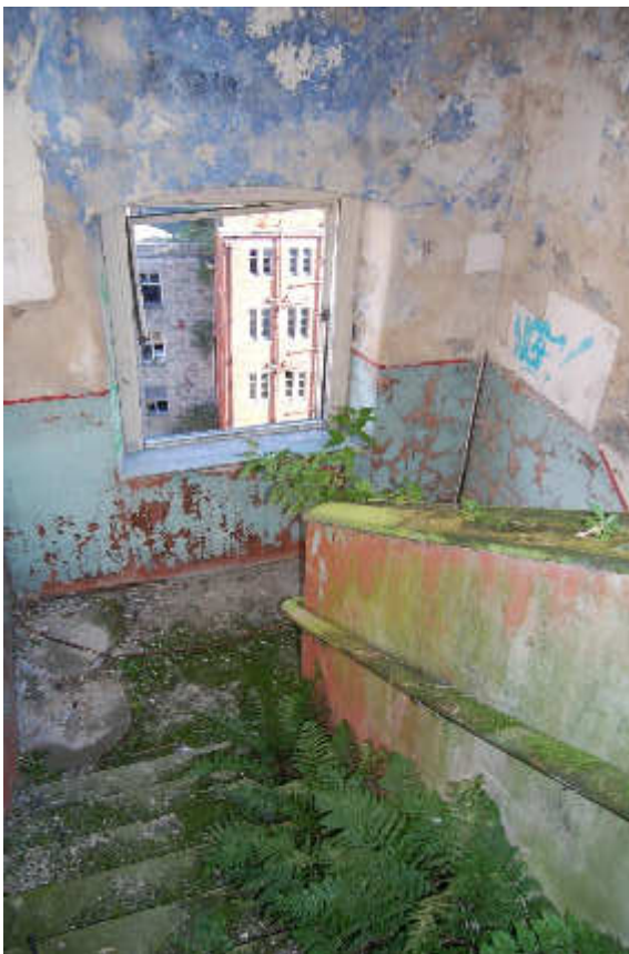
Illus 52 Building 32 SE staircase with window W32/20; facing E
