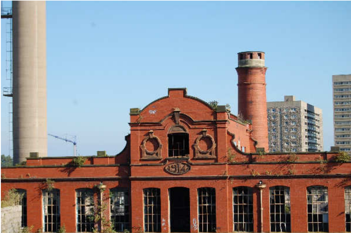
Illus 102 Building 85 date plaque '1914'; facing ENE
