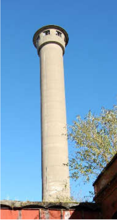
Illus 128 Concrete chimney Building 98 with gantry 100 below; facing SSE
