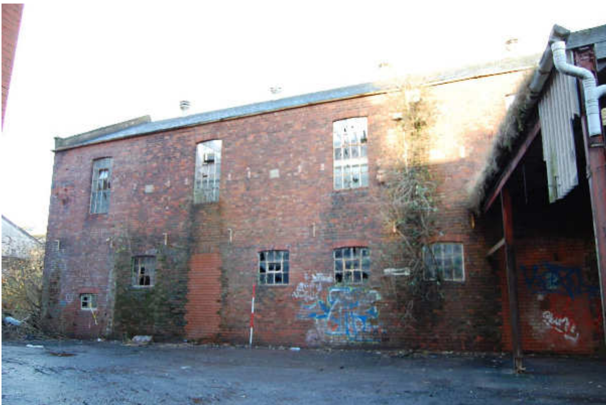
Illus 96 Building 83 S wall; facing NNW
