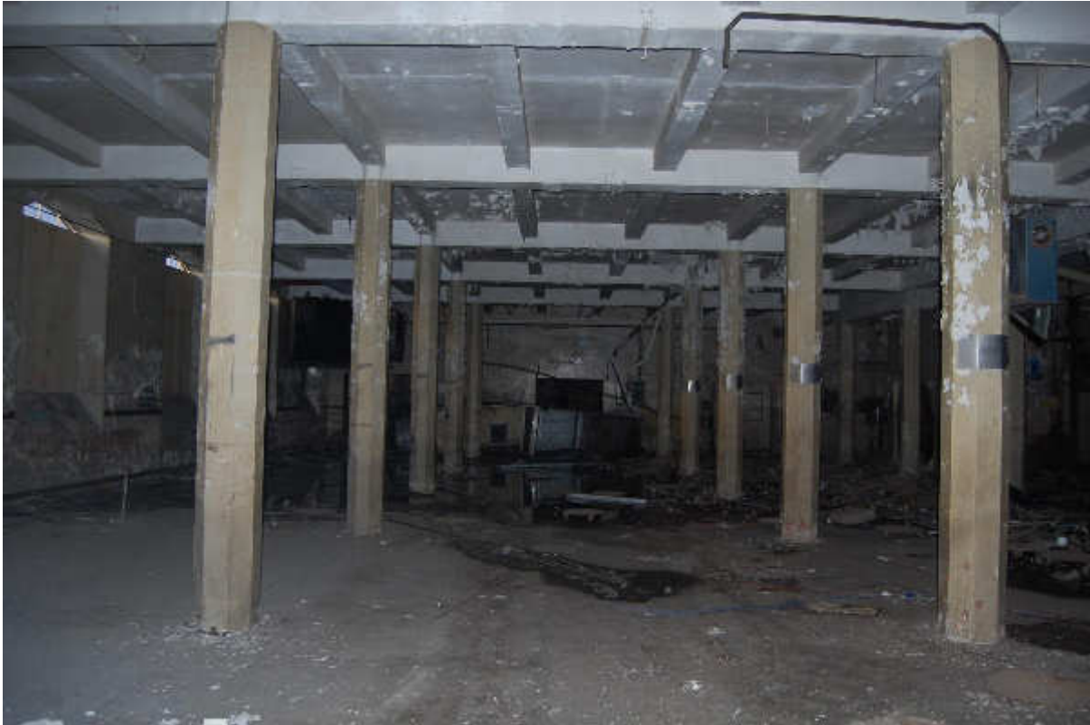
Illus 31 Building 20 1 st floor; facing NNW
