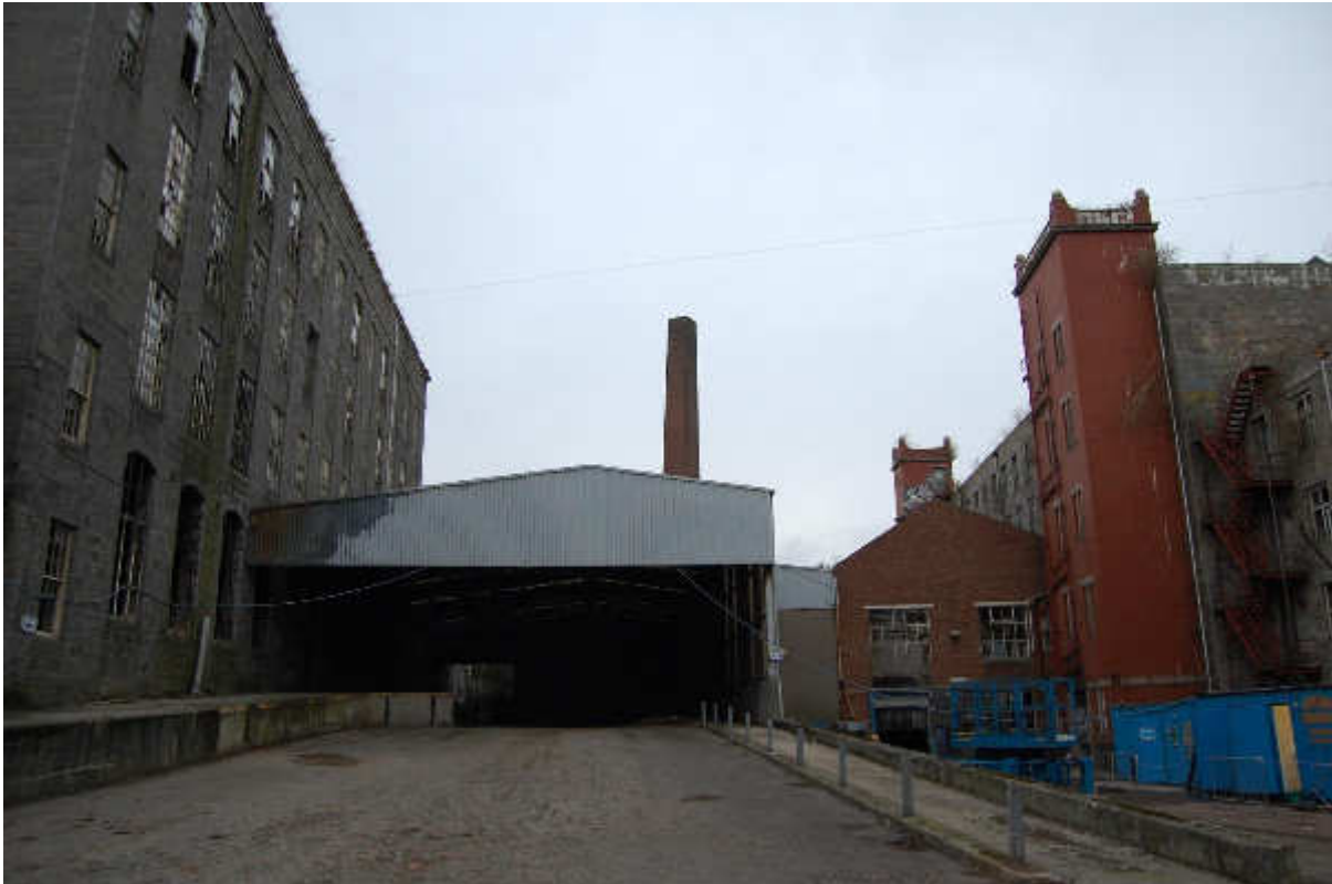
Illus 41 Loading bay Building 29 (centre) with Building 32 (left) Building 47 (centre right), Building 49 (right); facing NNW
