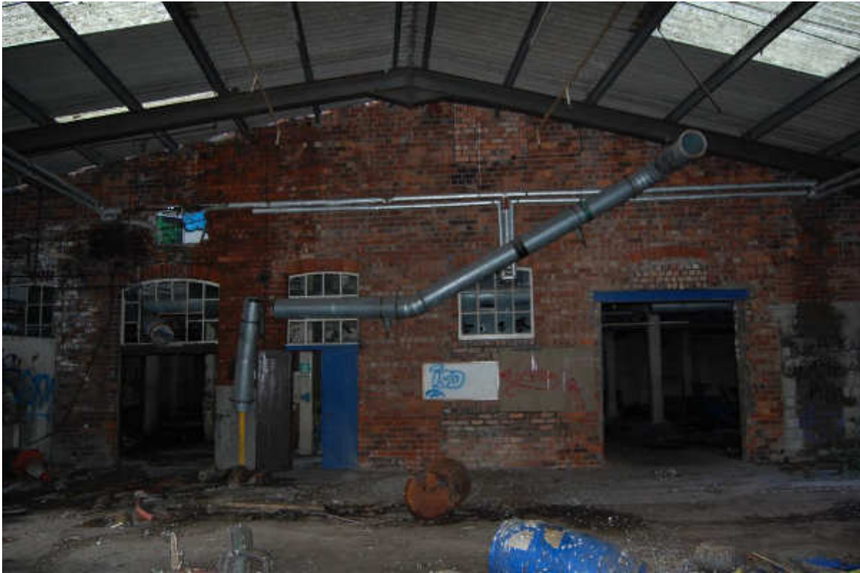
Illus 99 Building 83 S wall built into later Building 101; facing NNW
