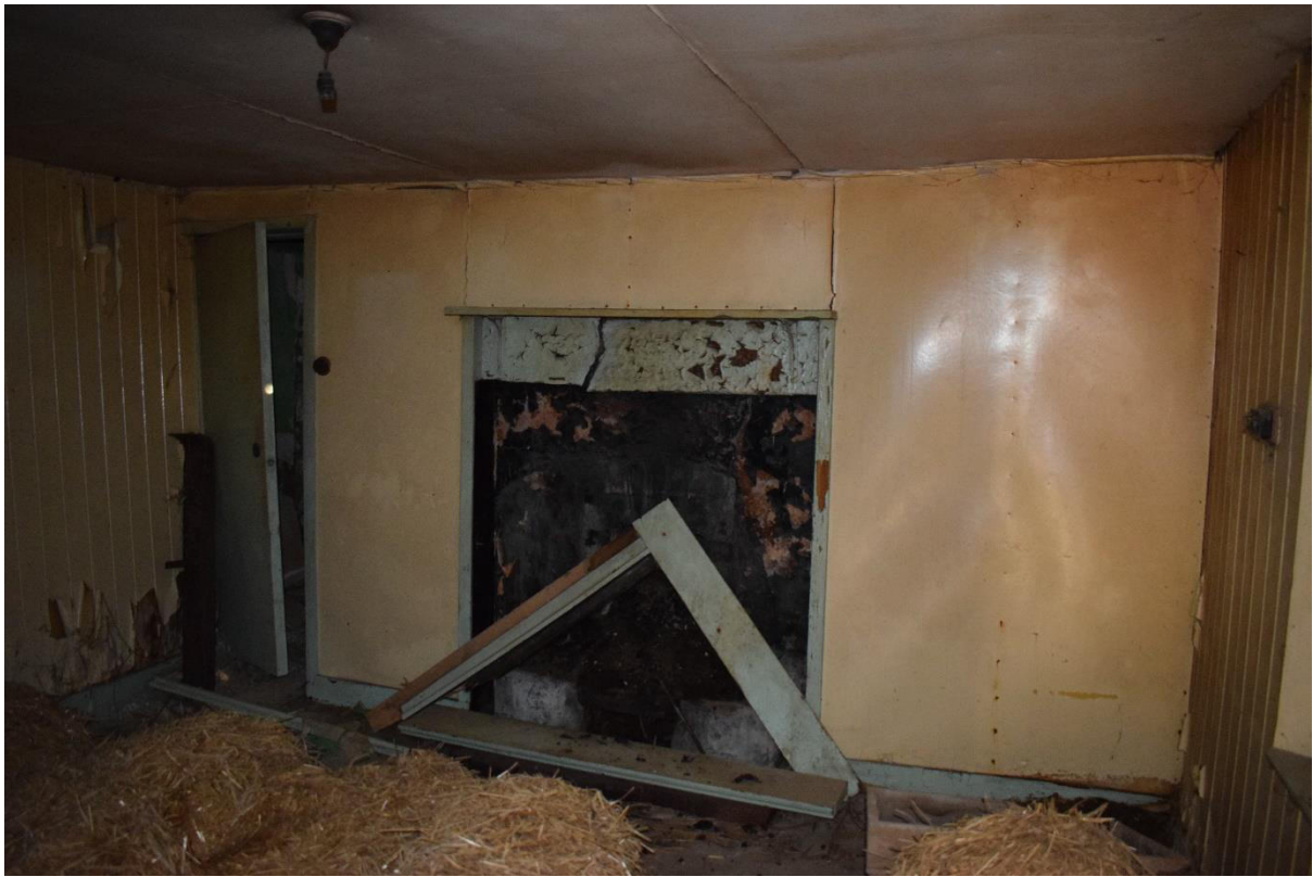
Illus 7 Room 2 interior NE wall with fireplace F9; facing NE
