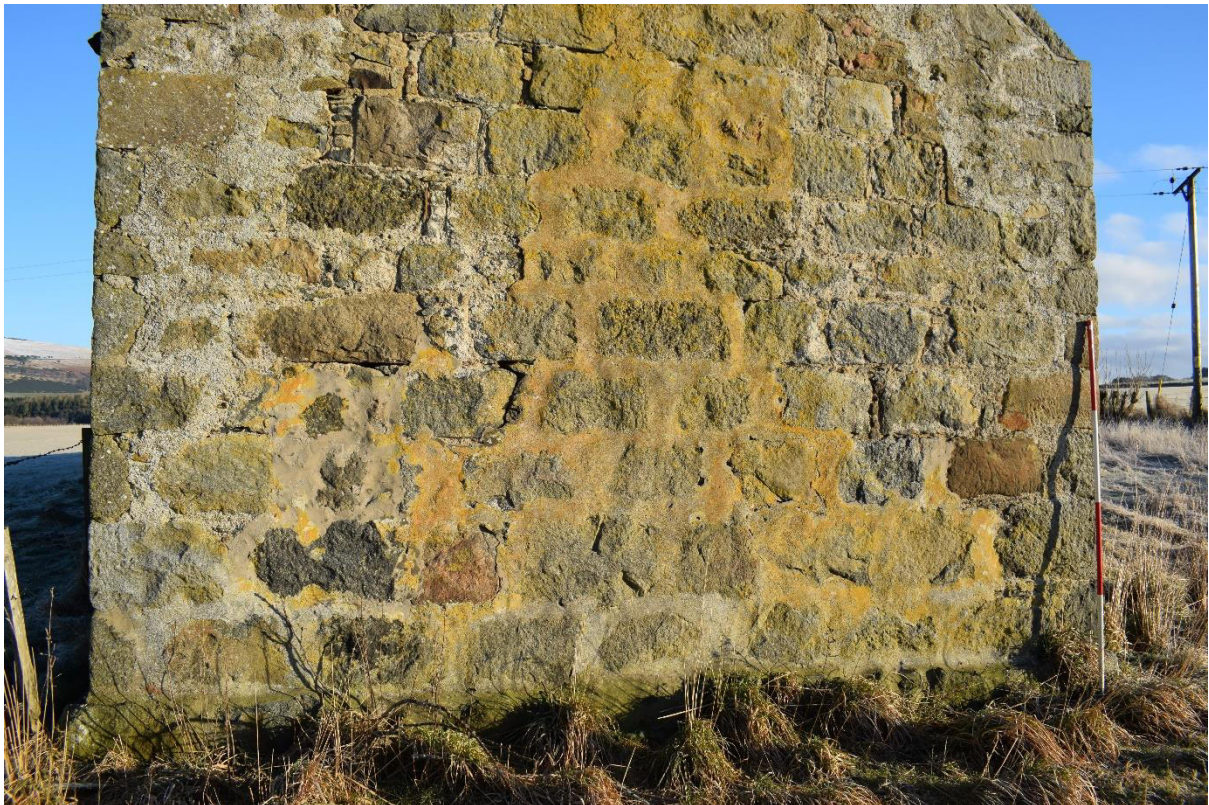
Illus 4 SW gable with blocked window W3 (left); facing NE
