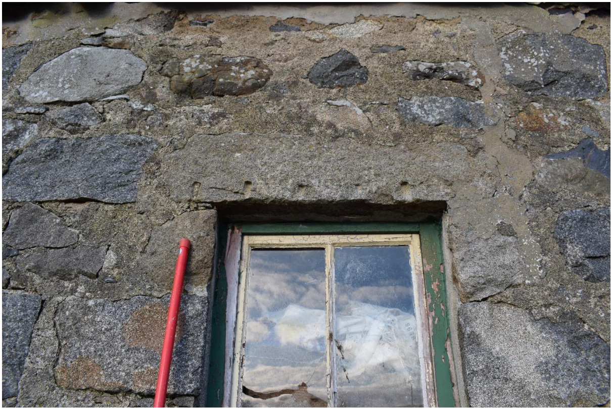
Illus 3 W1 lintel with drilled granite block lintel; facing NW
