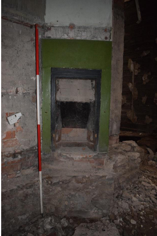
Illus 20 Room 5 corner fireplace F9; facing SE
