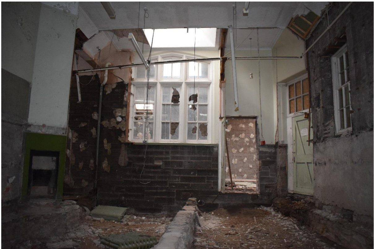
Illus 13 Room 5 south wall which was originally an outside wall with W36 (centre) with fireplace F9 (left) and D5 (right)
