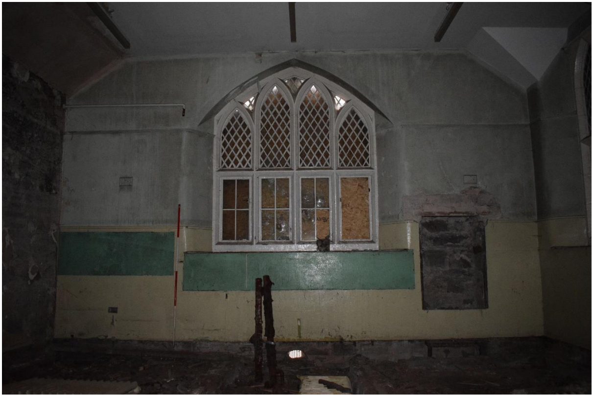
Illus 16 Room 9 E wall Phase 2 window W12; facing E
