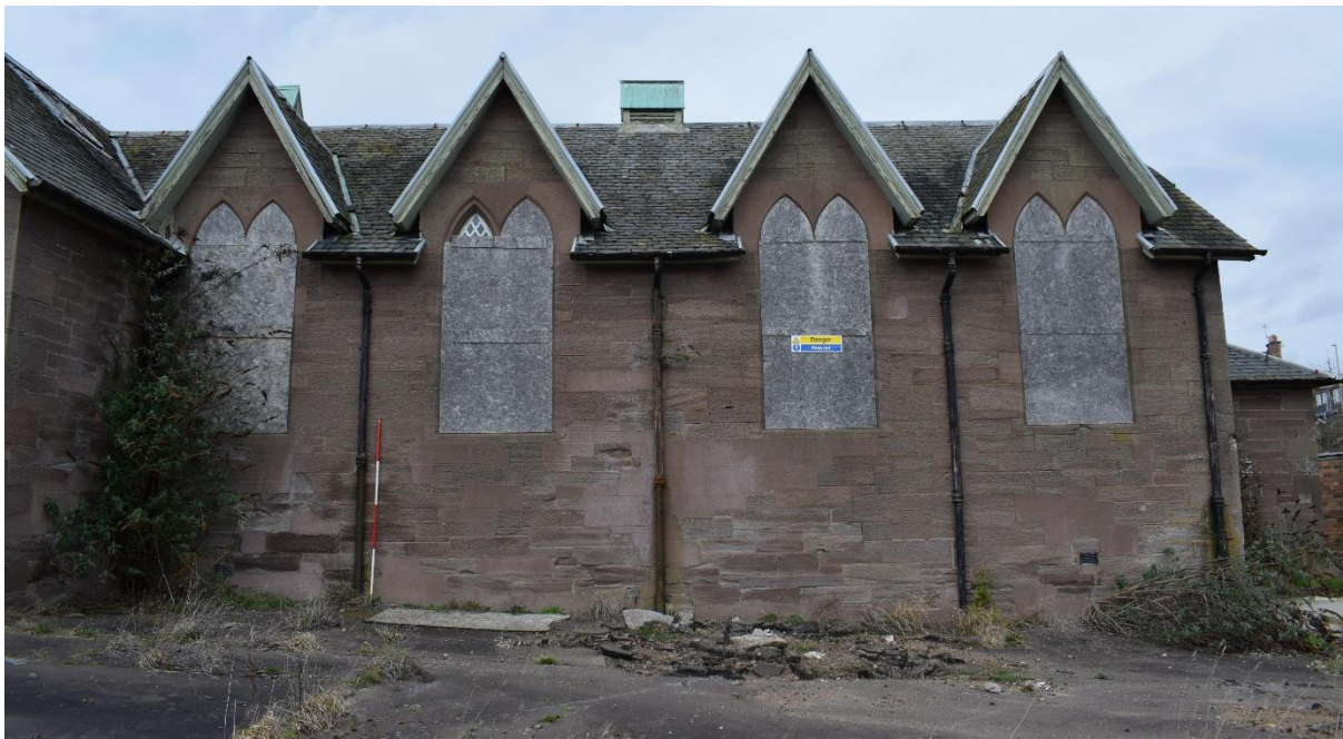
Illus 9 Phase 2 S façade W8, W9, W10, W11 (l-r); facing N
