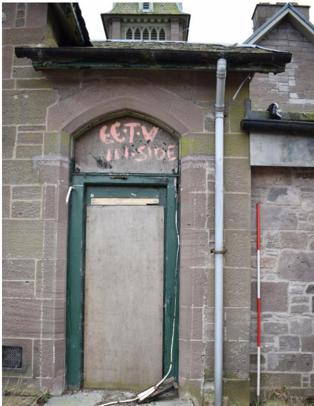
Illus 10 Sandstone doorway into Phase 2 school from N D4; facing S
