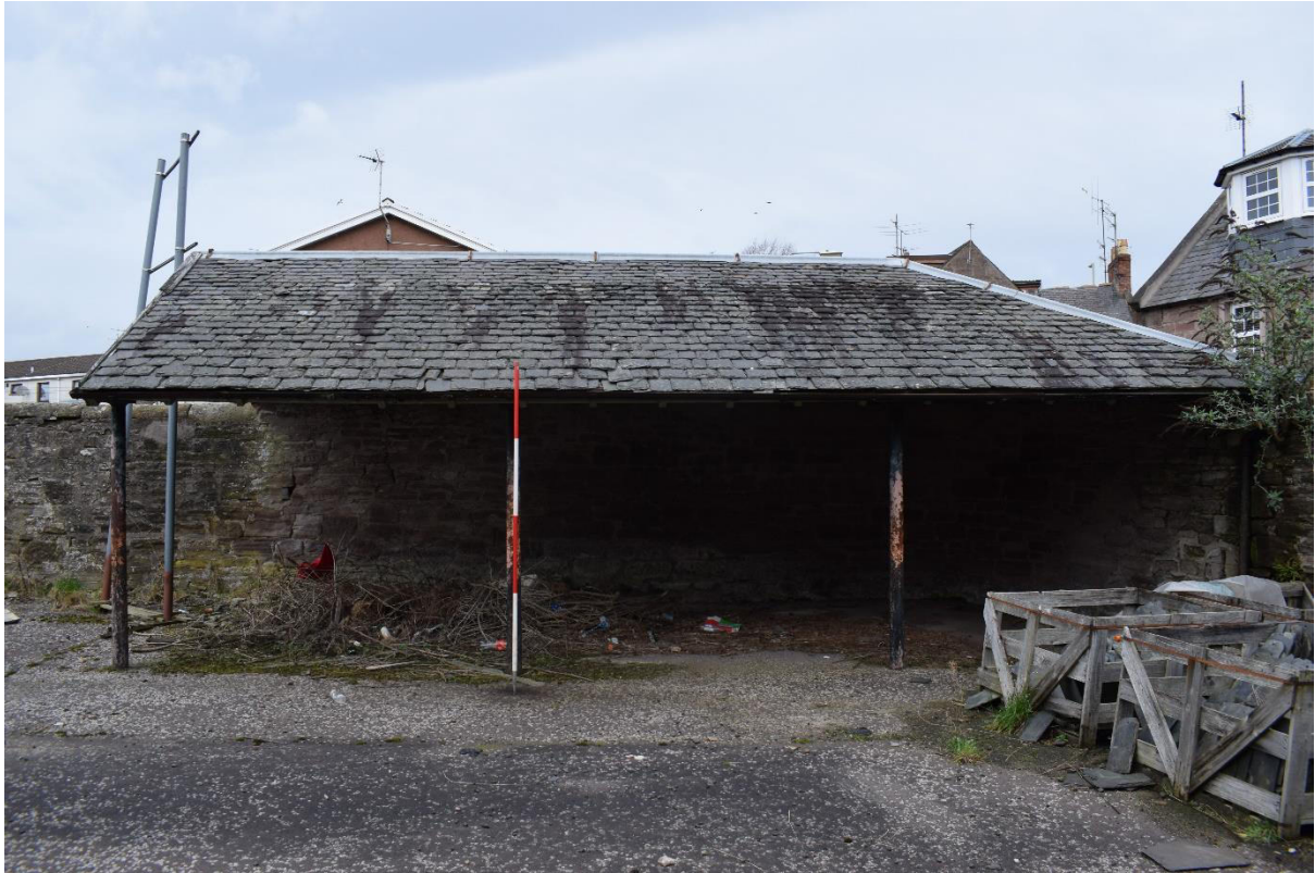
Illus 24 Cast iron pillar construction with slated wooden roof; facing N
