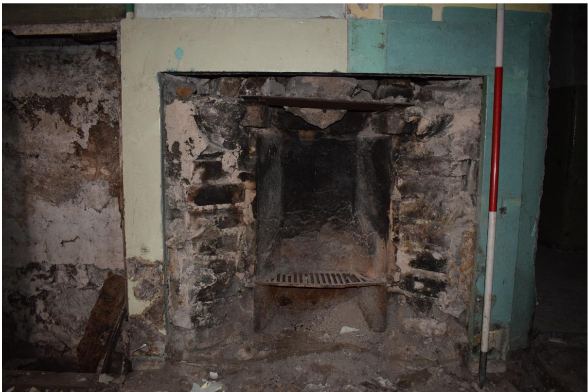
Illus 8 Room 3 N wall fireplace F7 with concrete surround; the tiles have been removed; facing N
