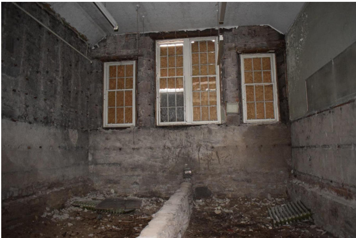
Illus 19 Room 5 N wall windows W18, W17, W16 (l-r) showing sleeper wall in centre for supporting wooden flooring and vent (above sleeper wall); facing N
