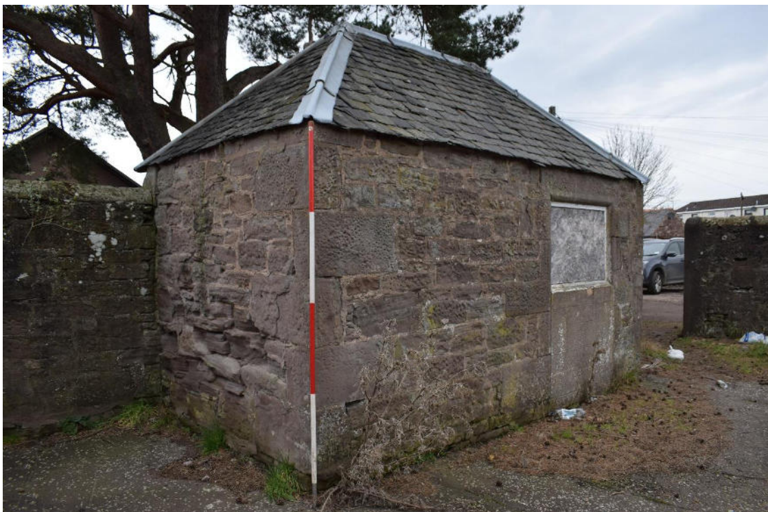
Illus 23 Building 3 showing D26 (blocked and reopened as window); facing NW
