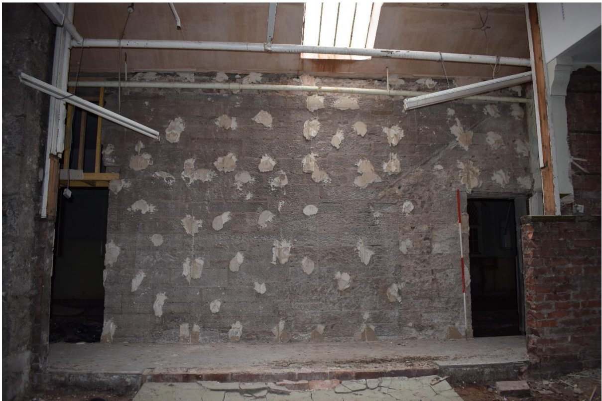
Illus 15 S wall Room 9 D20 (left) D19 (right) showing brick corridor inserted between rooms; facing S
