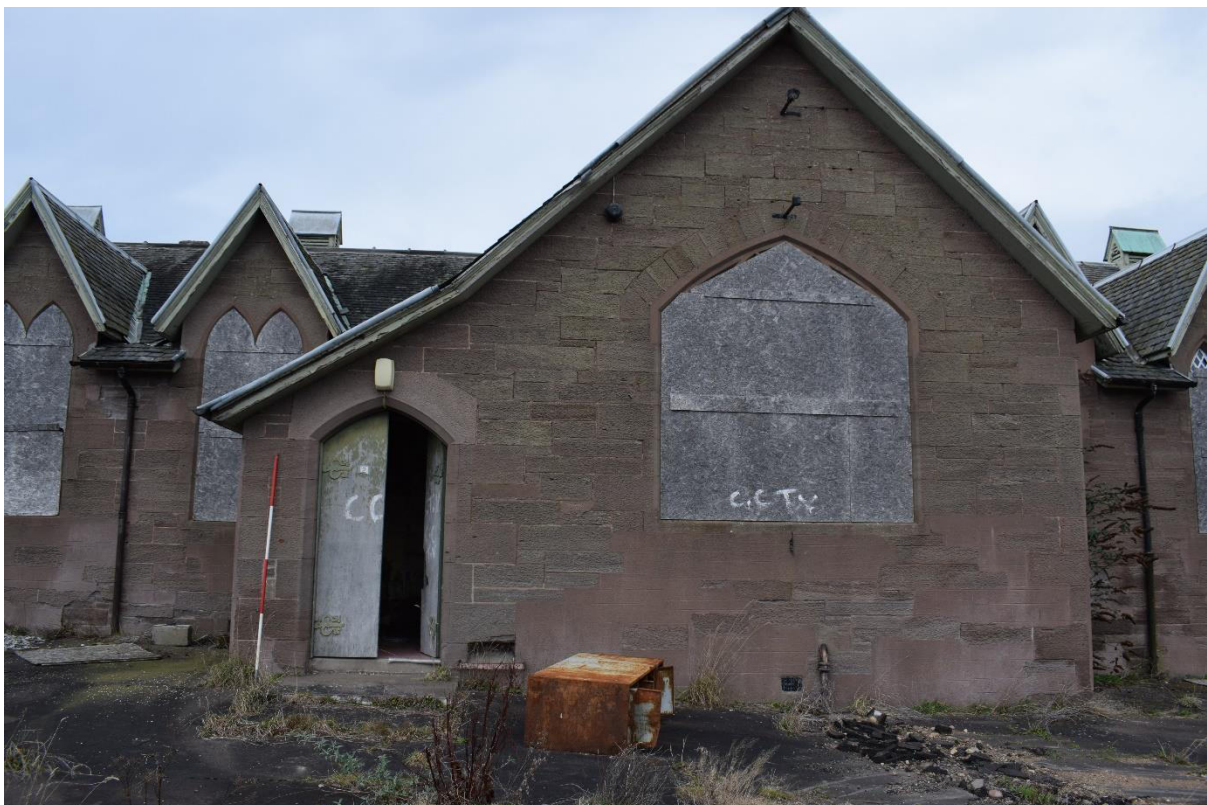
Illus 6 Phase 1 D1 and W7 on S façade; facing N
