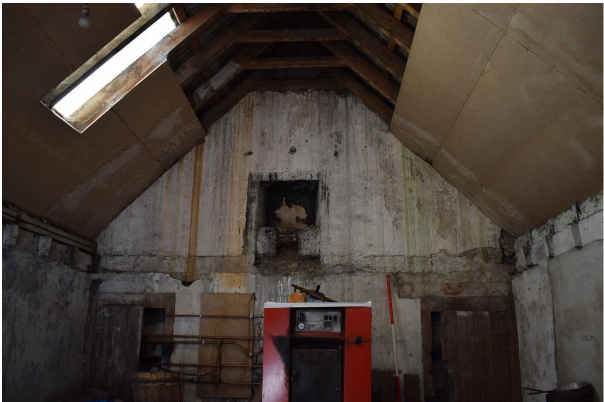
Illus 12 Building 1 Room 2 SW wall 1 st floor fireplace F22 (top) and wood alcoves F15 (left) F14 (right)
