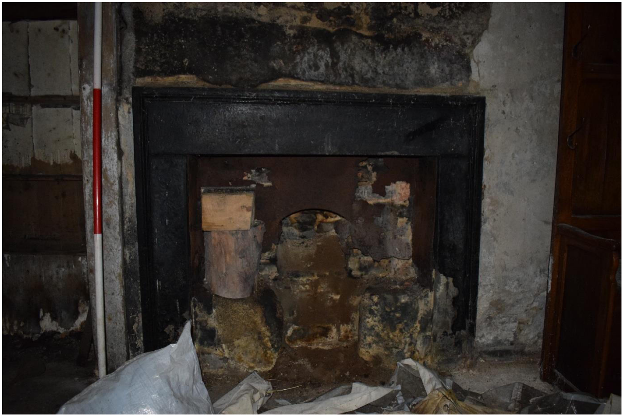
Illus 9 Room 1 fireplace on NNE wall F12; facing NNE
