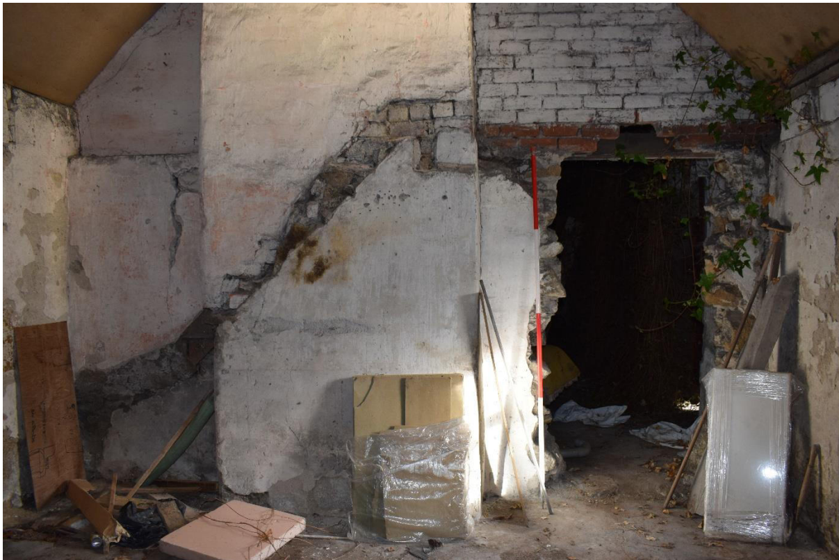
Illus 13 Room 2 NE wall with chimney breast F10 and scar where stair was removed; facing NE
