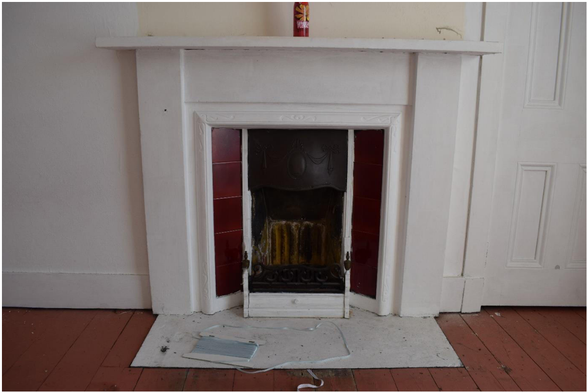
Illus 20 First floor Room 12 fireplace F19 ; facing ESE
