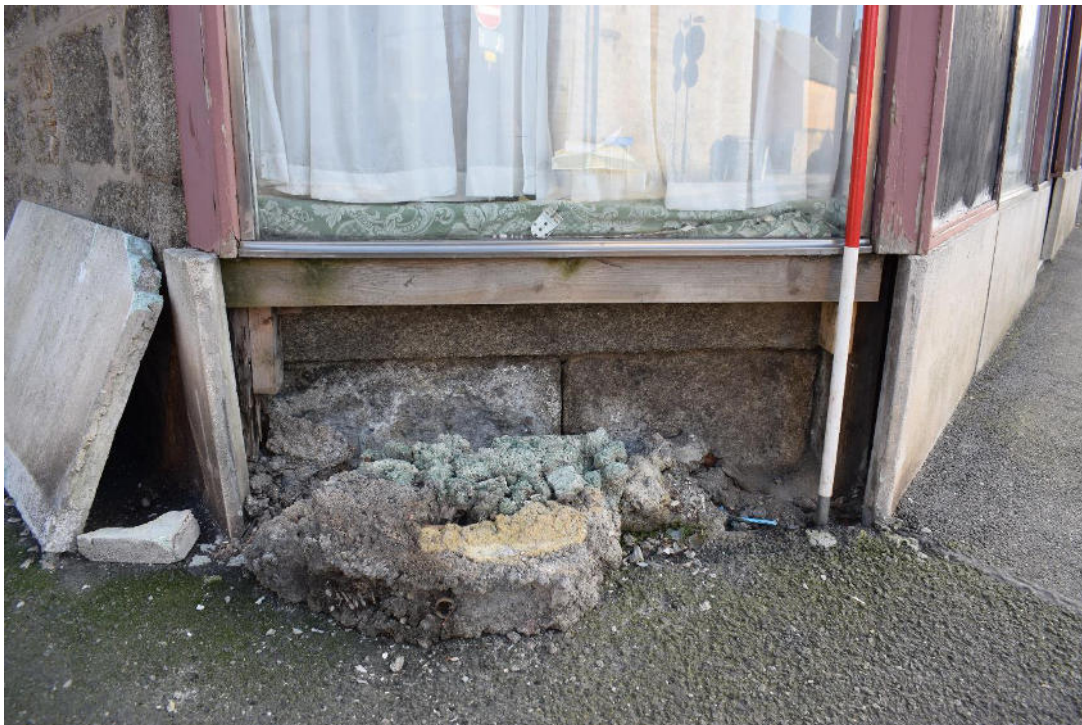
Illus 23 Building 2 W corner at junction of streets showing concrete shop frontage removed and granite building behind; facing E
