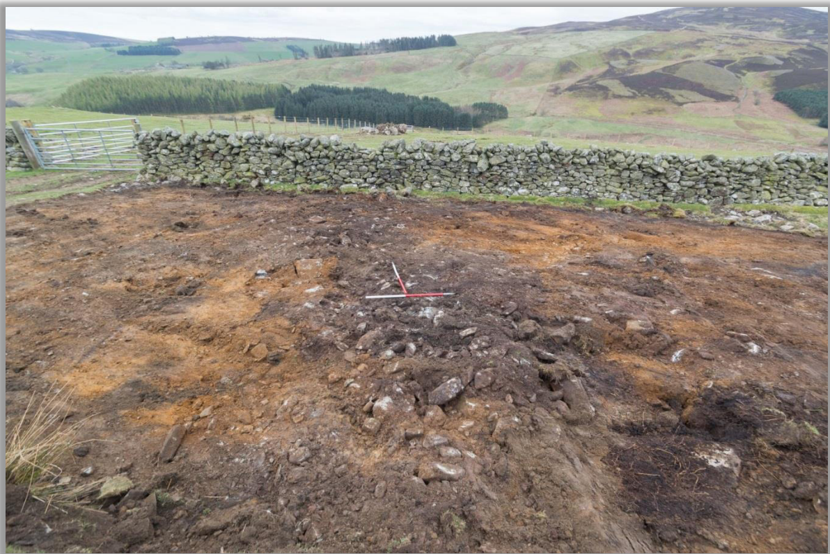
Illus 5: Natural stone-filled gully encountered during the early phases of the soil strip.
