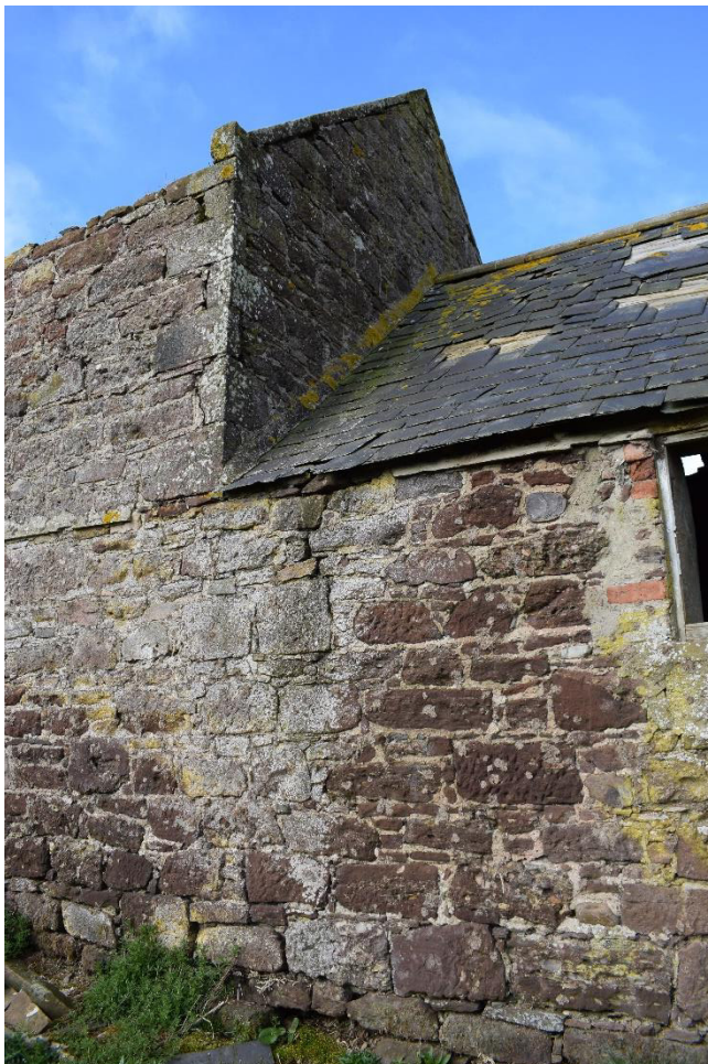
Illus 14 E wall Room 2 (right) and Room 3 (left); facing SW
