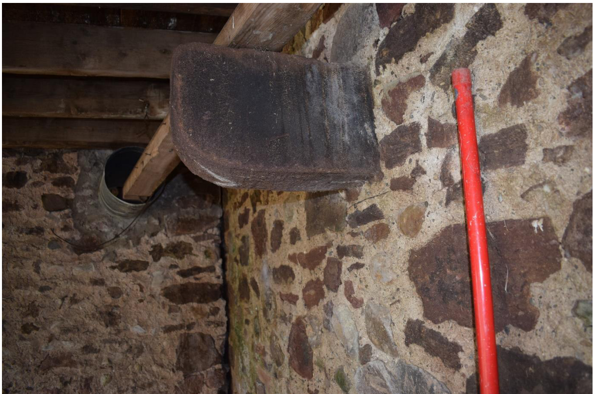
Illus 12 Room 3 sandstone corbel F6; facing NNE
