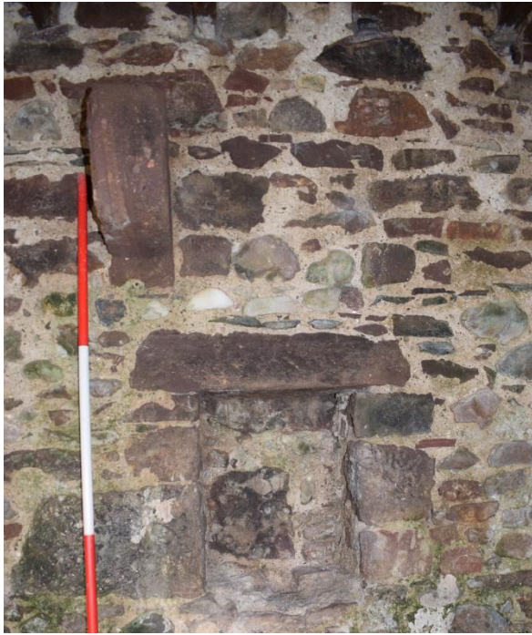
Illus 13 Room 3 E wall niche F3 with corbel F7 above; facing E
