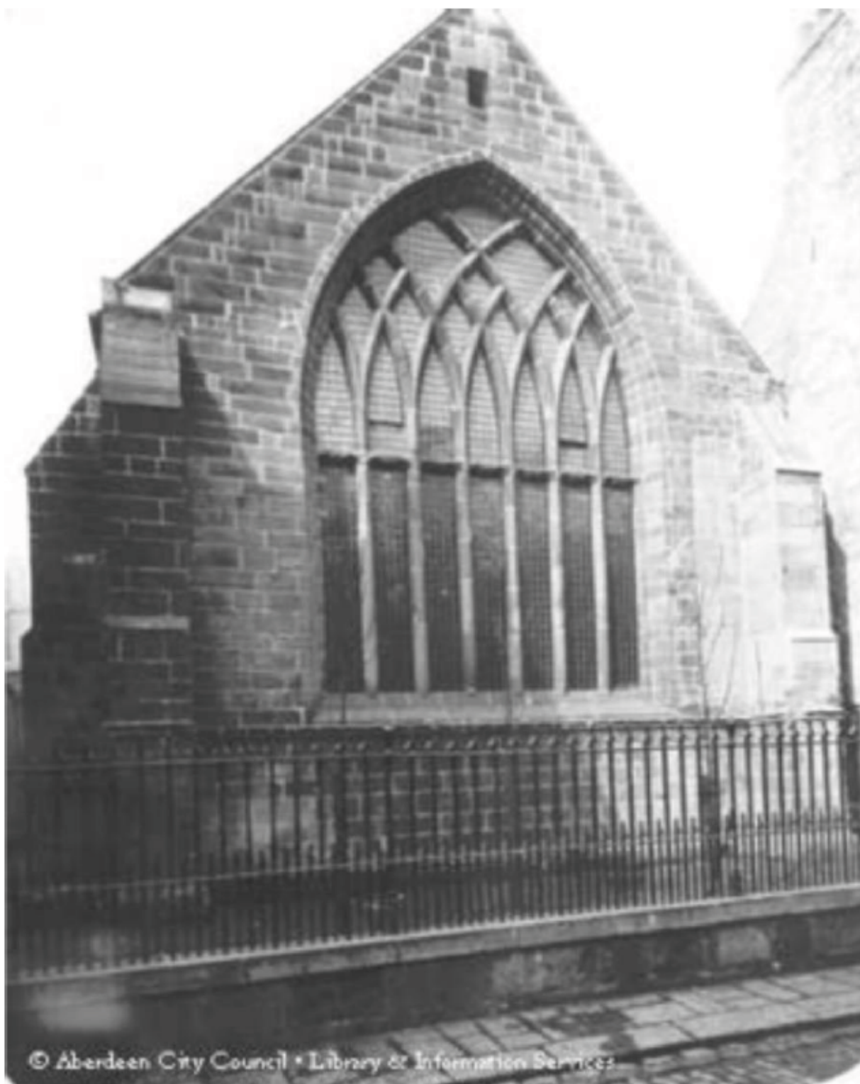
Illus 3 Old Greyfriars SE window rebuilt into the new church (W34); facing NW (copyright Aberdeen City Council Local Studies accessed through Silver City Vault online).
