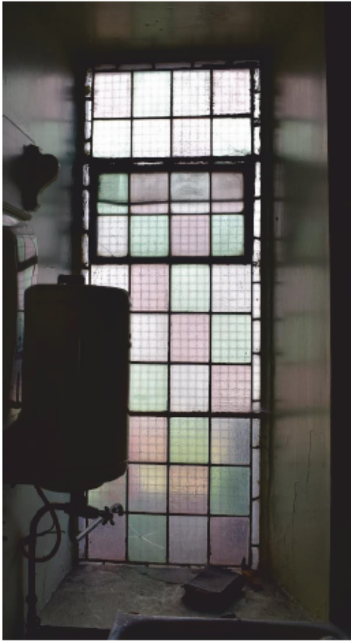
Illus 9 W31 SW half in Gents toilet cubicle
