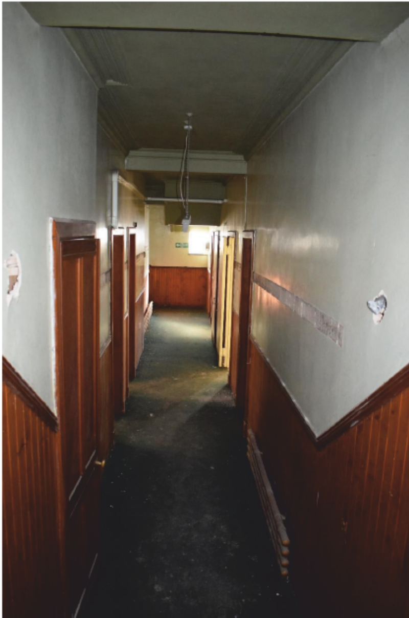
Illus 8 Room 6 lower ground floor corridor; facing SW
