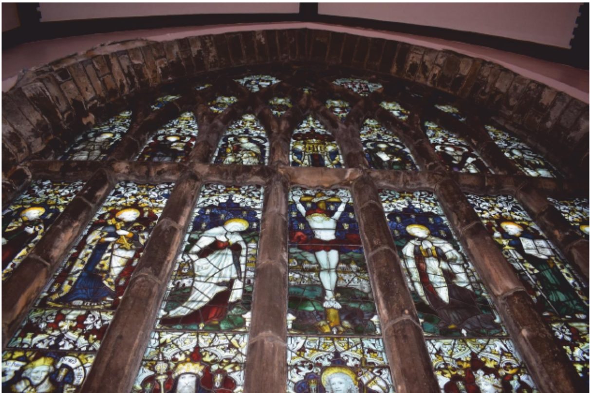
Illus 15 Detail of upper section of D34 showing sandstone tracery removed from SE window Old Greyfriars and rebuilt into SE wall of new church; facing SE
