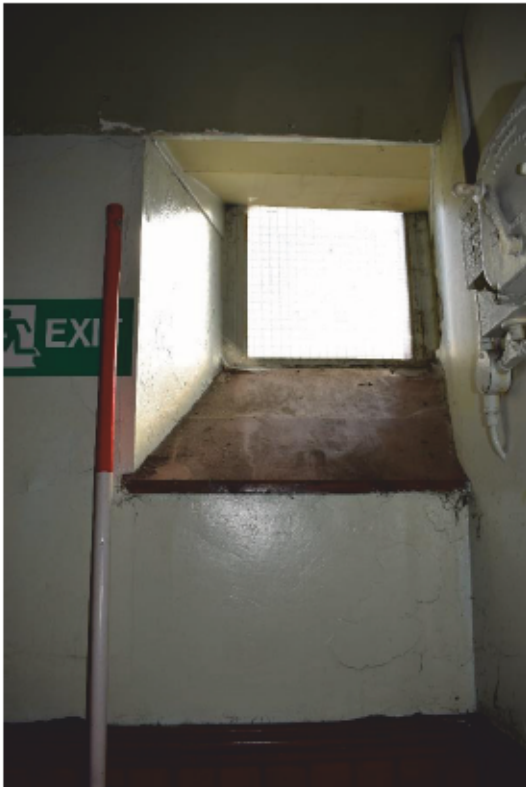
Illus 10 SW end of corridor Room 6 with W15 SE half; the window was divided by inserting wall for Ladies toilets (right); facing SW
