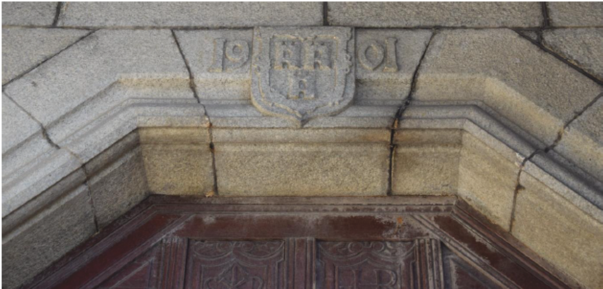
Illus 23 Detail of keystone in arched lintel above D3; facing SE
