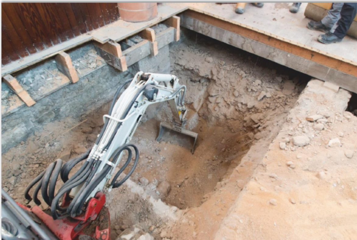
Illus 27 Test Pit 2 (TP2) adjacent to foundations of Marischal College (walling in upper left corner).
