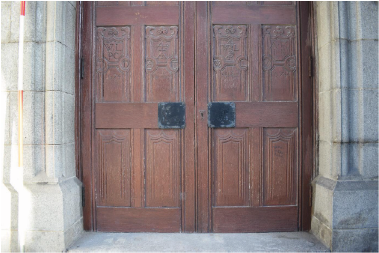
Illus 21 Door 3 reused wooden panels; facing SE
