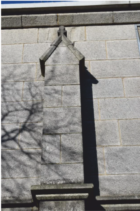
Illus 16 Detail of pointed top of decorative buttress F7 on SW façade of main church; facing NE
