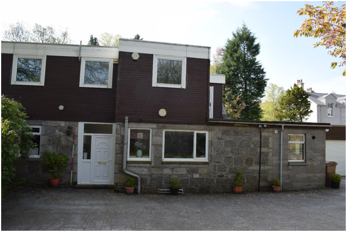
Illus 8 Inchgarth Steading NNW façade showing fragment of granite walling with modernized first floor and extension; facing SSE
