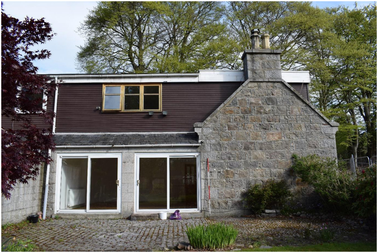
Illus 6 SSE façade of Lodge showing granite gable; facing NNW
