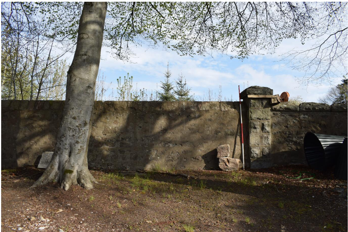
Illus 9 Wall with gatepost between Lodge and Inchgarth Road being retained; facing N
