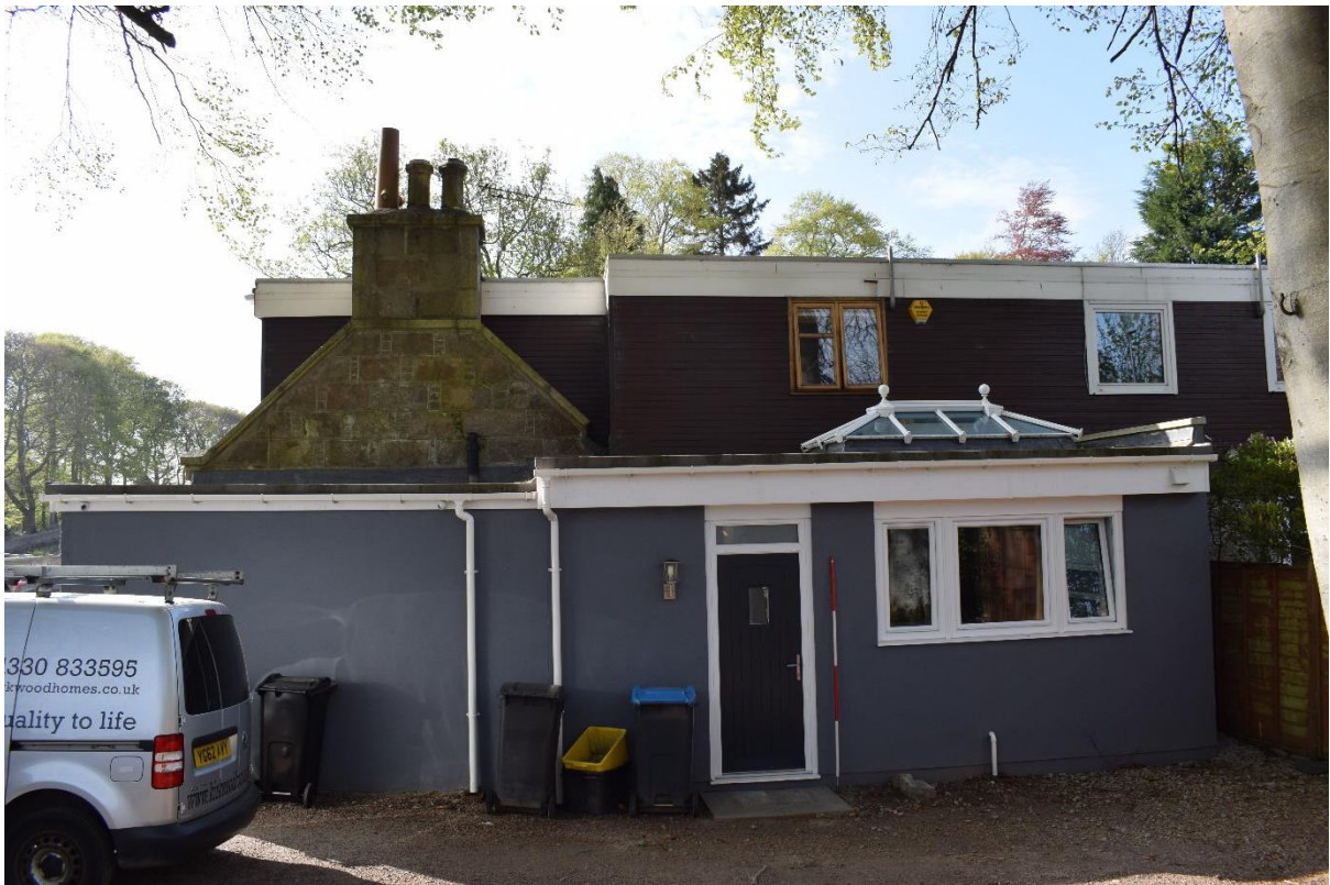
Illus 5 NNW façade of Lodge showing granite gable within heavily modernized exterior
