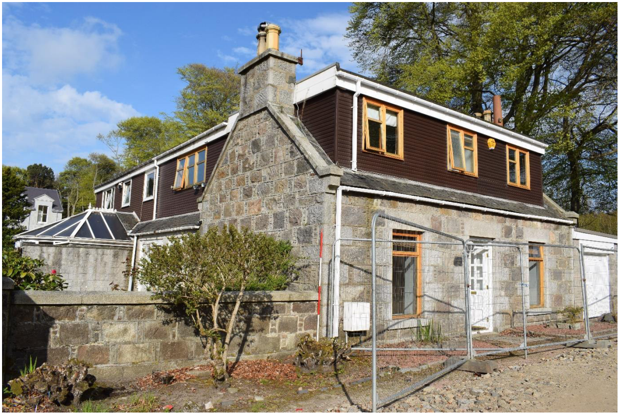
Illus 4 Inchgarth Lodge showing granite structure; facing NW
