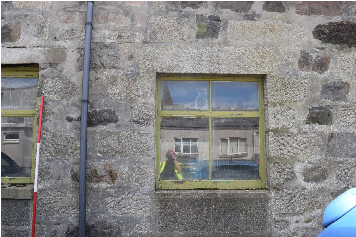
Illus 37 Building 6 N wall W33; facing S
