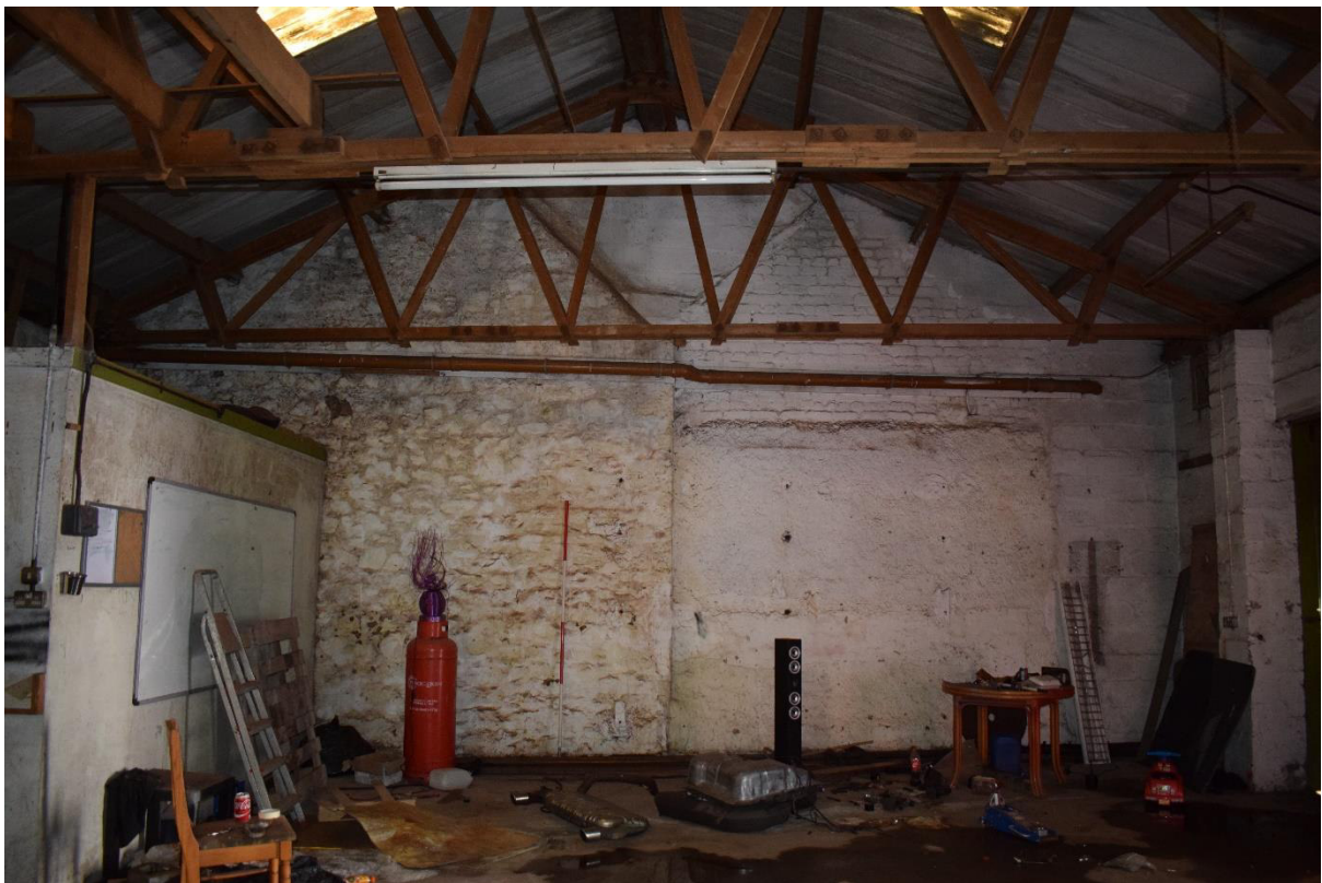
Illus 32 Building 4 W wall showing that the building was originally two structures and the N wall has been rebuilt (right); facing W
