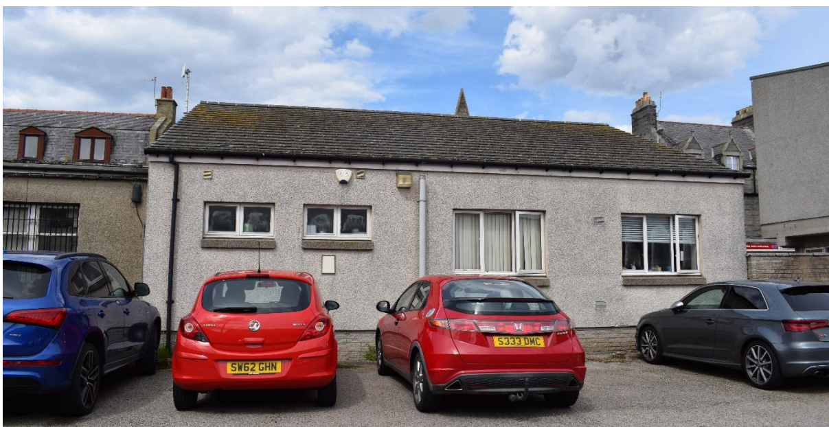
Illus 50 Building 7A rear south façade; facing N
