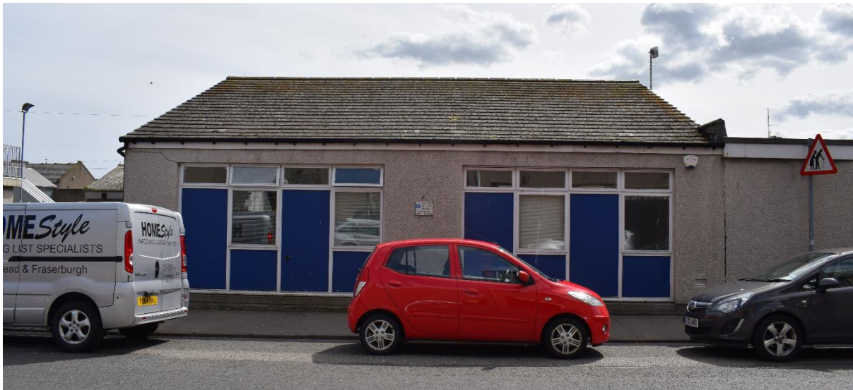
Illus 49 Building 7A north Mid Street façade; facing S
