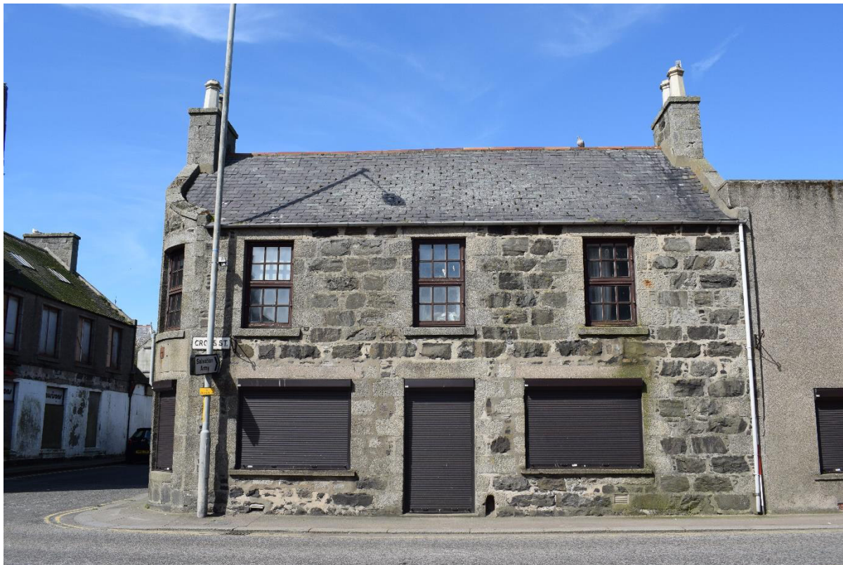
Illus 7 Building 1 E Cross Street façade; facing W
