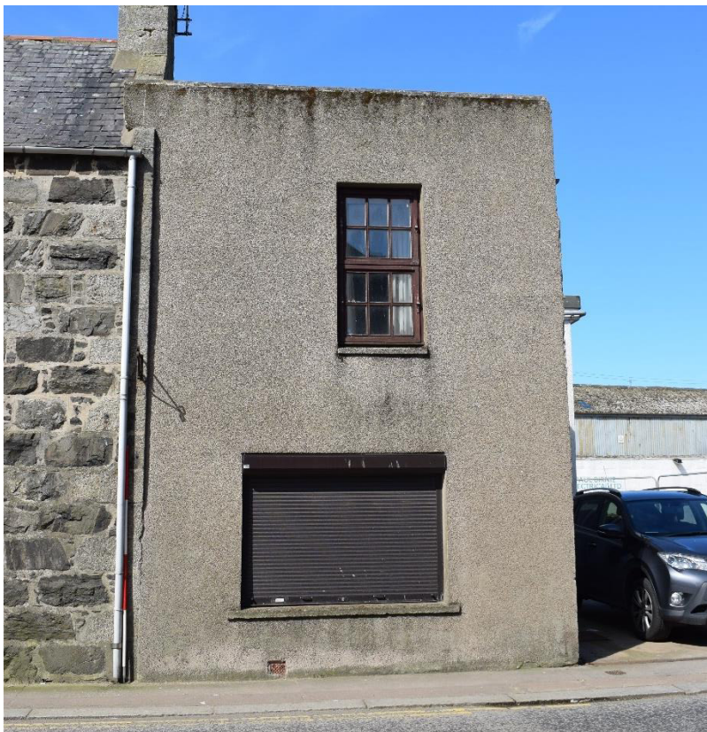
Illus 11 Building 1C east Cross Street façade; facing W
