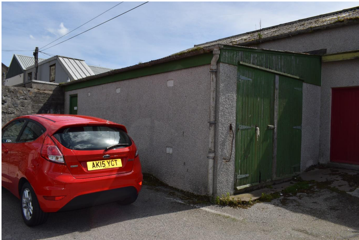
Illus 33 Building 5; facing SE
