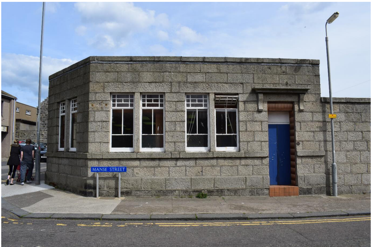
Illus 45 Building 7 W Manse Street façade
