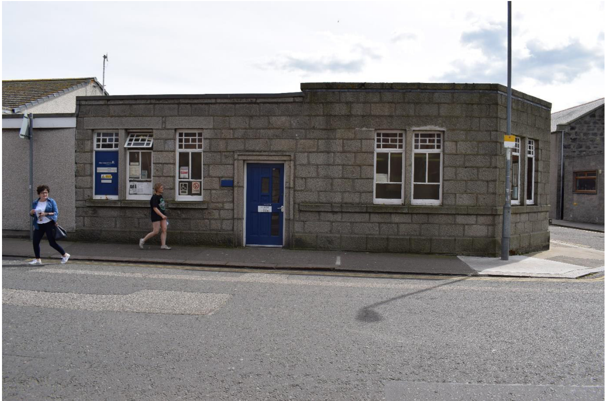
Illus 44 Building 7 north Mid Street facade
