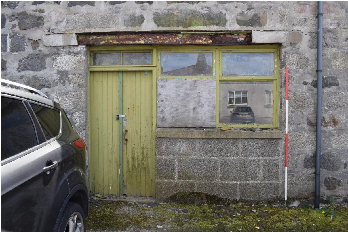
Illus 36 Building 6 N wall D4 reduce in size with glass and breeze blocks; facing S
