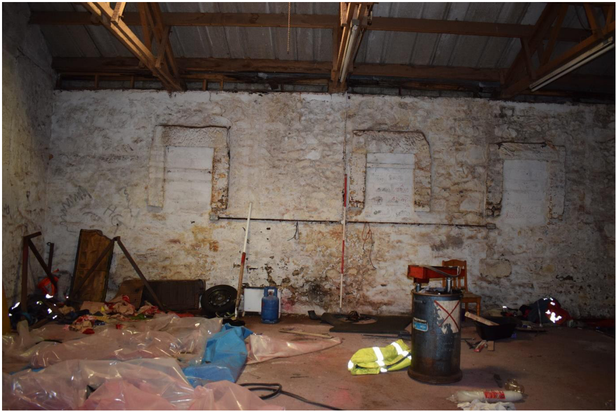
Illus 29 Building 4 S wall interior showing older section of building and fireplaces F12, F13, F14 (l-r); facing S
