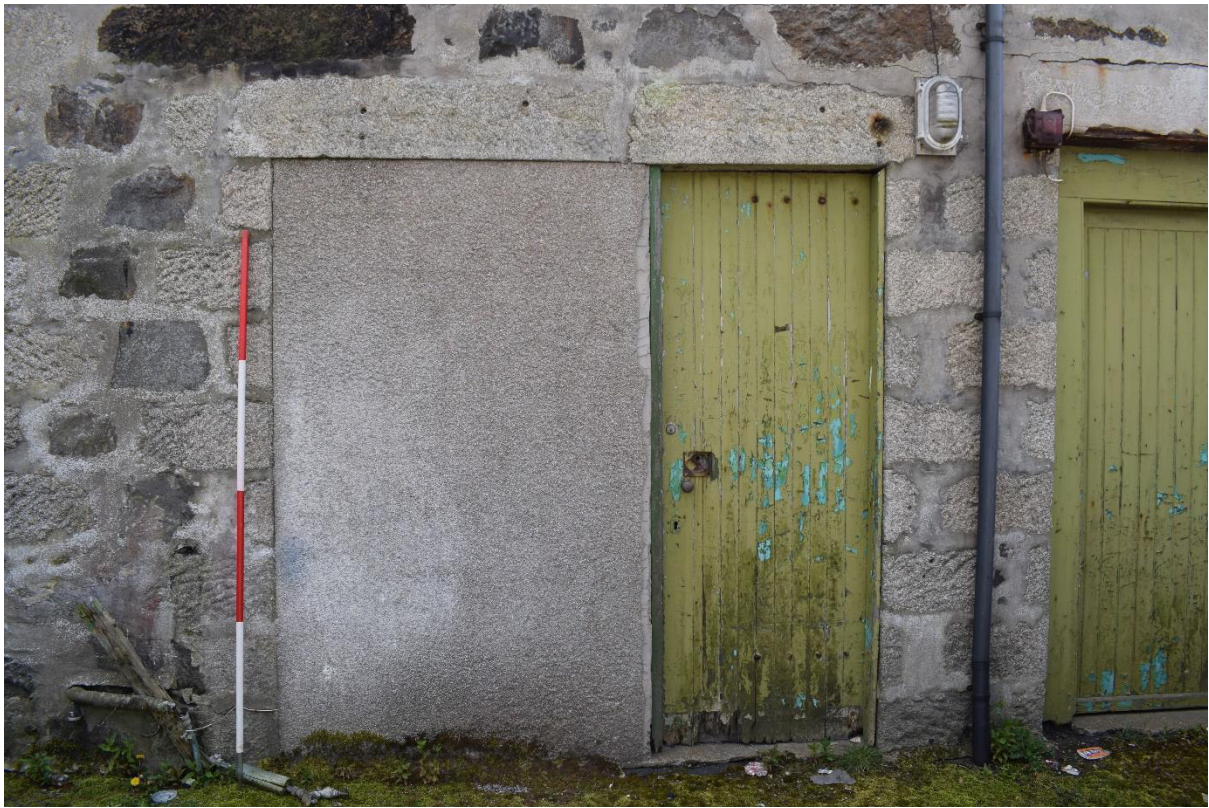
Illus 38 Building 6 N wall D5 showing reduction in with using harled concrete blocks; facing S
