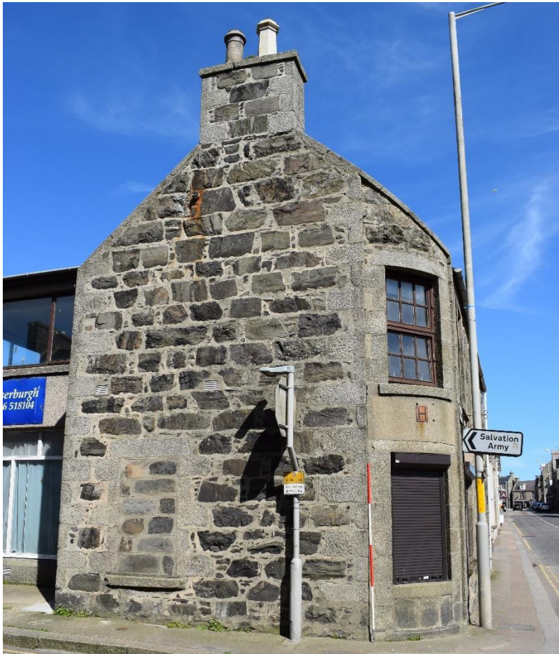
Illus 8 Building 1 south (Frithside Street) façade; facing N
