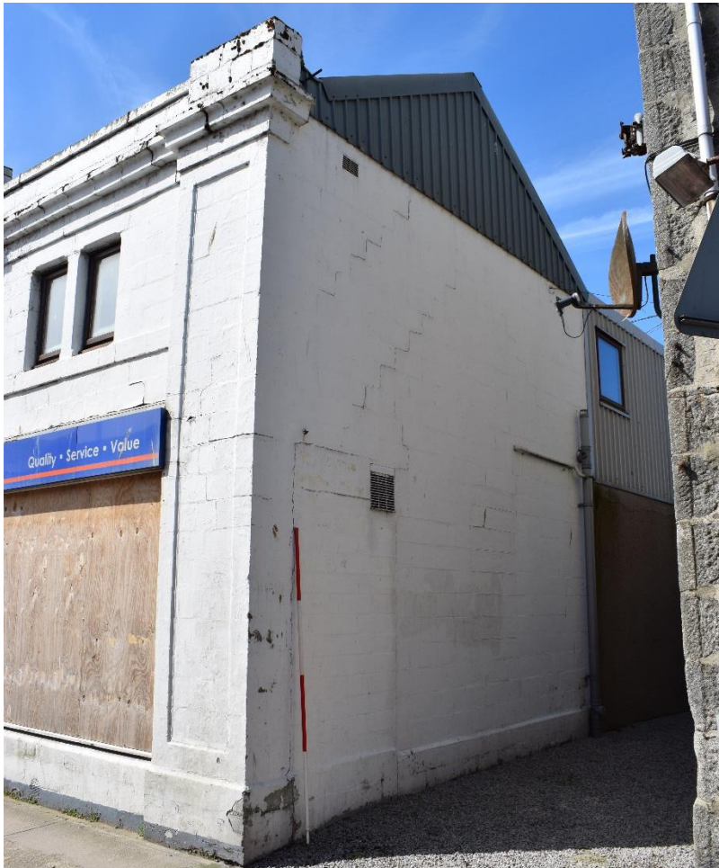
Illus 22 Building 3 N wall with blocked door D11; facing SW
