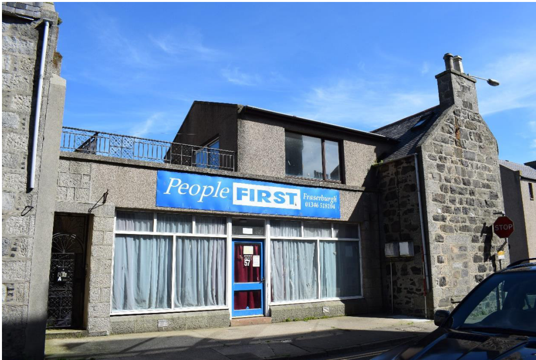
Illus 10 Building 1A south Frithside street façade; facing NNE
