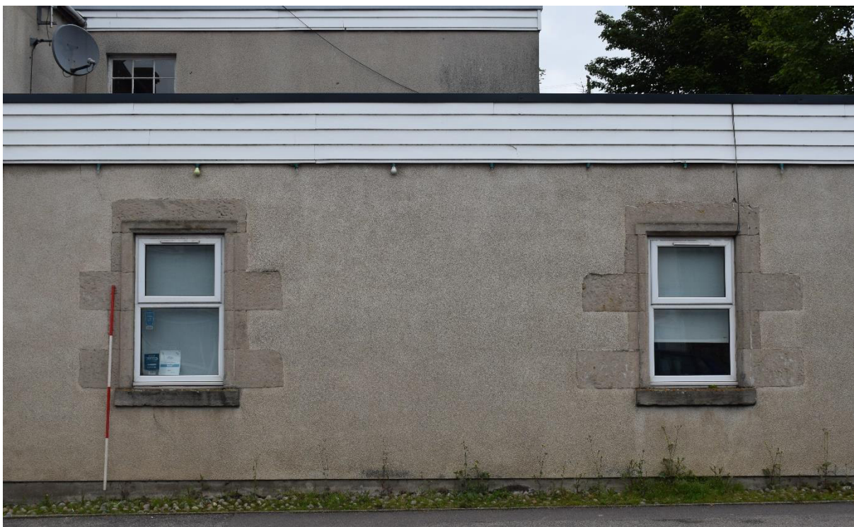
Illus 17 Phase 2 extension SW front façade sandstone windows W18 and W19
