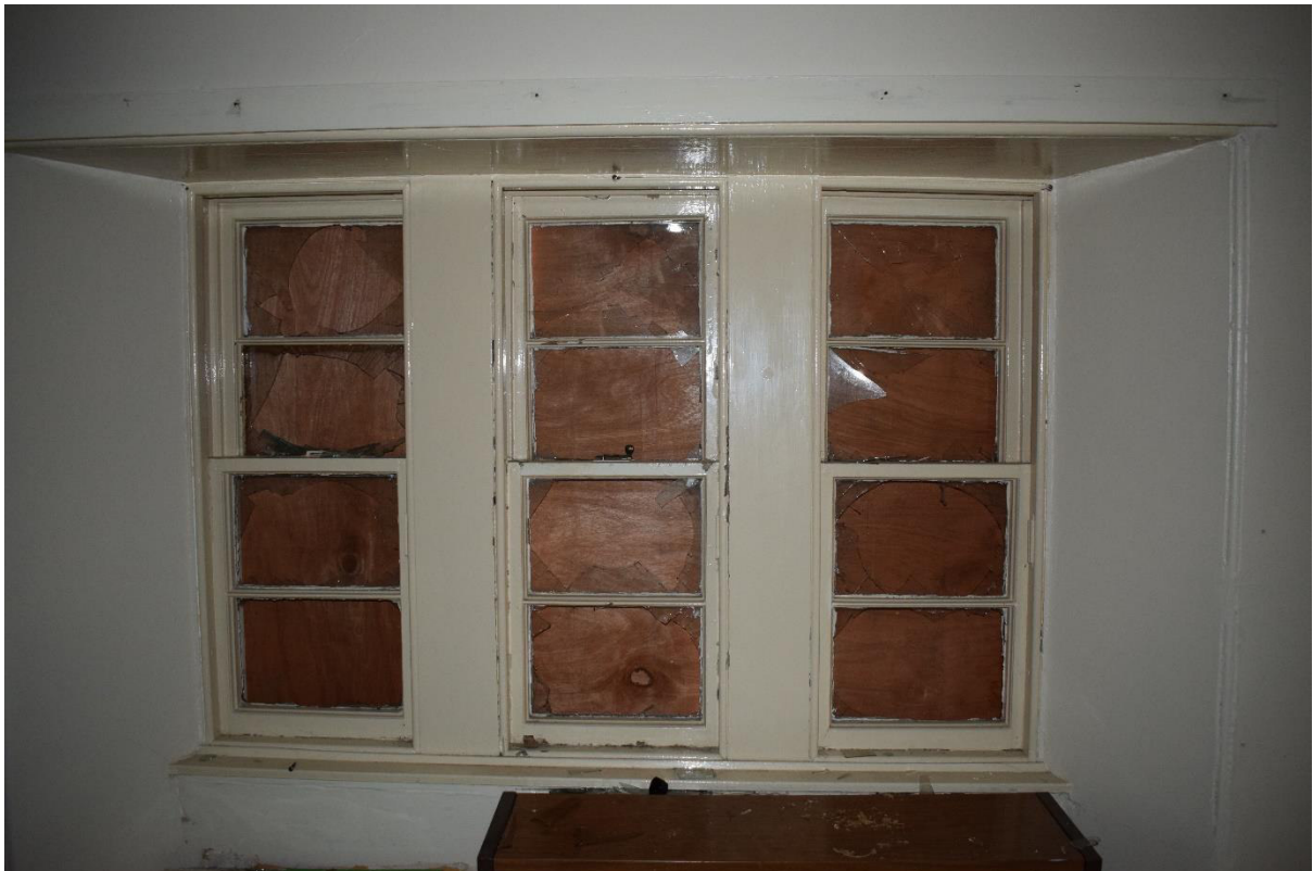
Illus 9 First floor corridor Phase 1 window W14 interior
