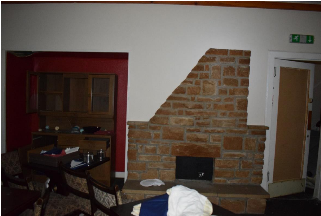
Illus 15 Room 8 NW wall with chimney breast and fireplace F15; facing NW
