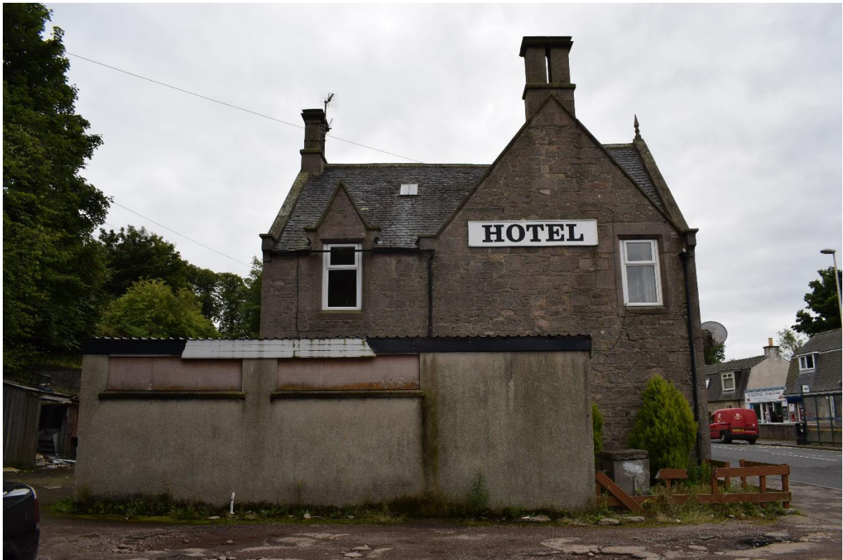
Illus 11 NW façade with W12 (top left) W13 (top right) and late 20 th -century shop extension (bottom); facing SE
