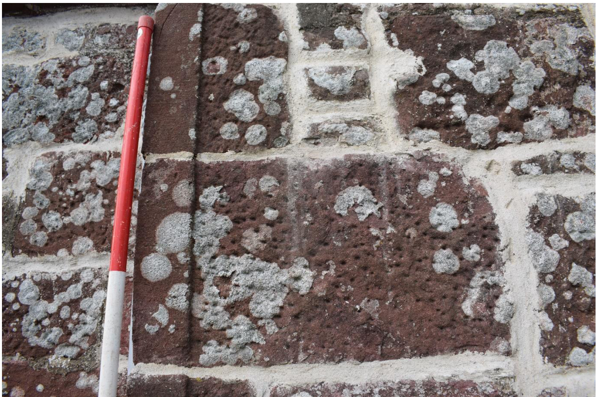
Illus 14 Sandstone quoin with pecked dressing, SE corner of church; facing W
