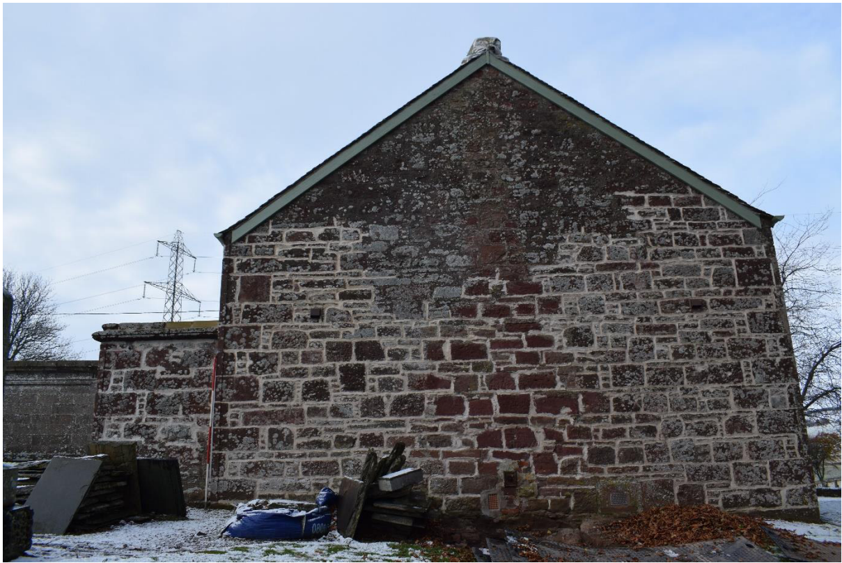
Illus 13 East gable; facing W
