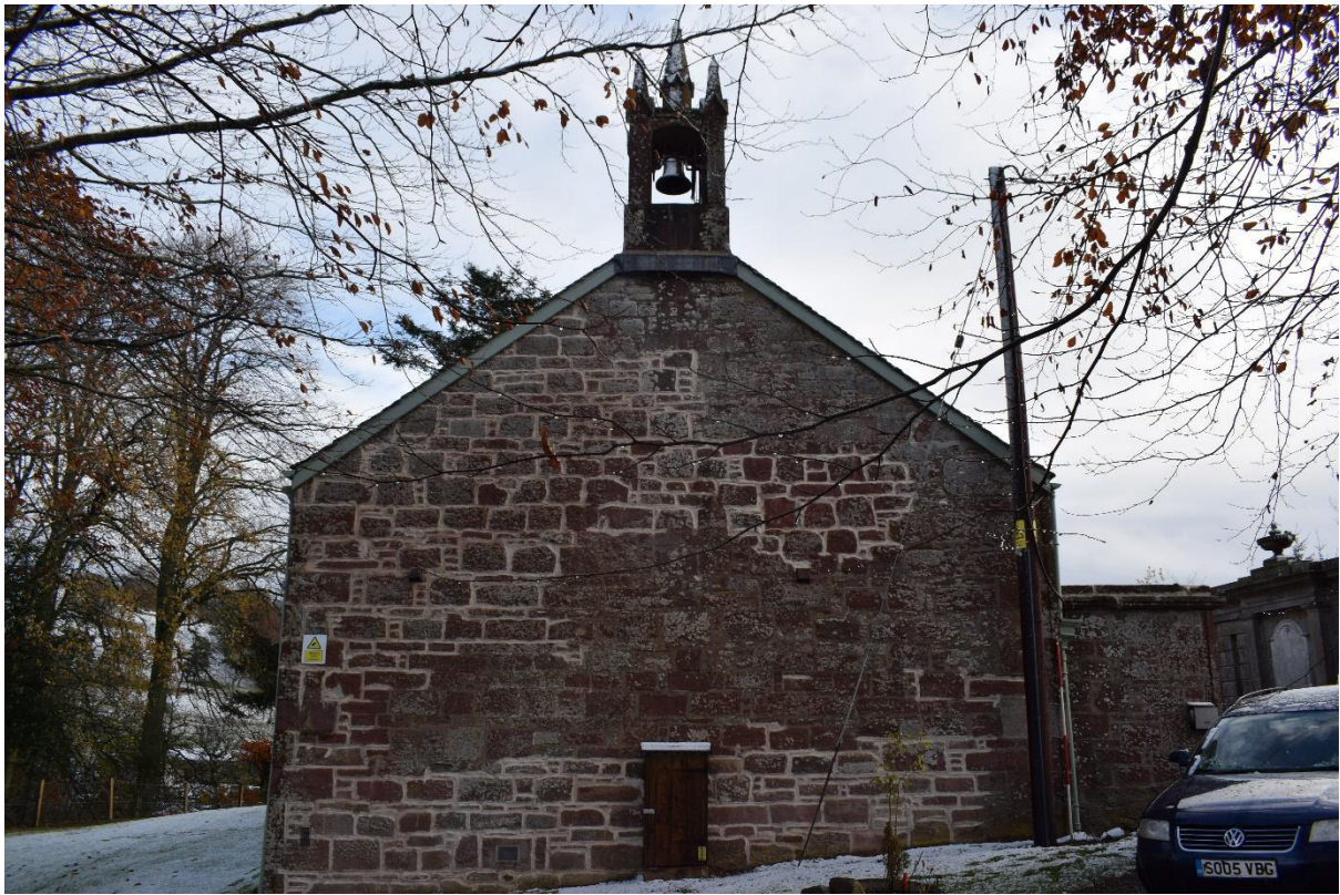
Illus 15 West gable; facing E
