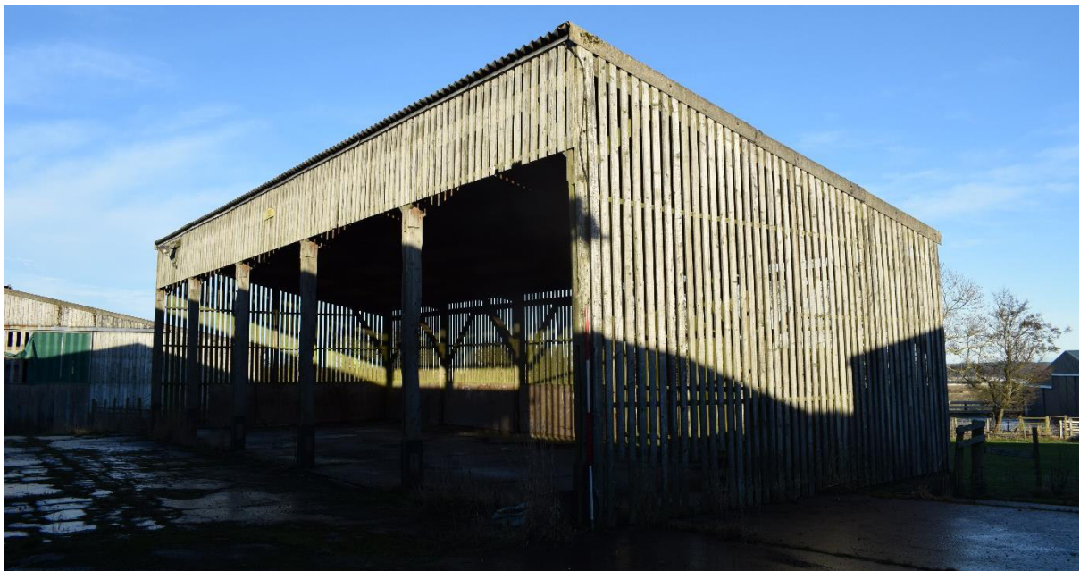
Illus 39 Building 8; facing N
