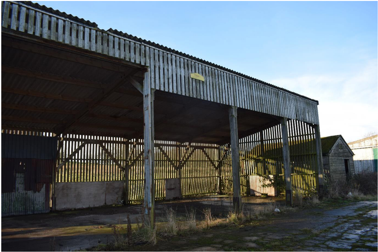
Illus 36 Building 7A NW end; facing NW
