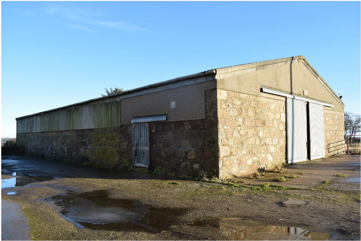
Illus 20 Building 4 from SW showing granite construction
