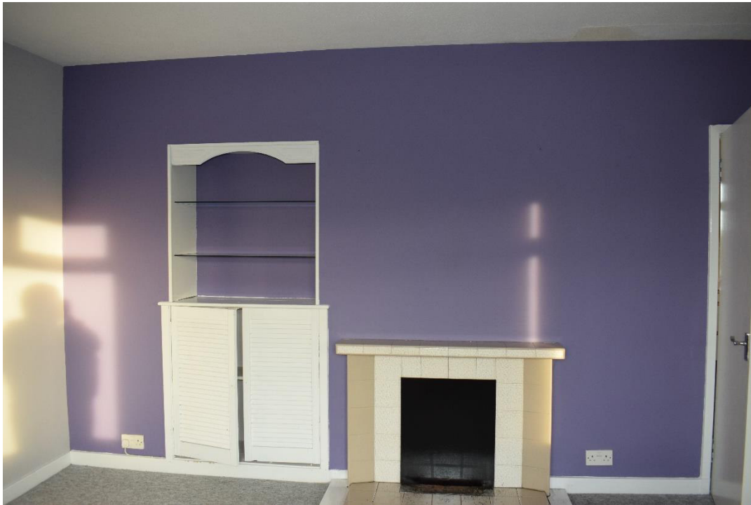
Illus 9 Building 1 Room 2 N wall fireplace F7 and alcove F8 (left); facing N
