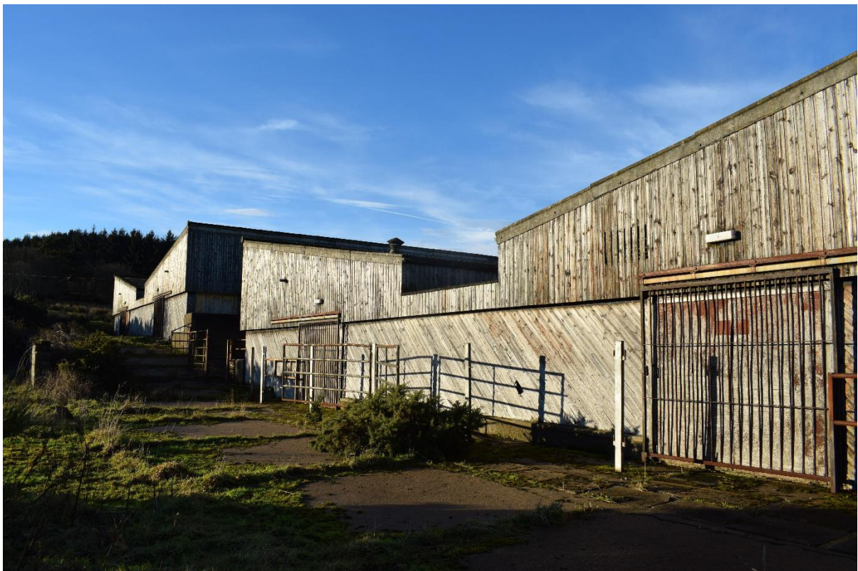
Illus 31 Building 7 SE wall; facing W
