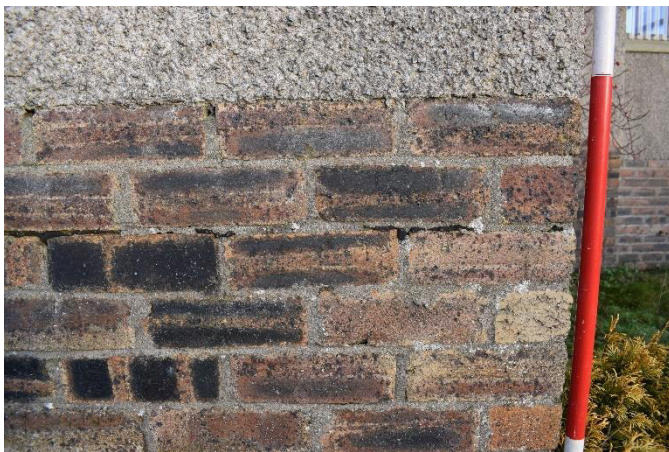
Illus 7 Building 1 S wall brick details; facing N
