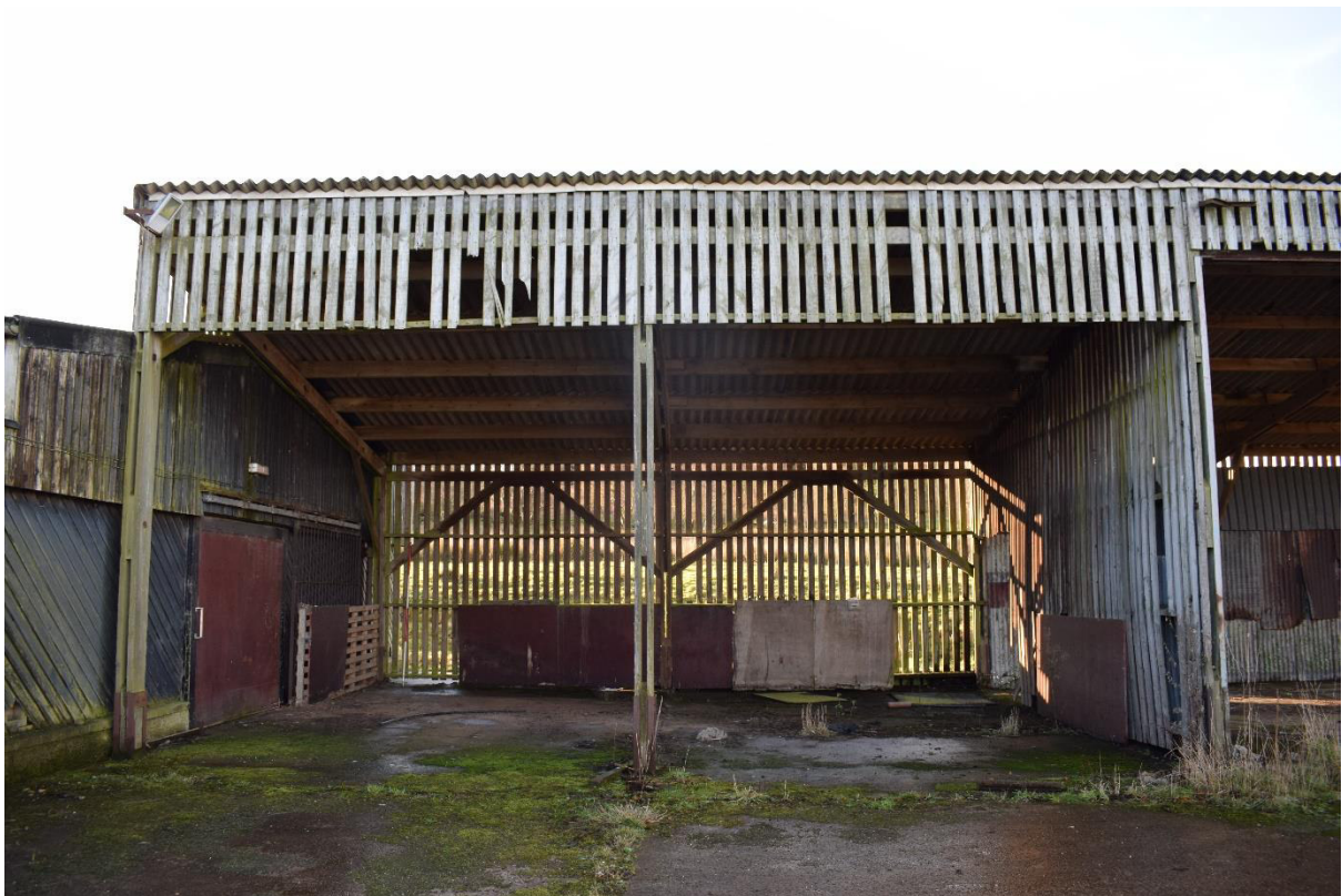
Illus 35 Building 7A SE end; facing SW
