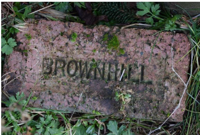
Illus 8 Building 1 Brownhill brick used in base of building
