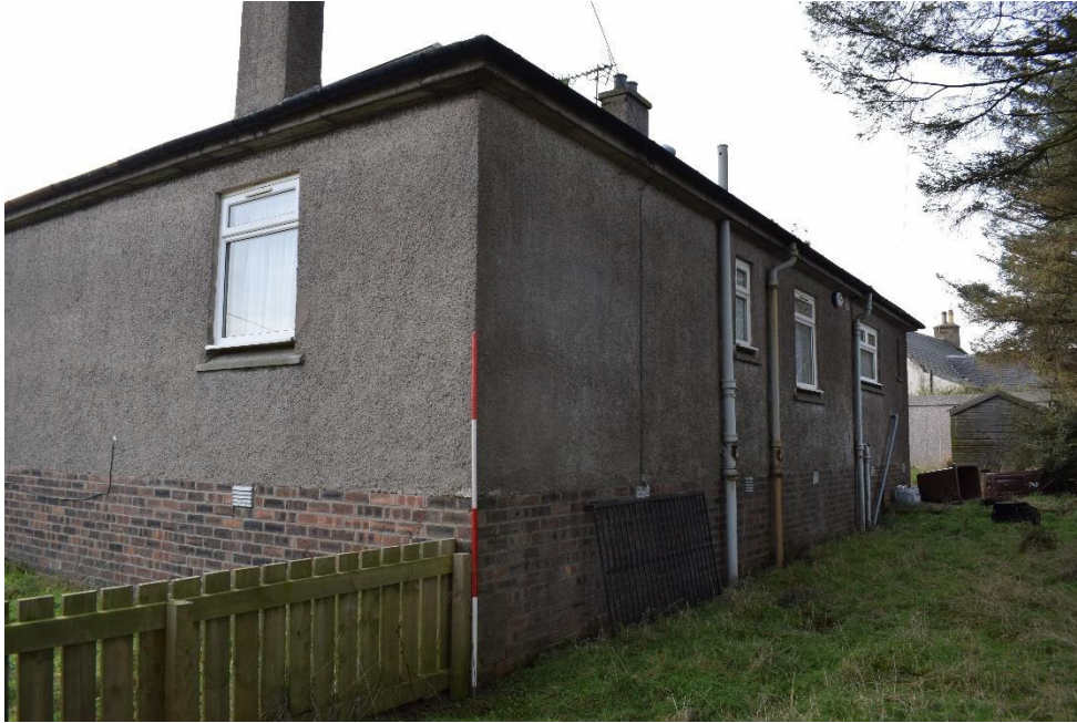
Illus 13 Building 2 from NE
