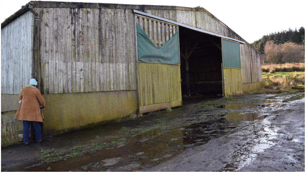
Illus 41 Building 9 NW wall with D16; facing SW
