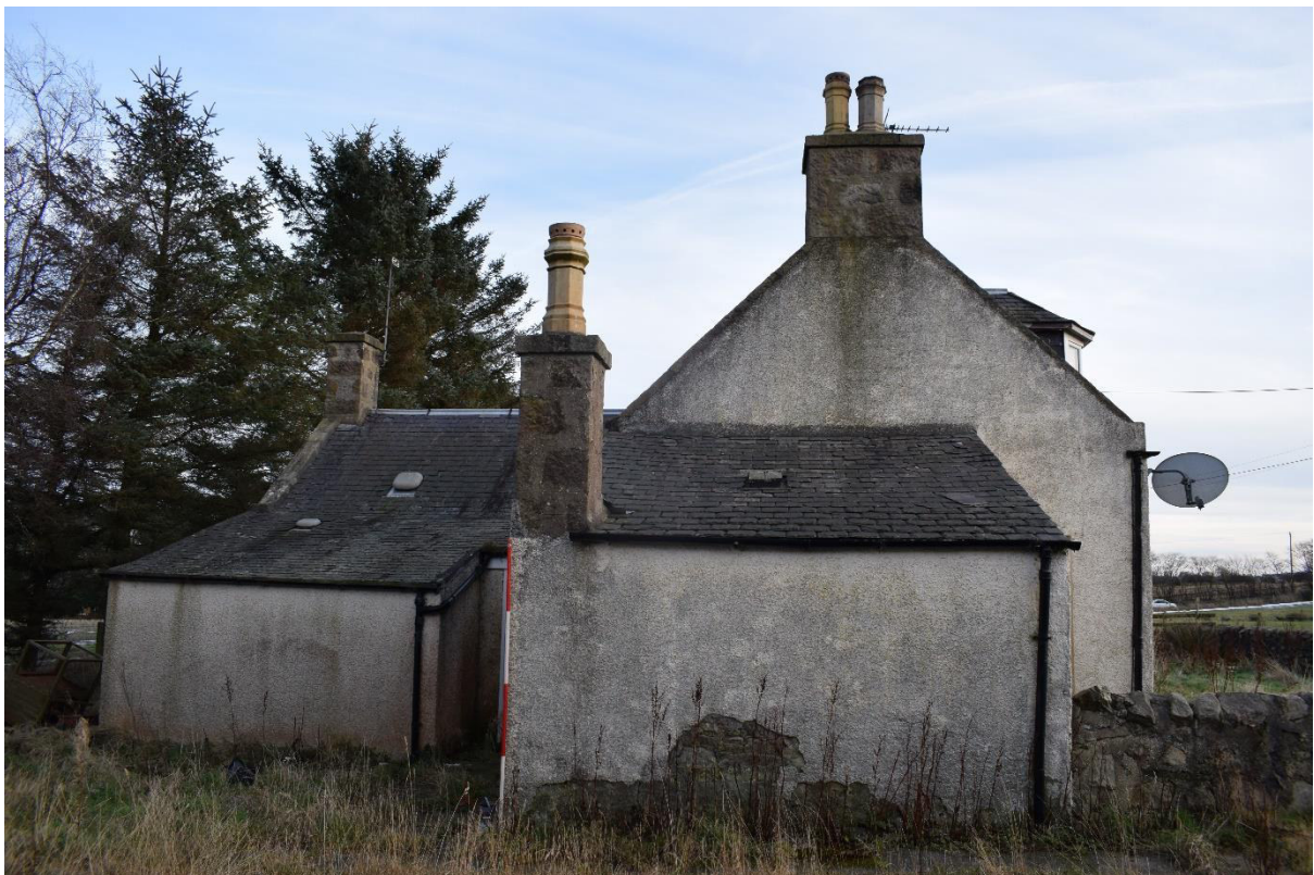
Illus 17 Building 3 W wall showing Phase 2 lean to (left) workshop with external chimney F19 (centre) and main cottage W gable (right); facing E
