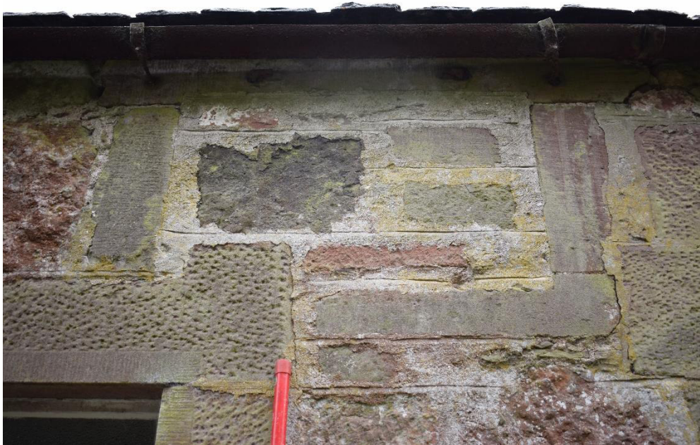
Illus 6 Phase 1 blocked window W17 above W16; facing E
