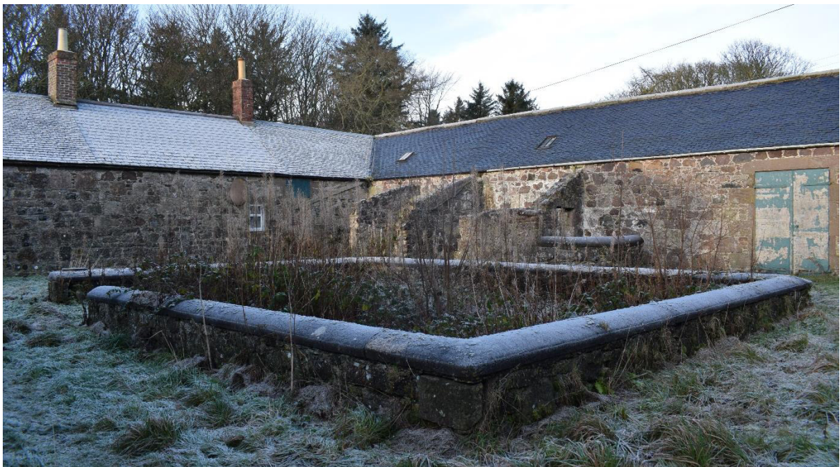
Illus 19 N courtyard low walled enclosure F9; facing NW
