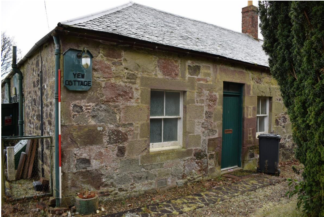
Illus 5 Cottage W façade W wing N end W16 (left), D6, W18 with Phase 1 upper window W17 blocked above W16; facing SE
