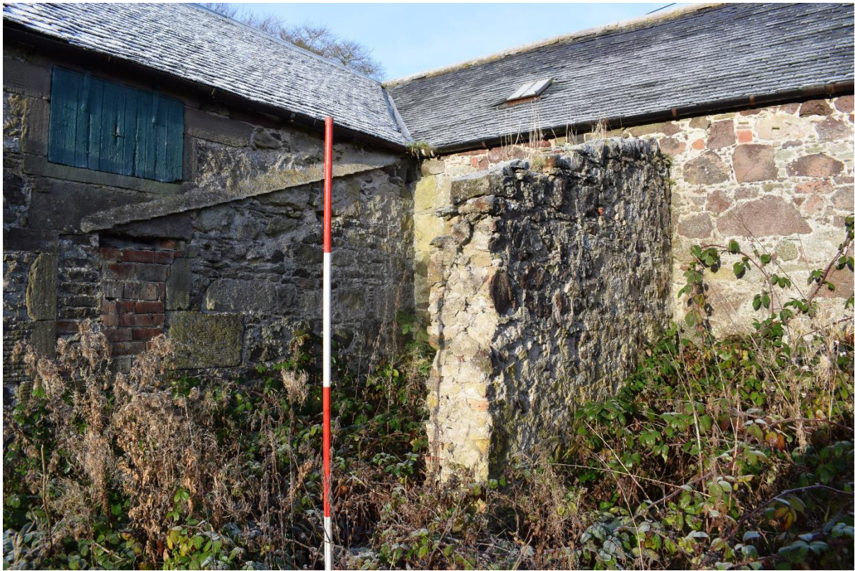
Illus 18 Room 9 (left) and Room 10 (right); facing NW
