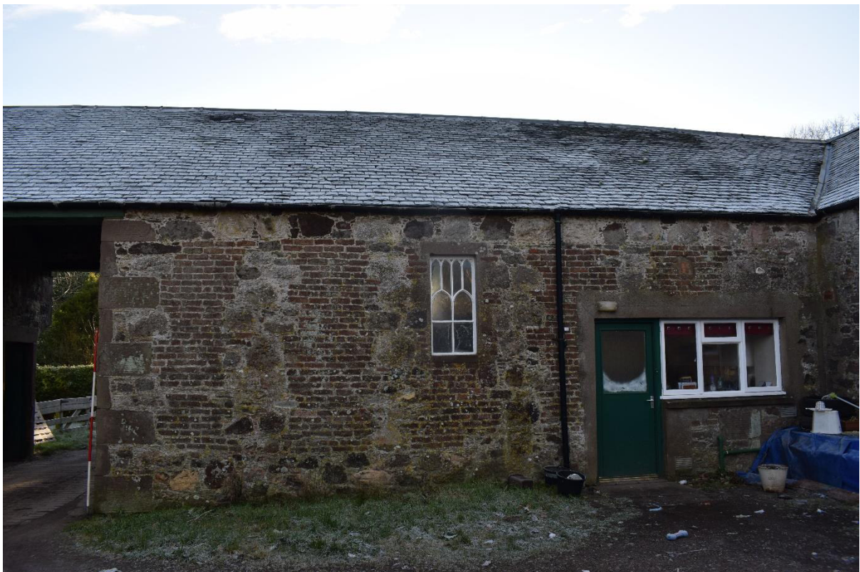
Illus 8 South wing N wall W end D3 (left) rebuilt wall sections F27, F28, F29 around window W47 and modern door and window into cottage D17/W48; facing S
