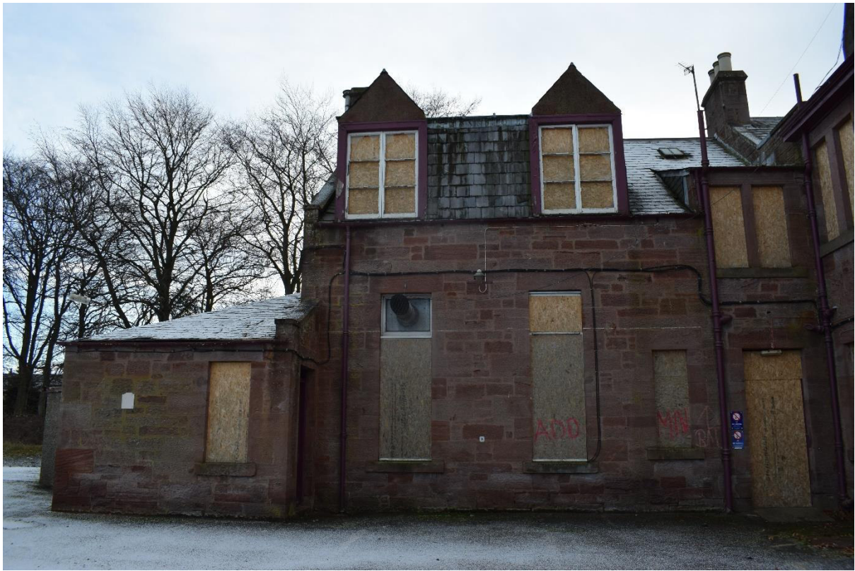
Illus 9 Phase 1 NE wing; the lintels and sills and stonework are identical to the main building and so considered built in one phase; facing SE
