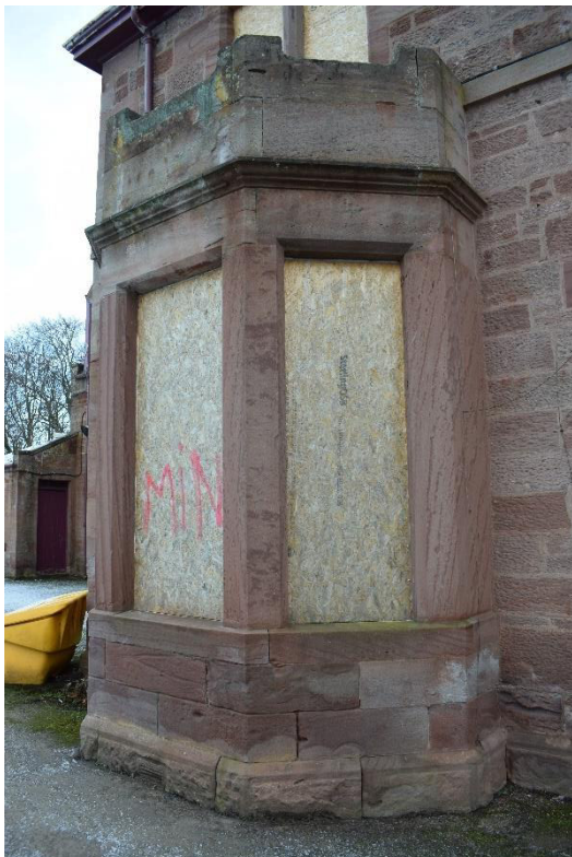
Illus 10 Bay window W10 showing sandstone block construction, rusticated sandstone base course and crenellated top; facing E
