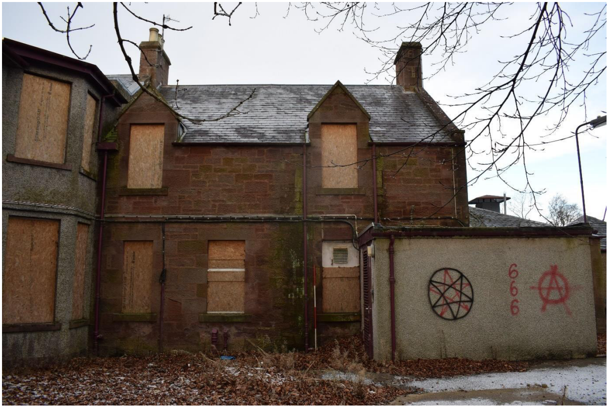
Illus 14 Phase 1 NE wing (centre) with Phase 3 SW extension (left) and Phase 4 switch room (right); facing NW
