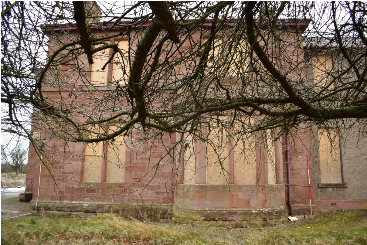
Illus 8 Phase 1 SW façade with bay window W24 (centre); facing NW
