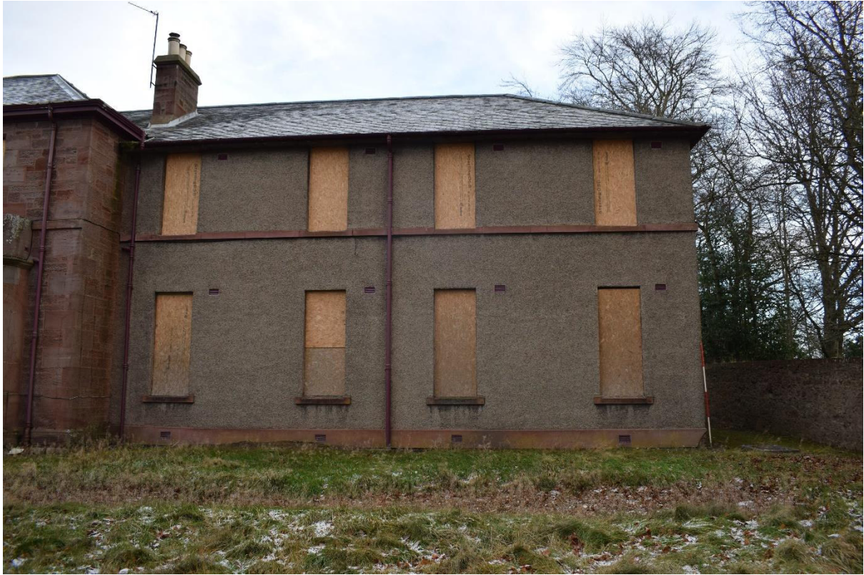
Illus 16 Phase 3 SE wing SW wall; facing NE
