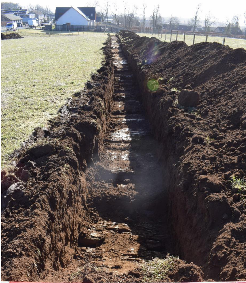
Illus 6 N end Trench 2 showing rocky clay natural and undulating silty areas of former palaeochannels; facing SSE
