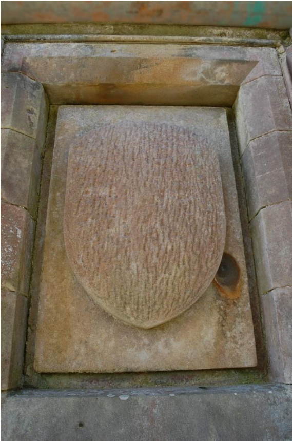
Illus 68 Sandstone plaque P1. Sandstone shield in rectangular border with hood moulding. The shield is roughly tooled and convex; facing W
