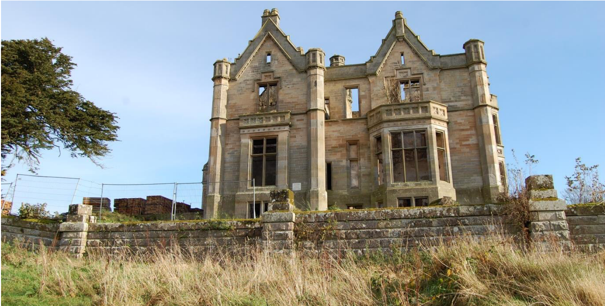
Illus 72 West façade with buttressed terrace walls (below); facing E
