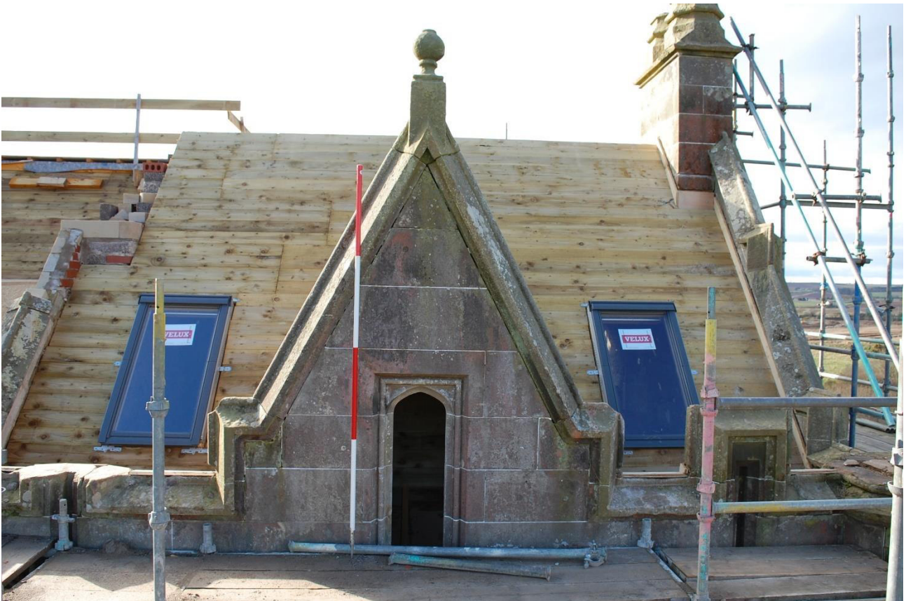
Illus 42 Room 48 Gablet with decorative finial and W32B; facing S
