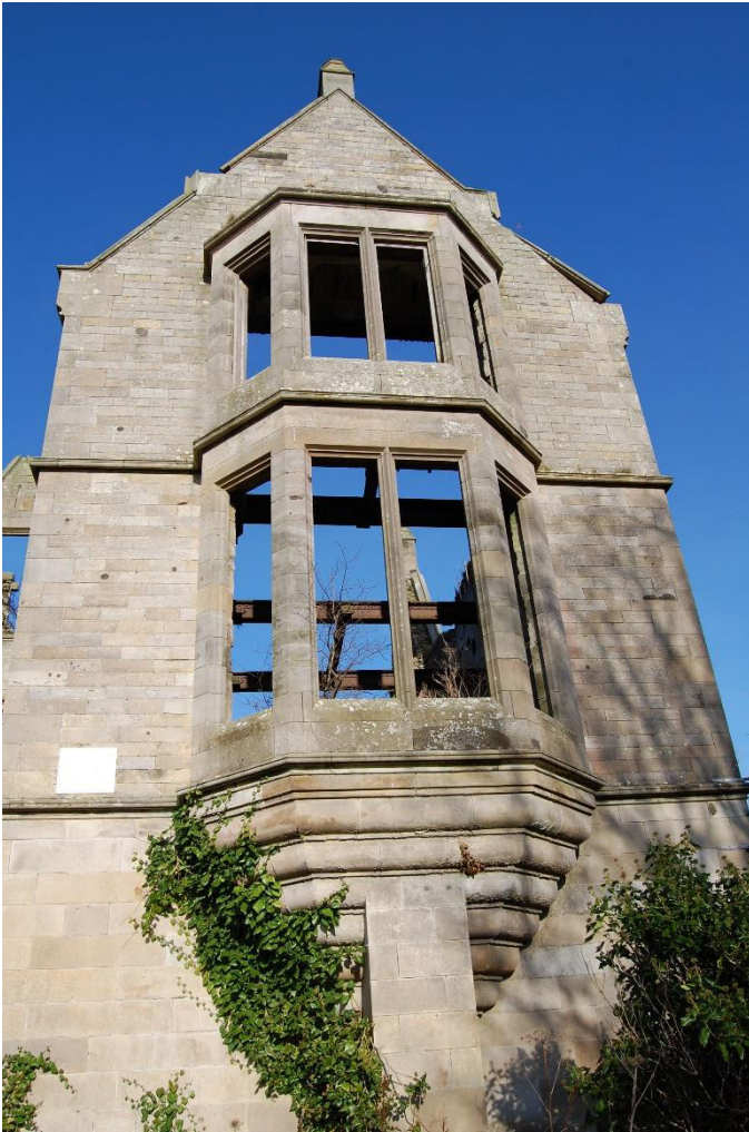
Illus 49 Room 15 (bottom), Room 32 (centre), Room 46 (top) oriel window W15/A east end south façade; facing N
