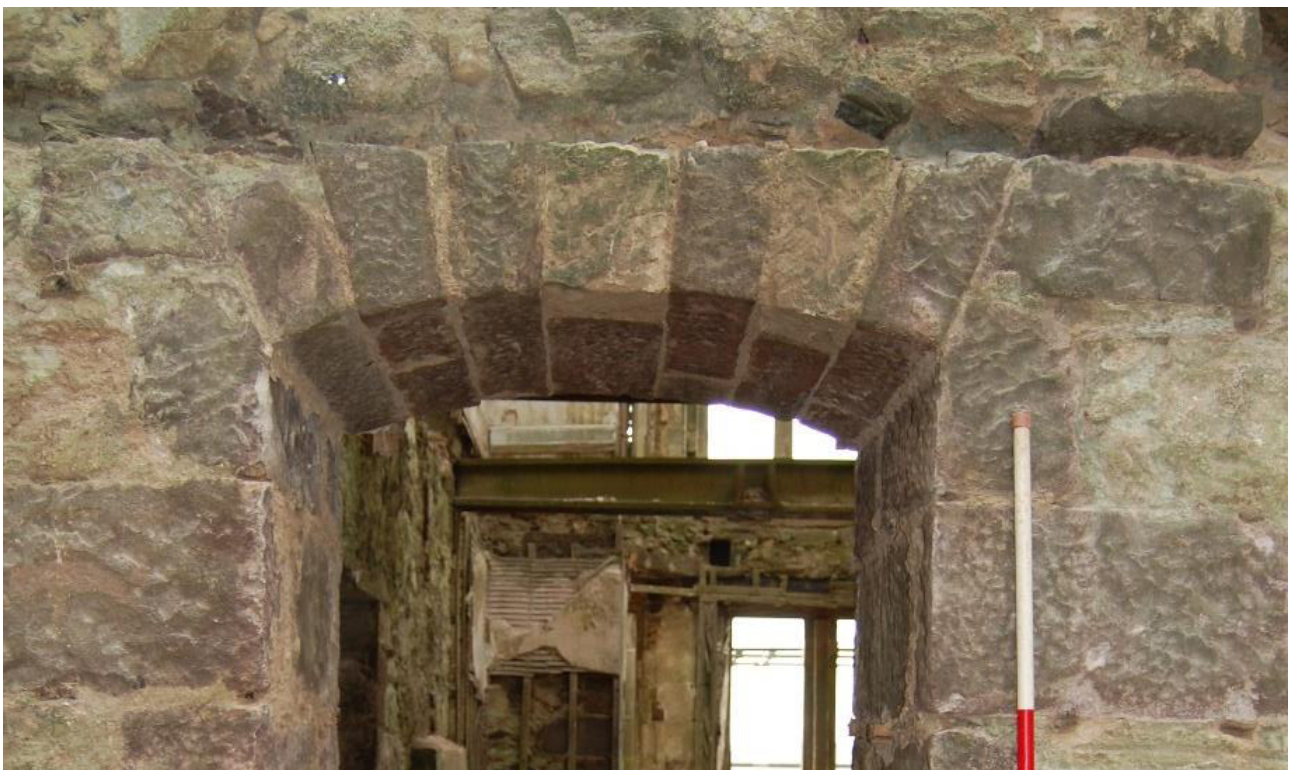
Illus 20 Stone arched lintel over Room 7 Door D11; the Phase 2 lintels are of brick
