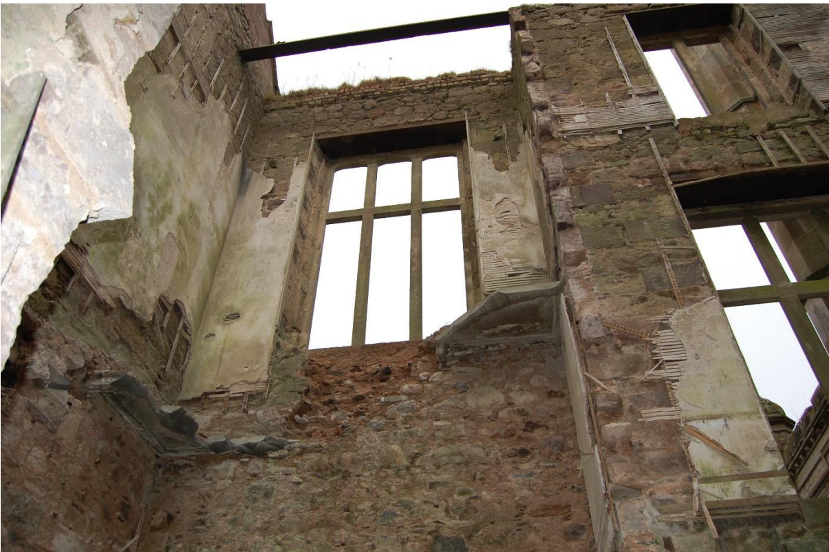
Illus 63 N wall Room 17 with remains of sandstone slab Stair 2 (centre); facing N
