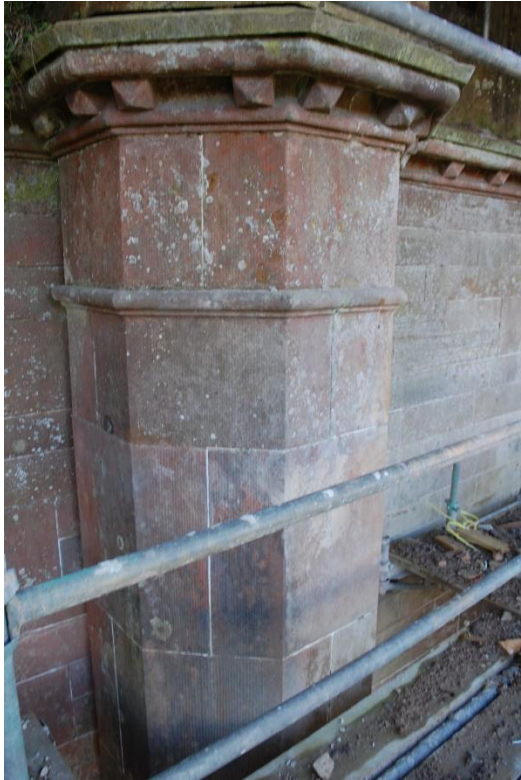
Illus 65 Top of F30 chimney; facing SW
