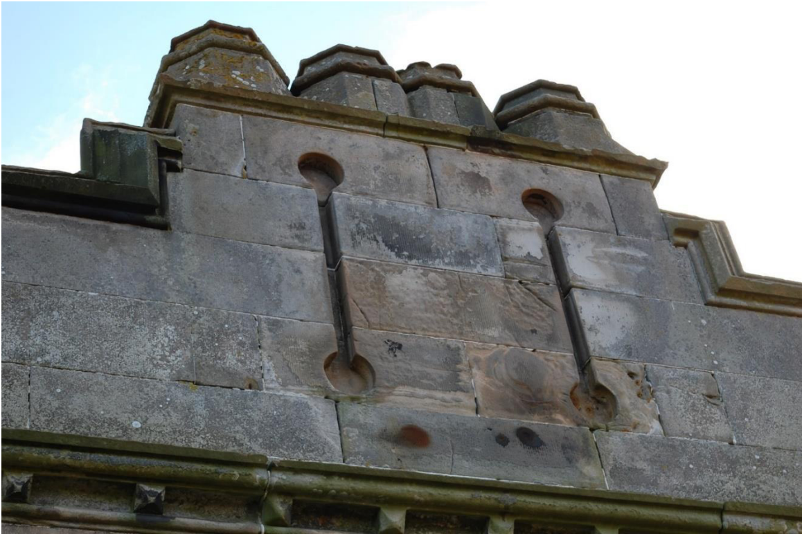
Illus 43 Tower decorative arrow slits F46; facing E
