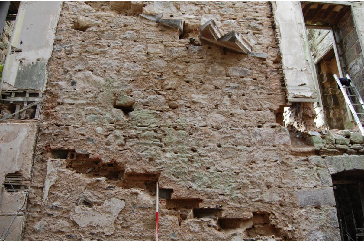
Illus 62 Scar after removal of Stair 1 showing remains of sandstone flags; south wall Room 7 with D13 (right); facing S
