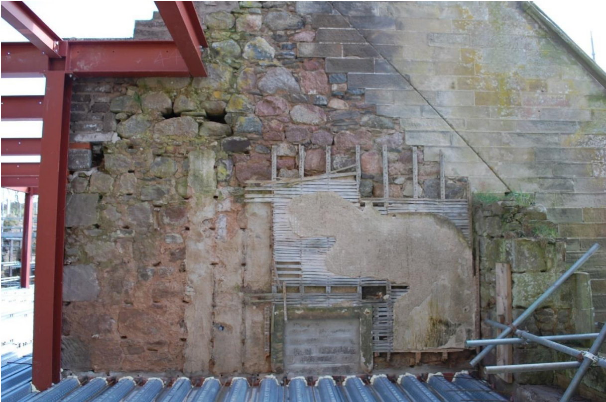
Illus 47 Room 57 E wall fireplace F13 with chimney F70 above with ashlar sandstone Phase 1 and Phase 1 roof raggle; facing E
