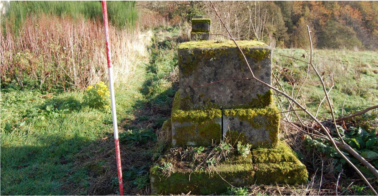
Illus 74 Detail of buttresses for terrace wall; facing E
