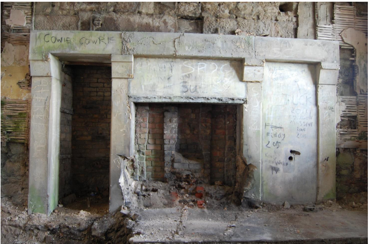
Illus 16 Room 3 concrete and brick fireplace F26; facing E
