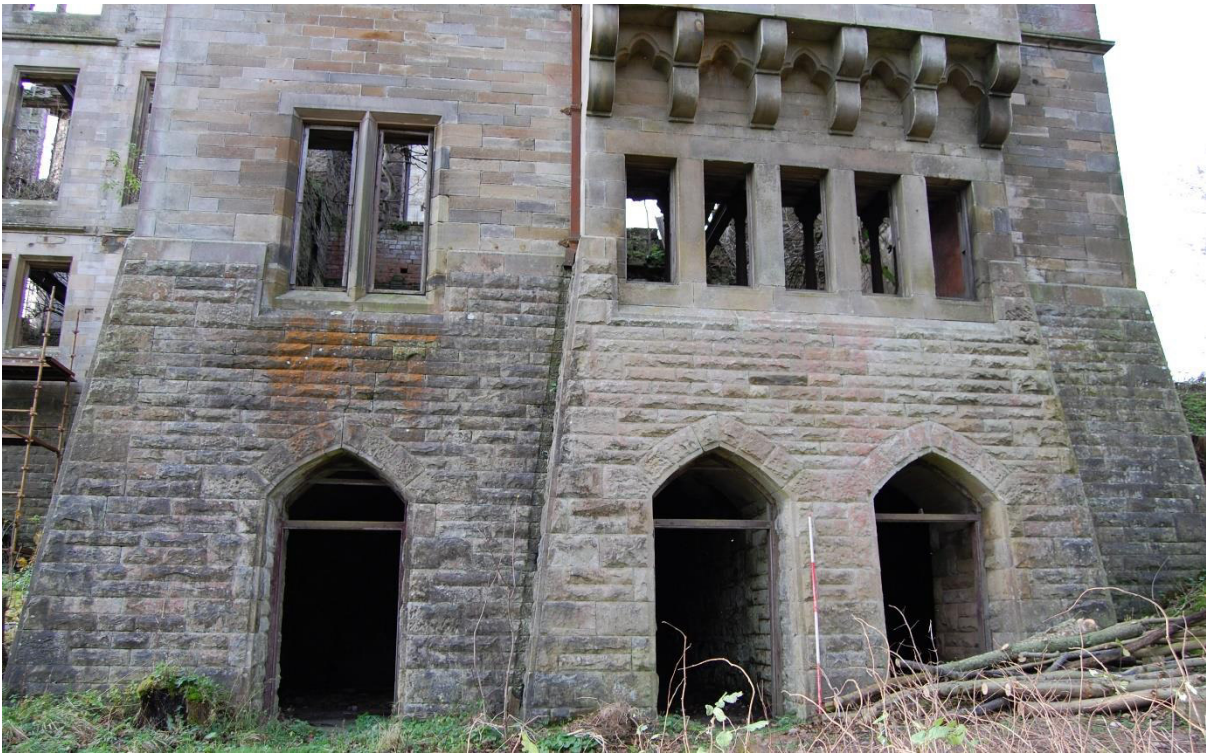
Illus 57 East wall showing three entrances (D2, D3, D4) into stone-lined brick-vaulted cellars (Rooms 66, 67, 68) probably used for preparation of game and other foodstuffs; windows W21, 22, 23 above; facing W
