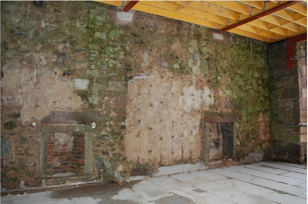
Illus 39 Room 39 was divided into 2 rooms with 2 fireplaces on E wall F76 (right) F8 (left); facing SE
