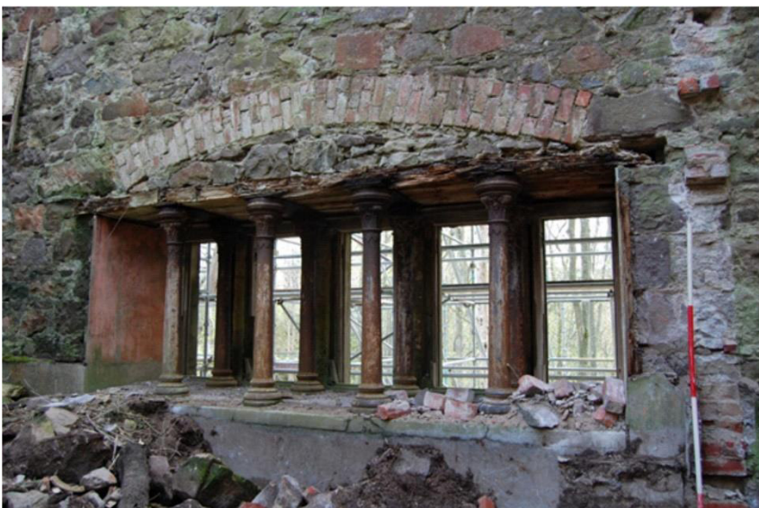
Illus 50 (left) Room 16 E wall window W24 with brick relieving arch and cast iron supports (right) Rooms 16 and 19 on 1882 plan with window supports arrowed ( copyright RCAHMS )
