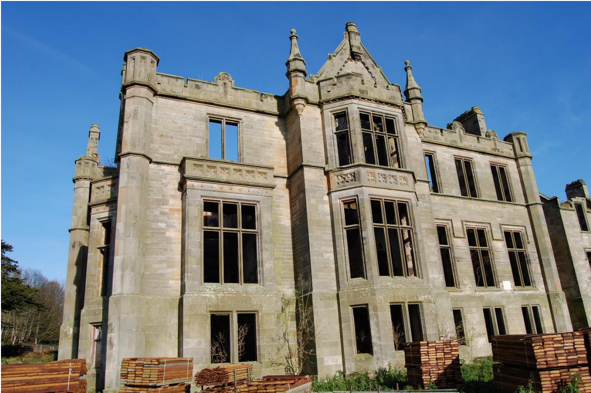
Illus 15 West end of south façade Phase 1 house; the lowest floor is the basement with ground, 1st and 2 nd (attic) above; facing N
