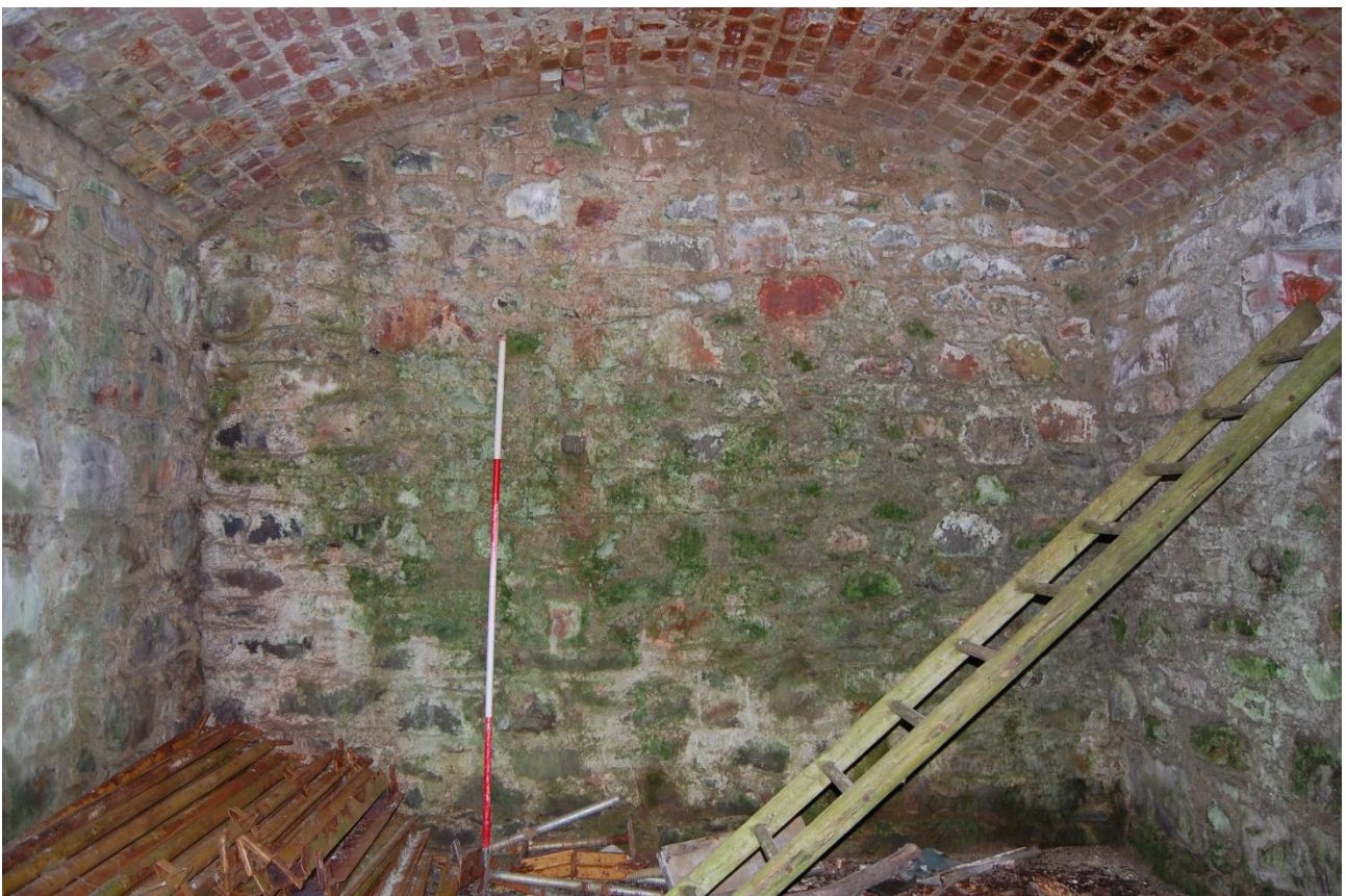
Illus 58 Detail of cellar brick-vaulted roof Room 66; facing W
