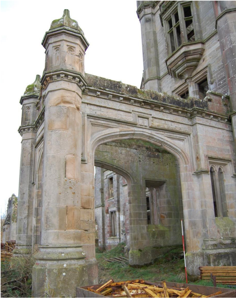
Illus 26 Room 20 Portico or carriage porch (D5; porte-cochere ) on north wall with initials AB above carriage door and ogee topped octagonal turrets (left); facing ESE
