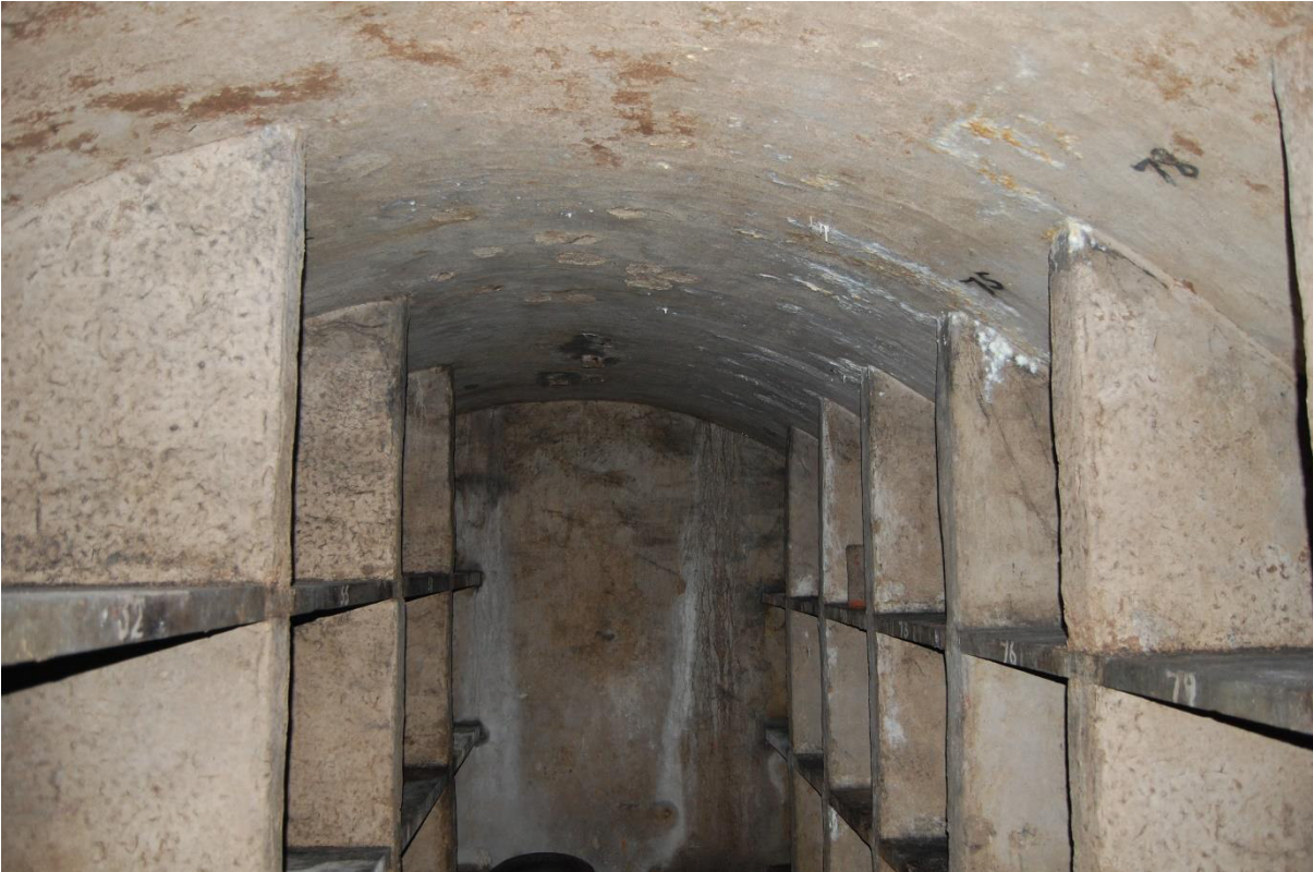
Illus 24 Room 10 showing stone shelves and brick uprights built into the brick-vaulted room
