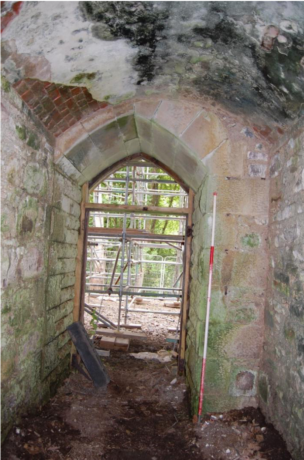
Illus 60 Room 67 internal façade D3; facing E
