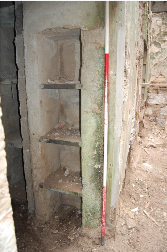
Illus 23 Door 49 entrance into Room 9 showing stone shelves within doorway on both W and E jambs; facing WNW
