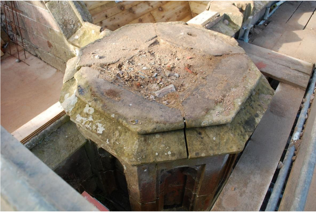
Illus 66 Top of F30 chimney; facing SW
