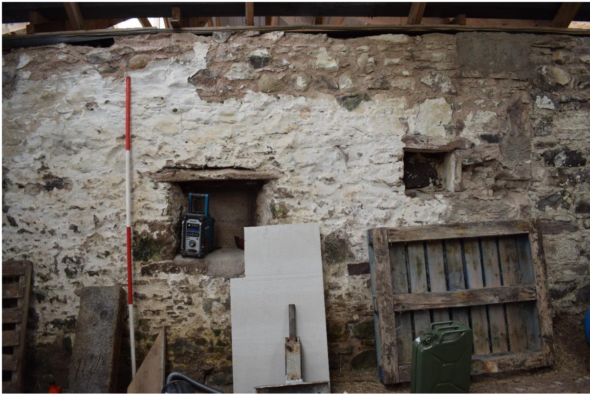
Illus 12 Room 5 SW interior wall W11 (left) W10 (right); facing SW
