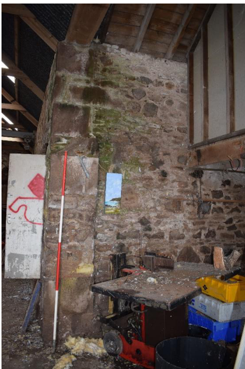
Illus 15 D31 (behind ranging rod) showing location of wall removed between Room 3 (left) and Room 2 (right); facing E
