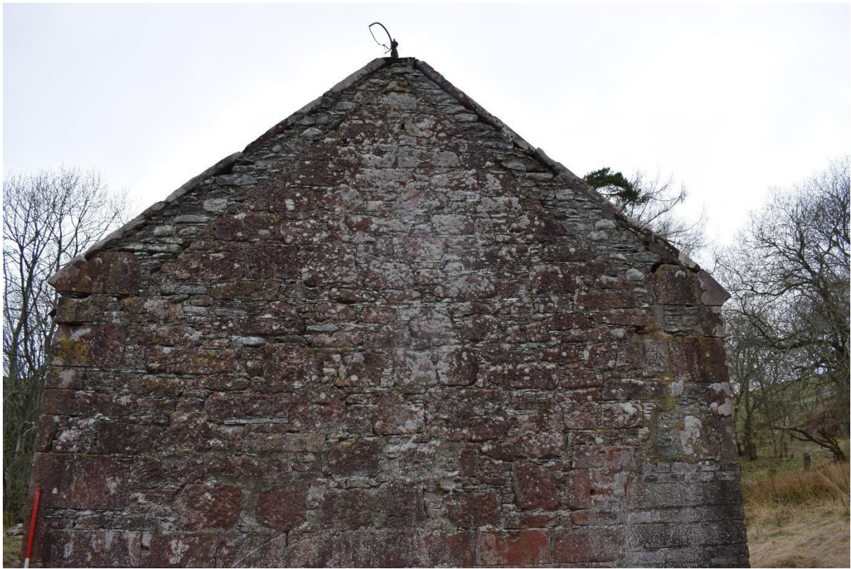
Illus 20 SE gable upper section showing grey sandstone scar under roofline where structure was attached for mill wheel; facing NW
