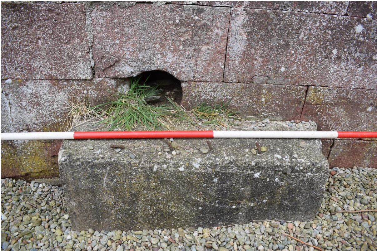
Illus 22 Concrete block possibly the outer headstock (F9) and circular axletree aperture (F8; above).
