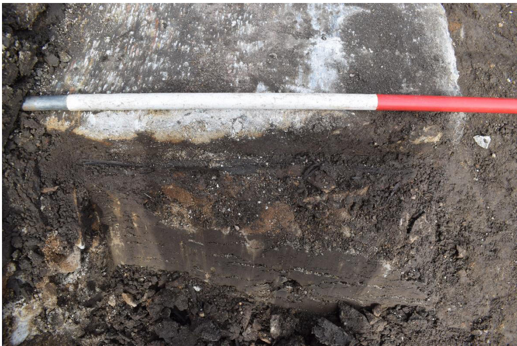
Illus 4 Wood shuttering in situ along the base of the concrete plinth (centre); facing WNW
