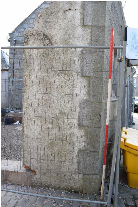
Illus 7 NW corner showing N wall cut down prior to this survey
