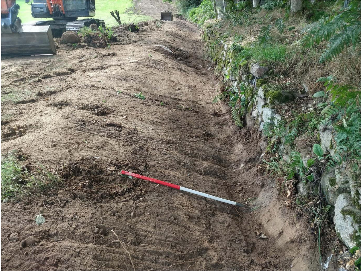
Illus 3 Section of ditch adjacent to ha-ha wall after clearing. Note varying levels of wall preservation in this particular section.
