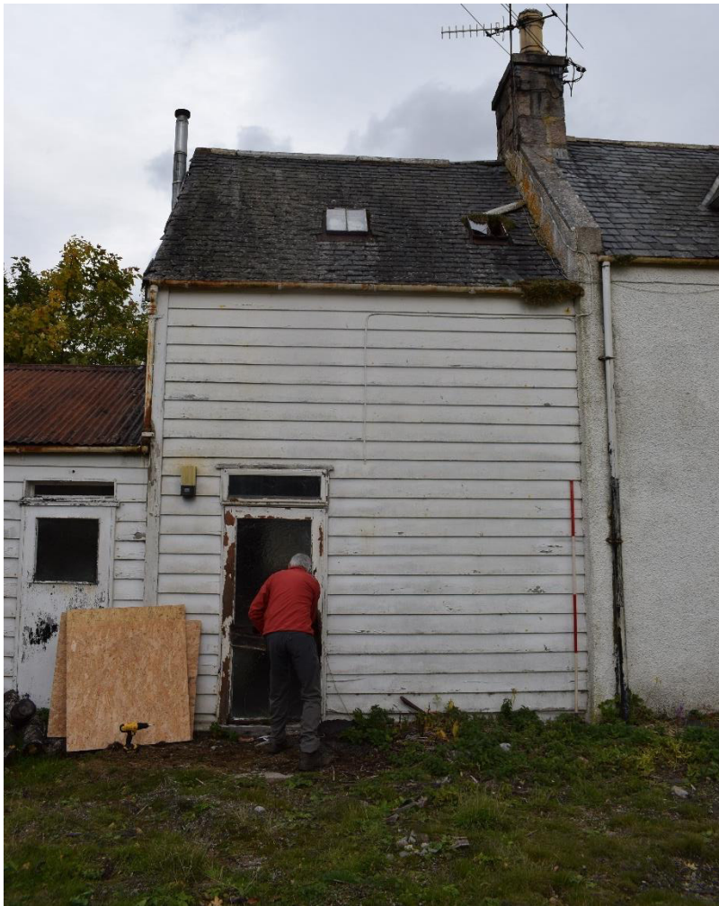
Illus 14 Phase 3 wood paneled S façade with D2 and grey slate roof; facing N
