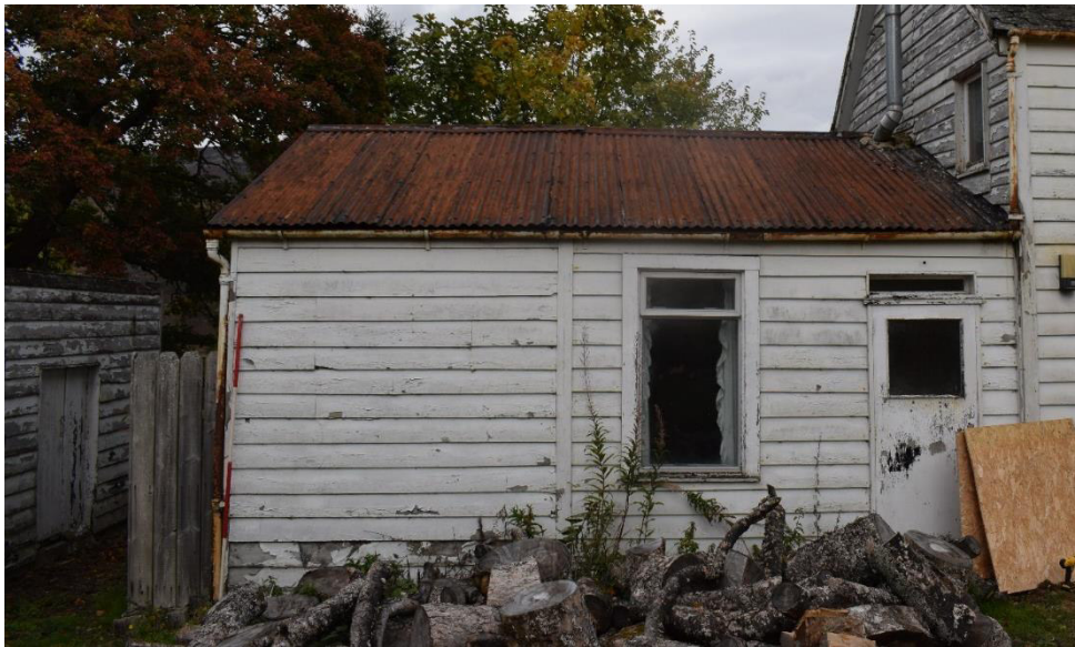
Illus 16 Phase 4 metal-roofed wood-panelled extension with W1 and D1; facing N
