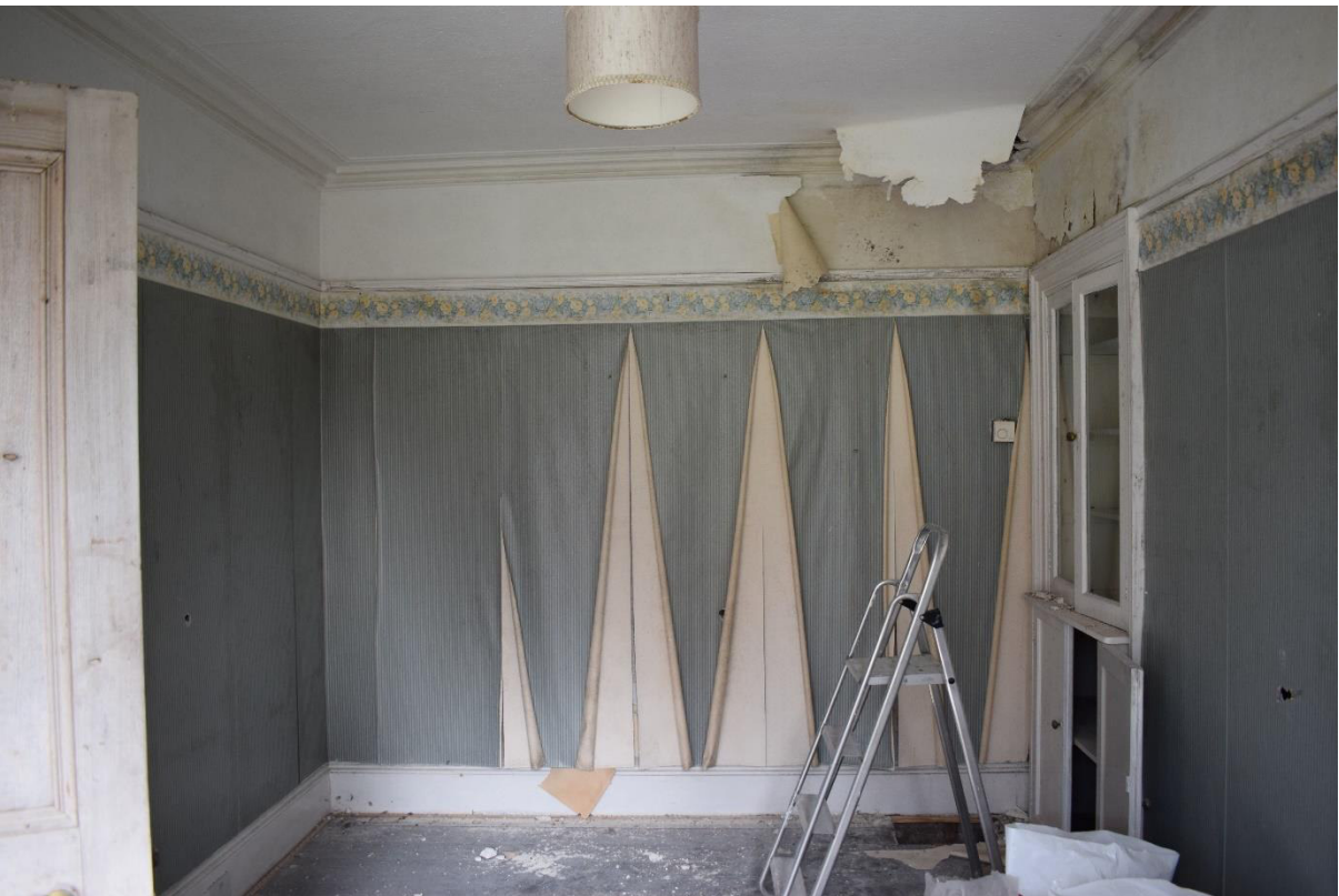
Illus 12 Room 2 N wall showing corning; facing N
