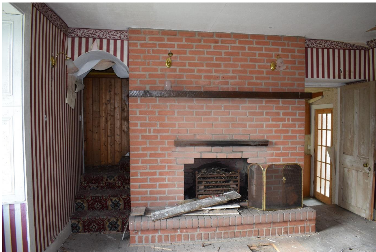
Illus 13 Room 5 W wall, originally the W wall of the phase 1 cottage, with 1970s (?) fireplace F10 and door to upstairs room (left); facing W
