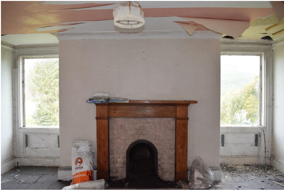
Illus 10 Room 1 N wall W7, fireplace F1, W8; facing N
