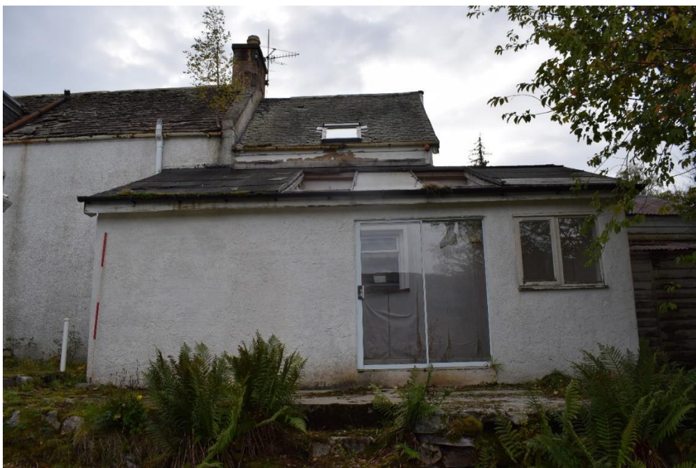
Illus 17 Room 11 N wall; facing S
