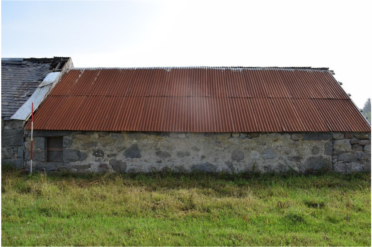
Illus 8 Phase 2 SW façade; facing NE
