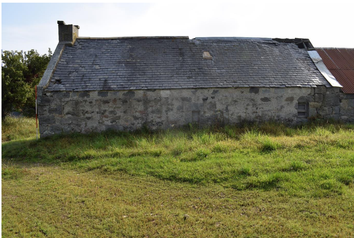
Illus 5 Phase 1 cottage SW façade; facing NE
