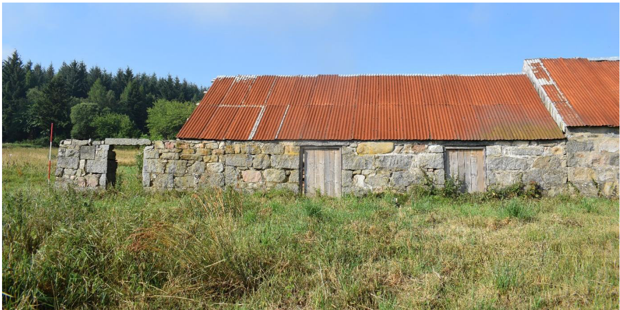
Illus 7 Phase 2 (right) and Phase 3 (left); facing SE
