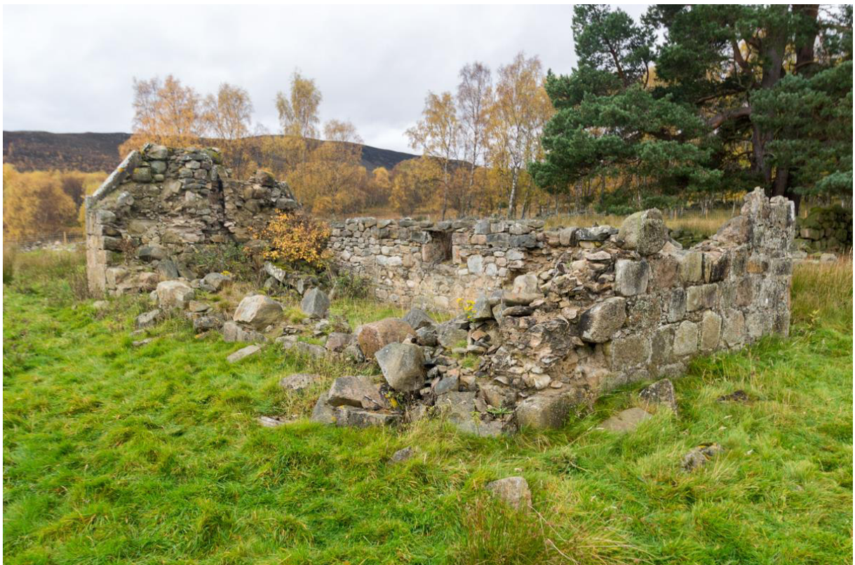
Illus 8: Longhouse A – view looking W. Note central window (W1) on NW facing wall and infilled double-wall construction visible in foreground corner.
