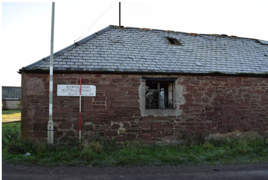
Illus 5 Building 1 Room 7A NW wall W1 (left blocked with red sandstone) and W2 inserted in Phase 3; facing SE
