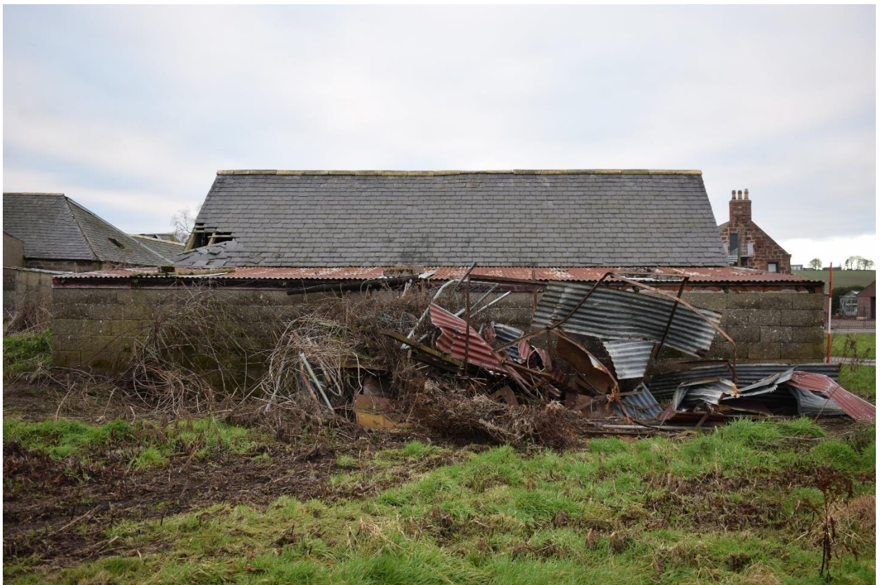
Illus 33 Building 4; facing NW
