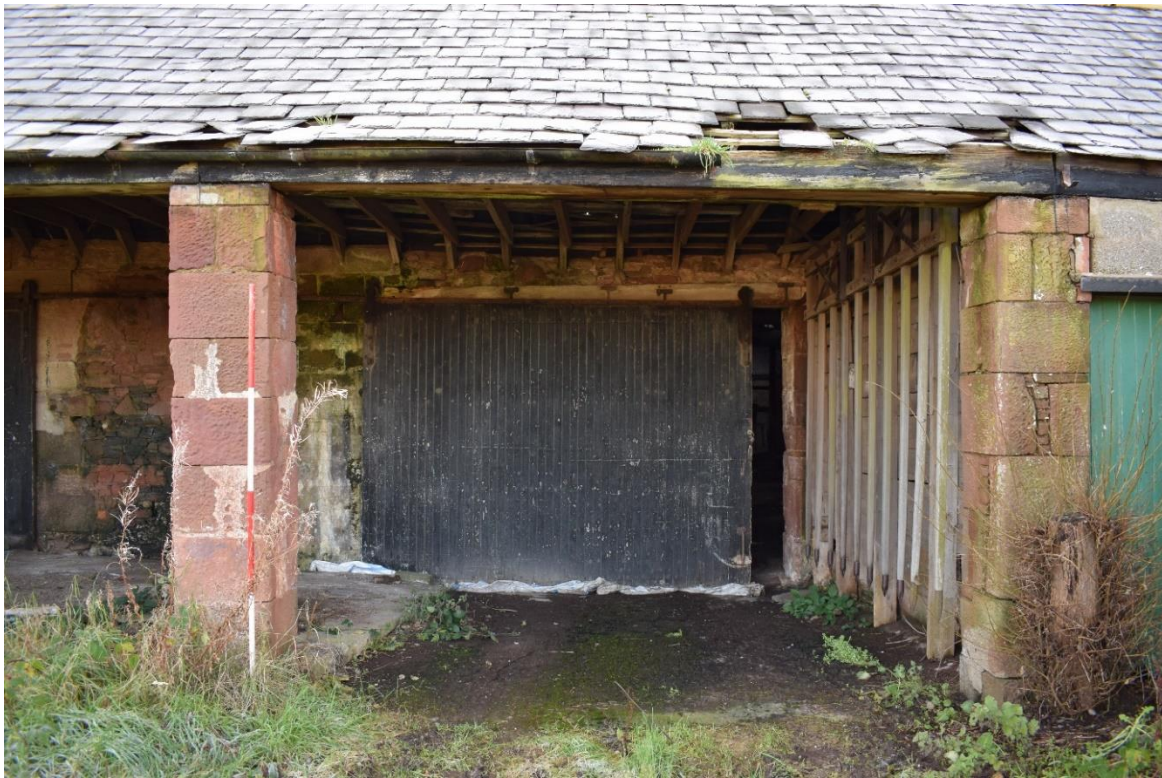
Illus 6 Building 1 Room 1 NE wall cart door D3; facing SW
