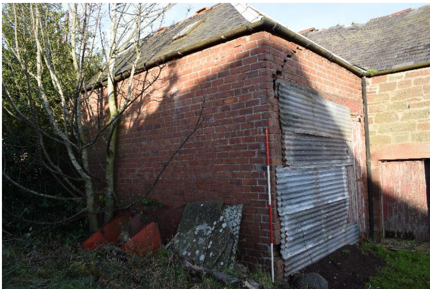
Illus 10 Building 1 Room 10 red brick extension; facing N
