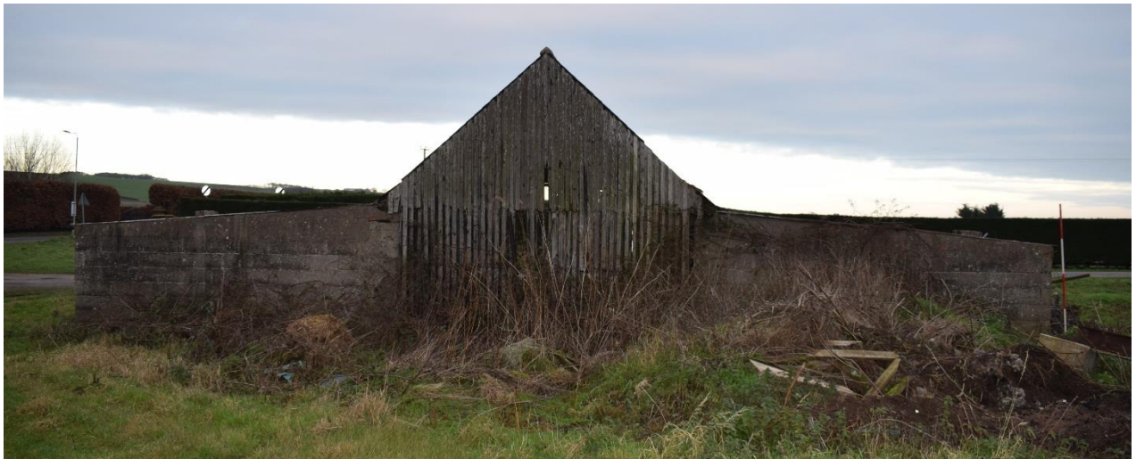
Illus 34 Building 4; facing NE
