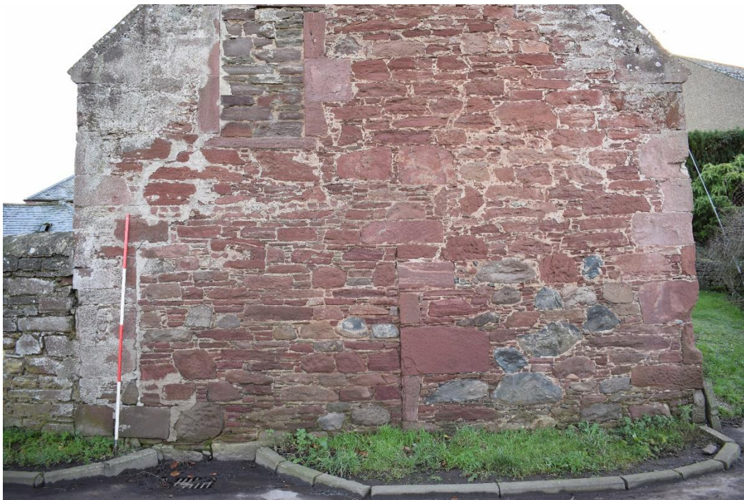
Illus 24 NNW gable lower section showing D41 (top left) with dated skewputt F3 (left) and blocked D42 (bottom); facing SSE
