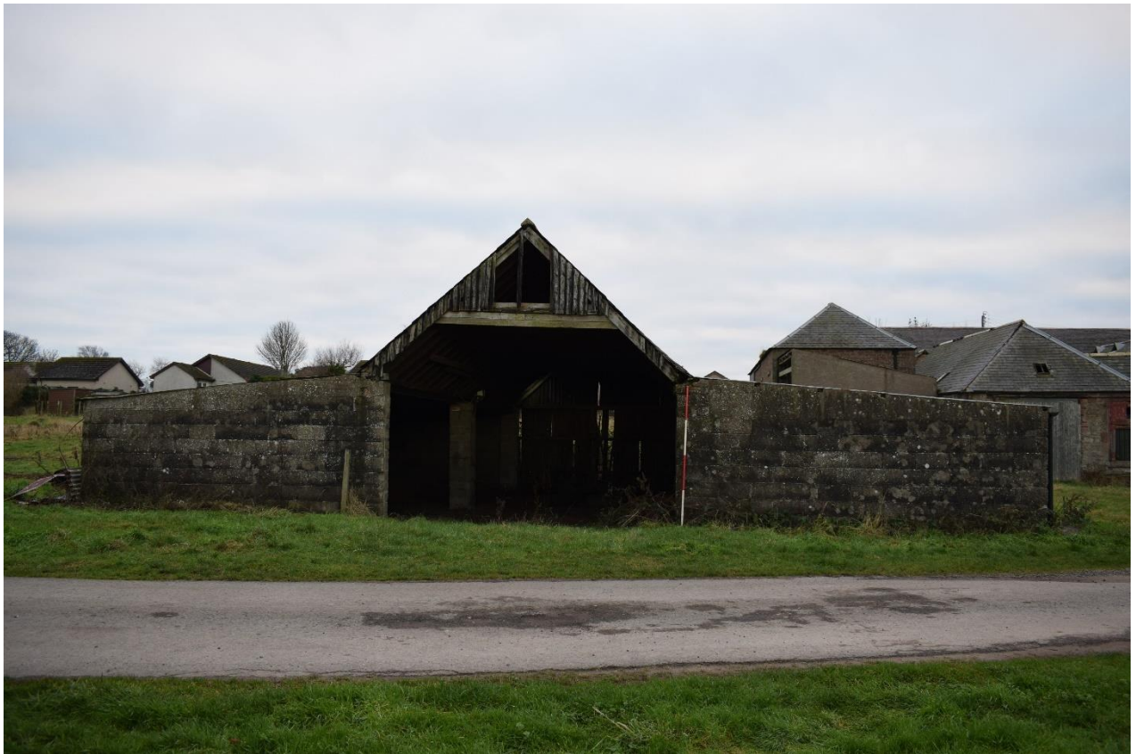
Illus 32 Building 4; facing SW
