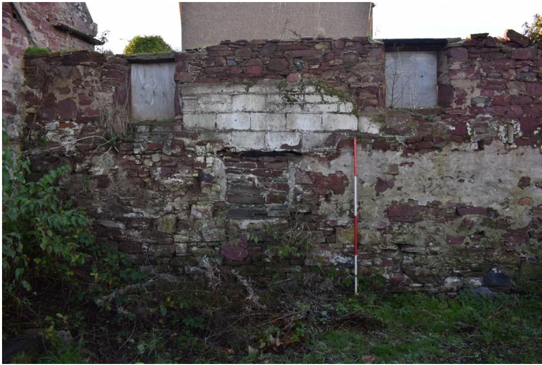
Illus 21 Building 2 WSW wall W14 and W16 (top) W15 below infilled with stone; facing WSW
