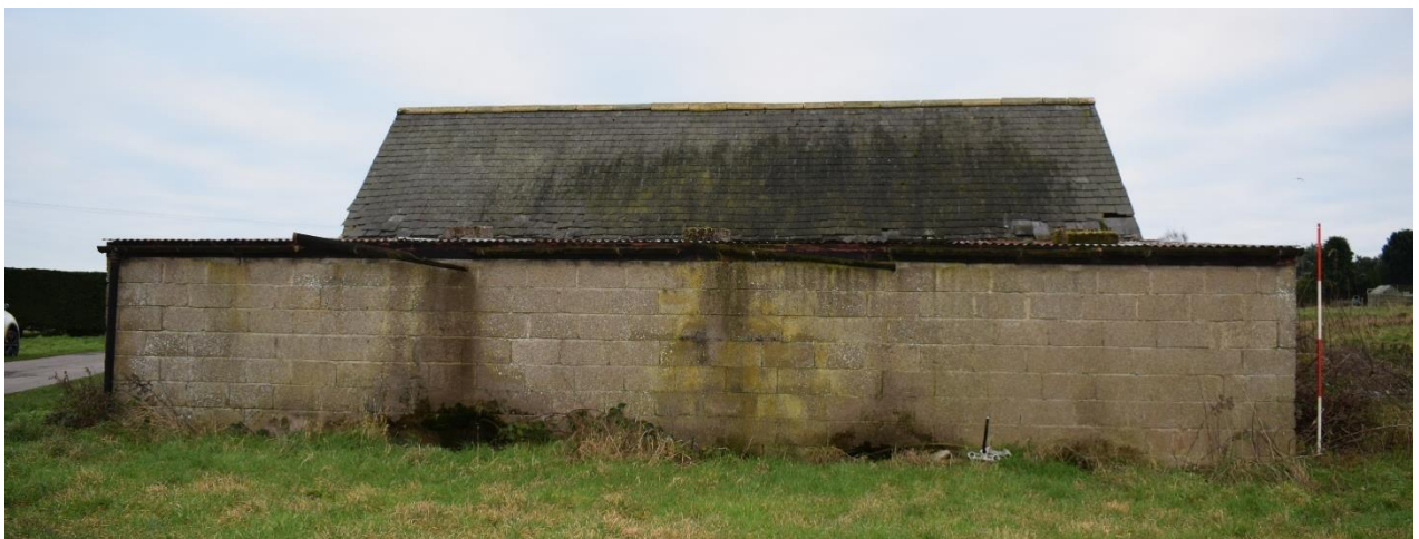
Illus 35 Building 4; facing SE
