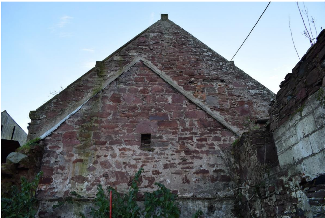
Illus 20 Building 2 gable (bottom) Building 2A gable (above); facing SSE
