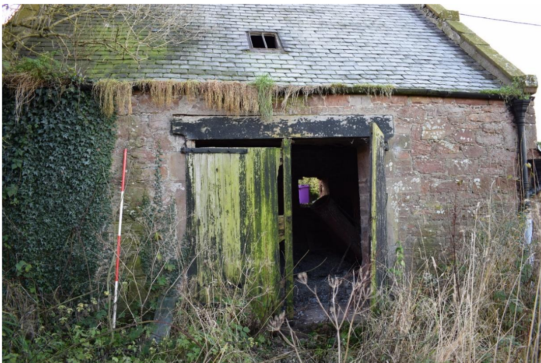
Illus 26 Building 2A ENE wall D43; facing WSW
