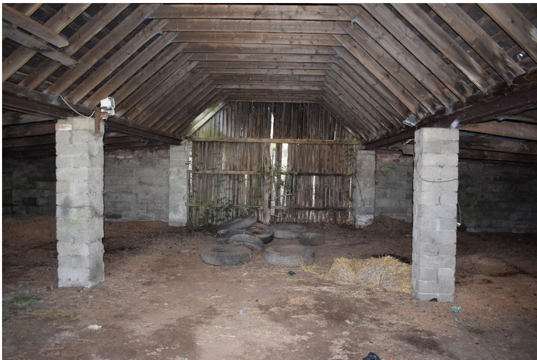
Illus 36 Building 4 interior; facing SW
