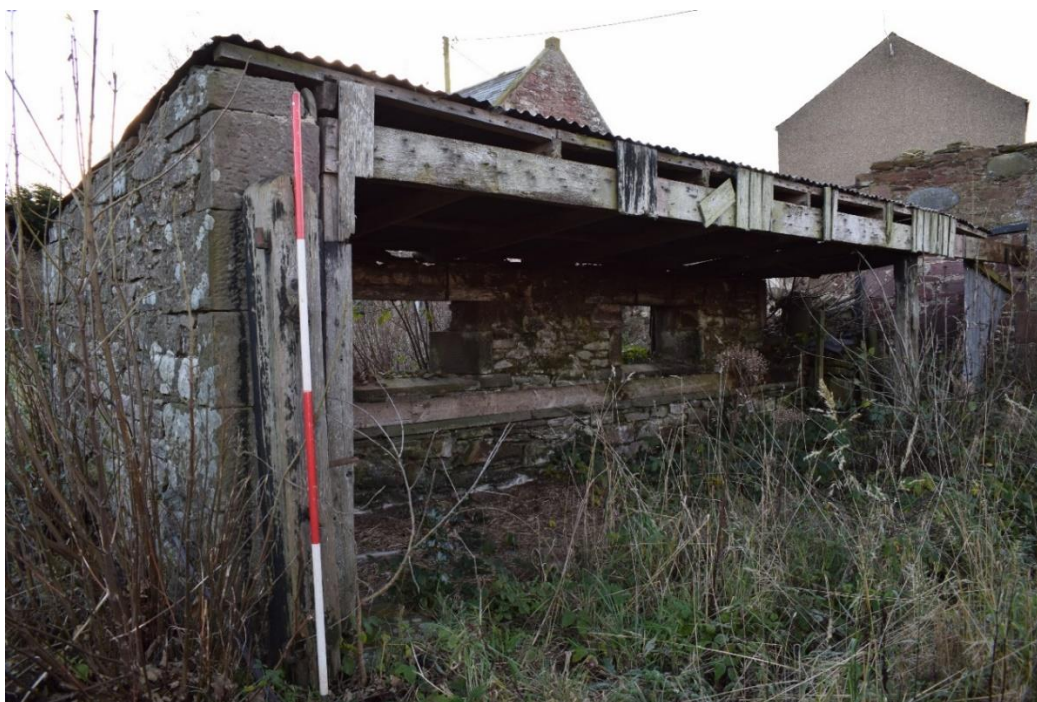
Illus 29 Building 3; facing S
