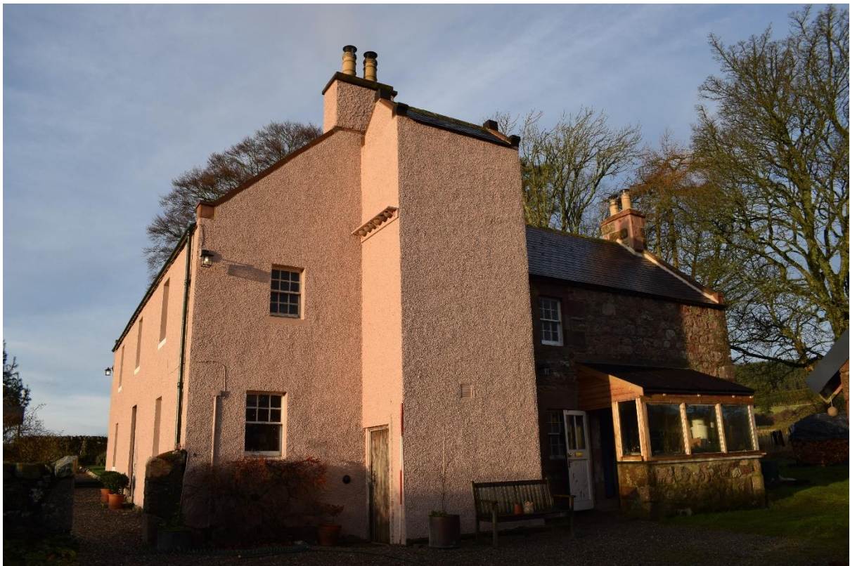
Illus 5 Building 1 E façade; there are internal alterations within the water tower (centre); facing W
