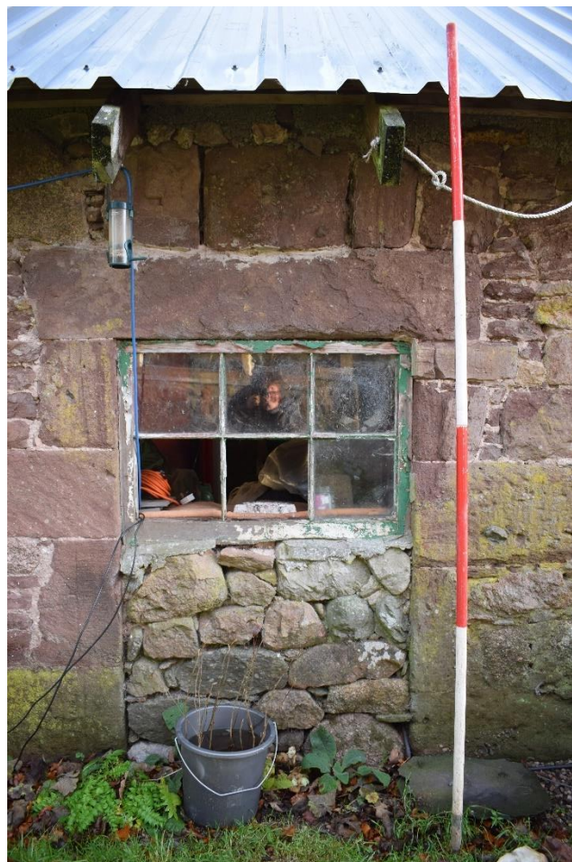
Illus 11 Building 2 Room 3 D7 converted to a window (W5); facing E
