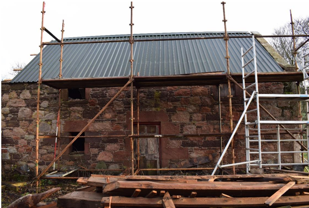
Illus 14 Room 8 W façade; facing E
