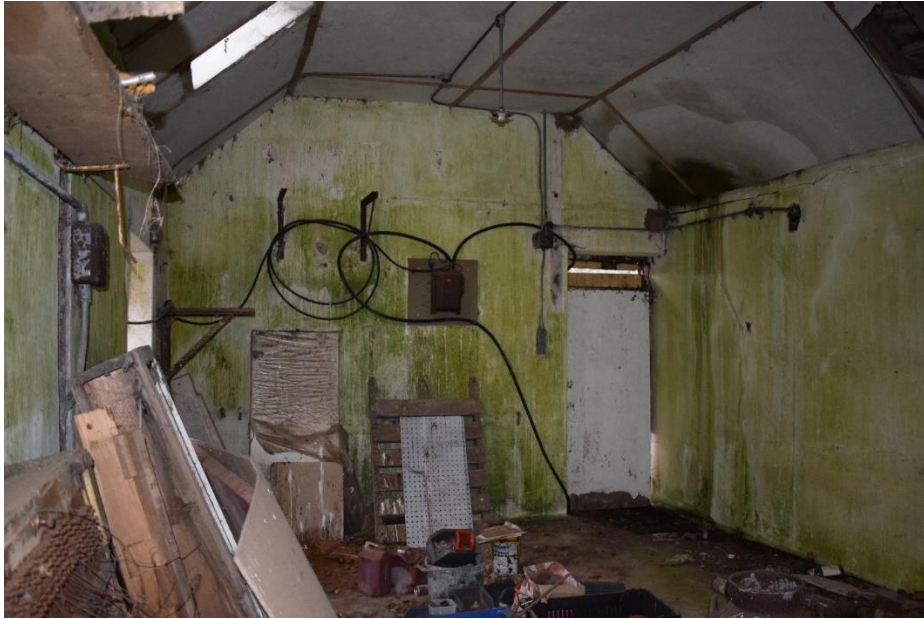
Illus 11 Building 2 interior; facing NNE
