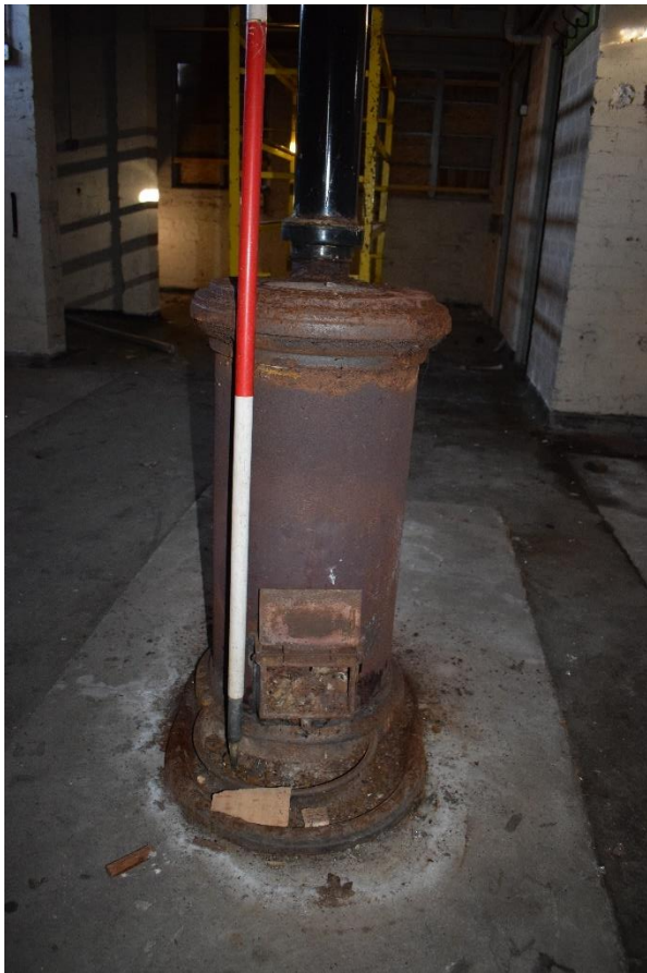
Illus 34 Building 6 stove F1 in centre of Room 6; facing N
