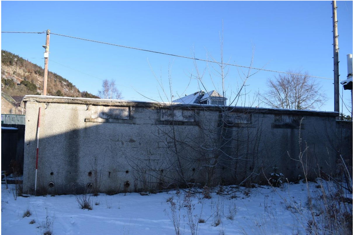
Illus 29 Building 5 S façade with windows W15-W18; facing N
