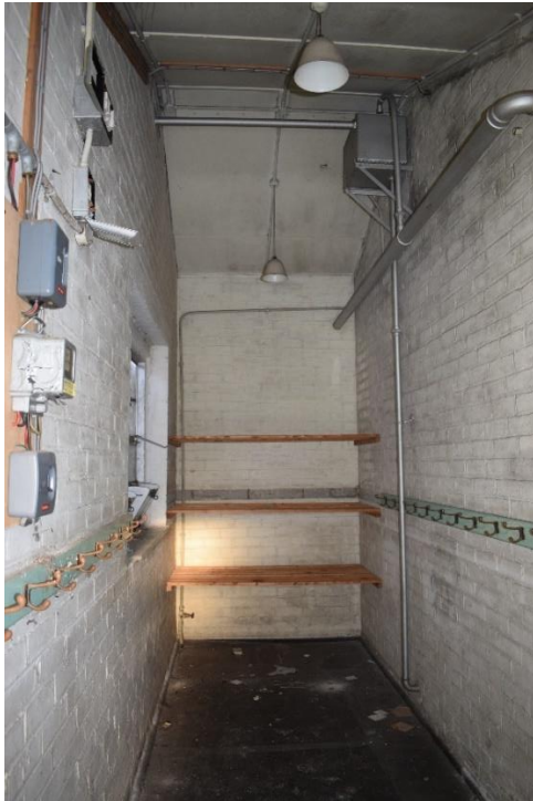
Illus 27 Room 3 showing brick construction; facing N
