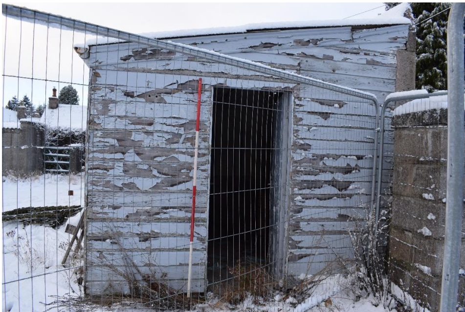
Illus 19 Building 2 E façade Room 3 with D1; facing W
