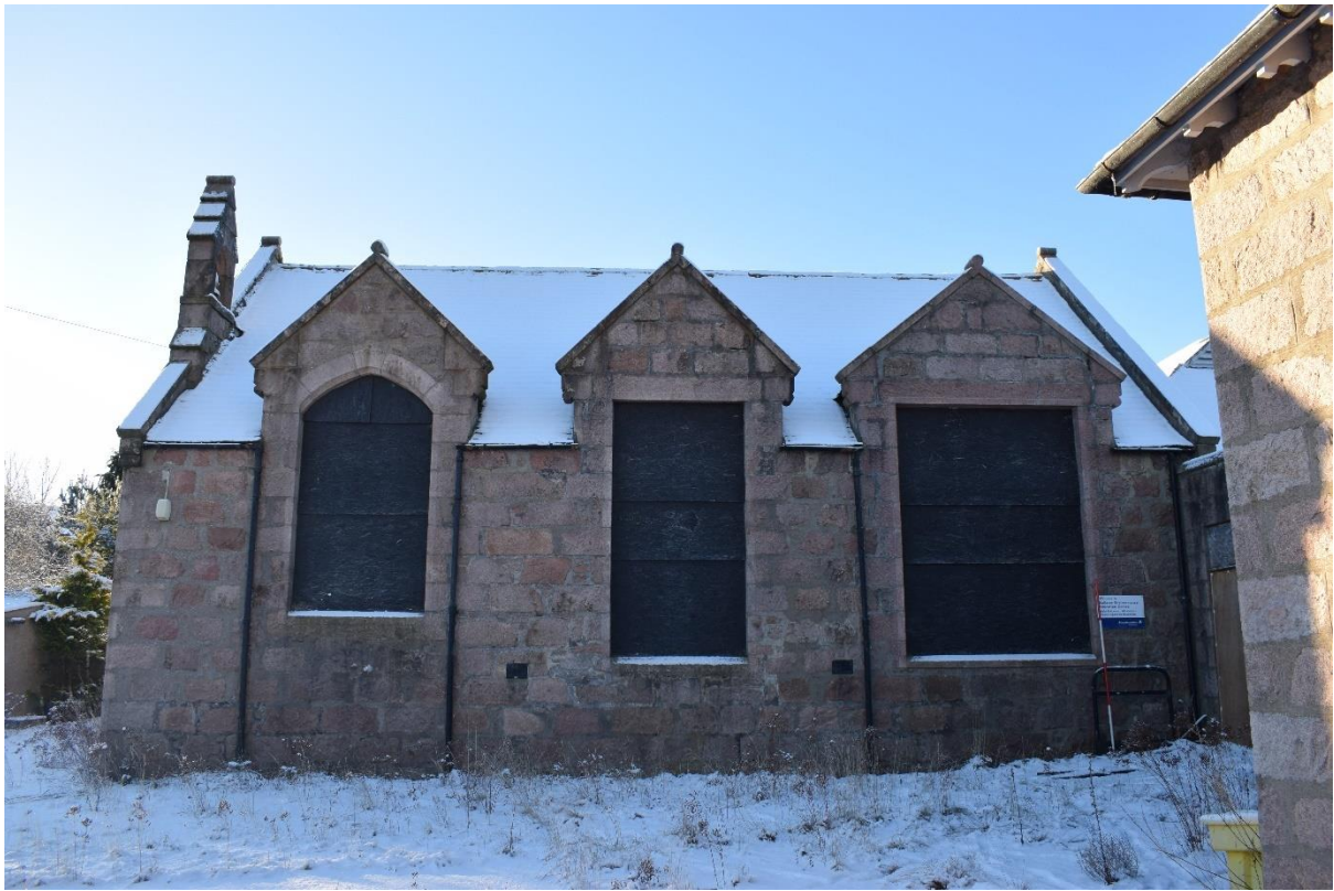
Illus 6 Rooms 2 and 3 male dormitory N wall windows W44, 45, 46; facing S
