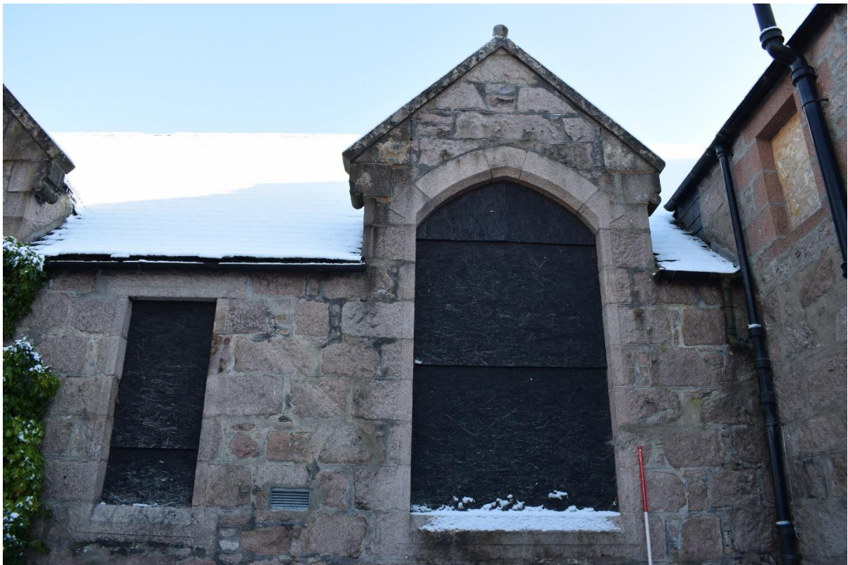
Illus 13 Room 7 W façade windows W53 (left) W50 (right); facing E
