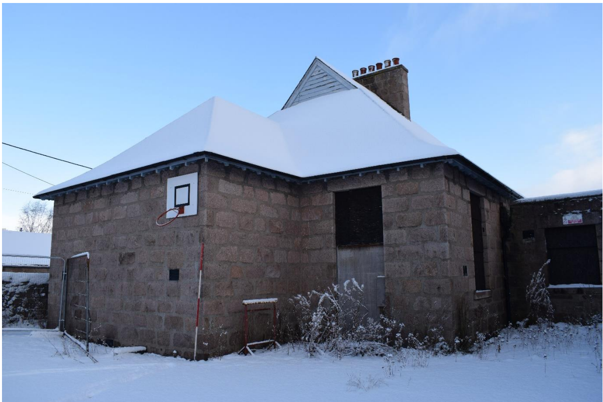
Illus 15 Phase 2 pavilion Room 10 with link corridor (right); facing NE
