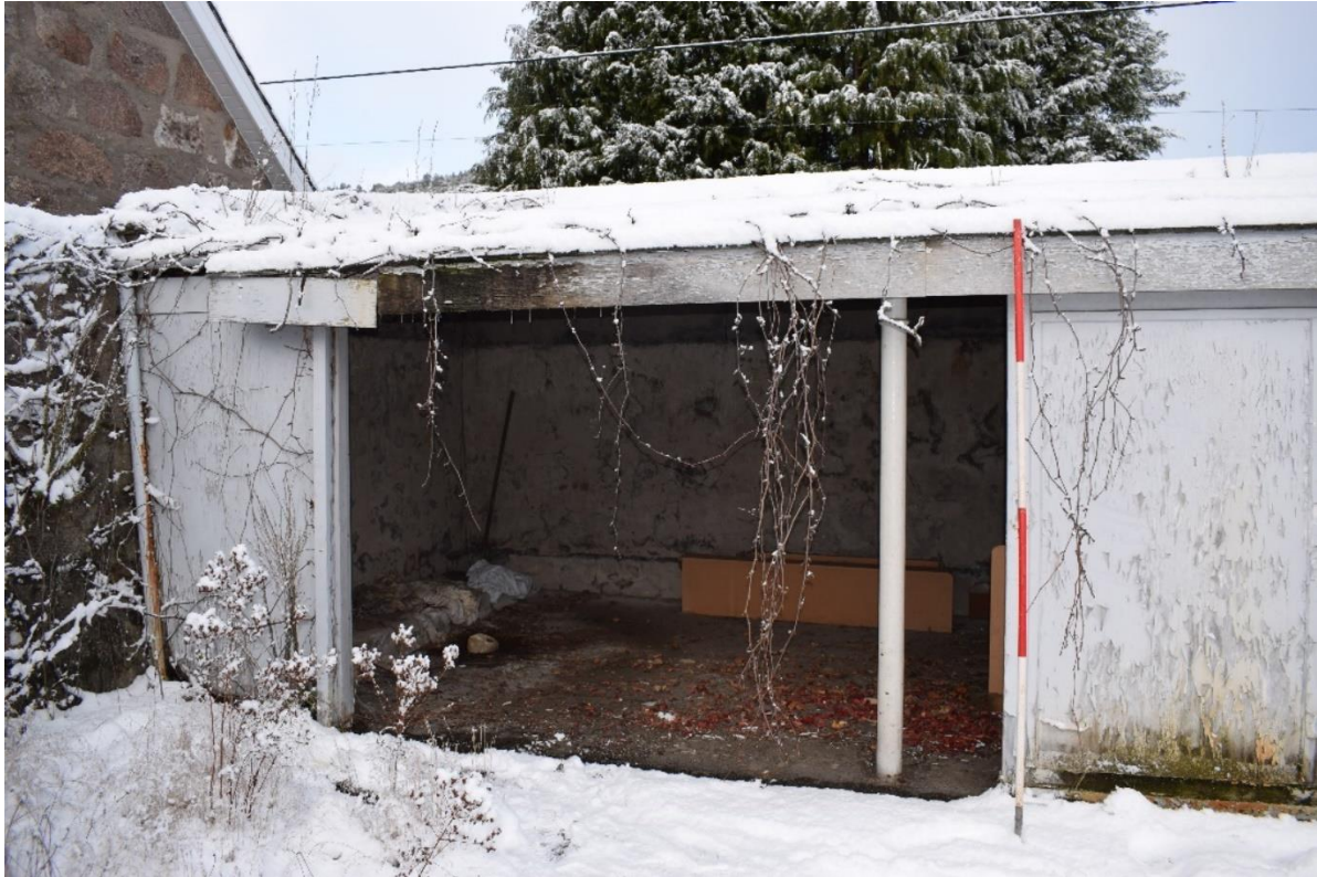
Illus 18 Building 2 S façade Room 1 with cast iron pillars; facing N
