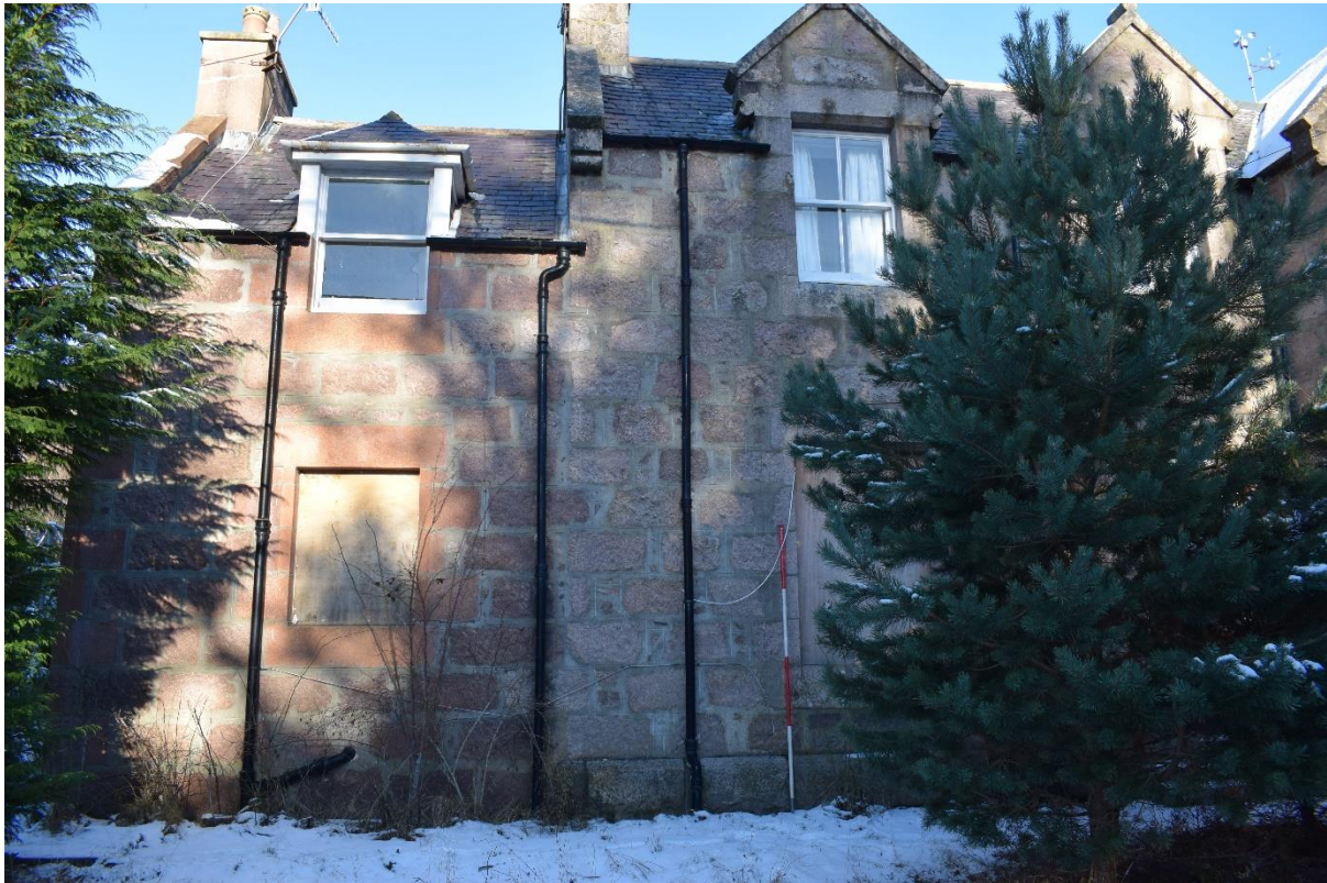
Illus 41 Front S façade Building 9 showing Phase 2 extension (left); facing N
