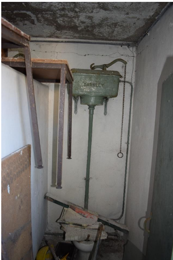
Illus 30 Building 5 toilet cubicle Darnley cistern; facing S
