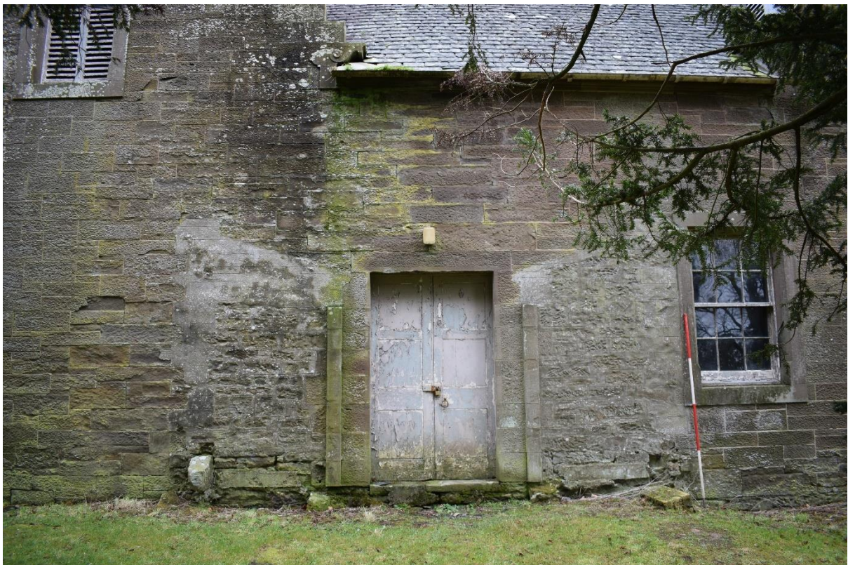
Illus 15 Stables SSE façade D1 with scars F24A (right) and F24B (left) where small extensions seen on OS maps have been removed; facing NNW
