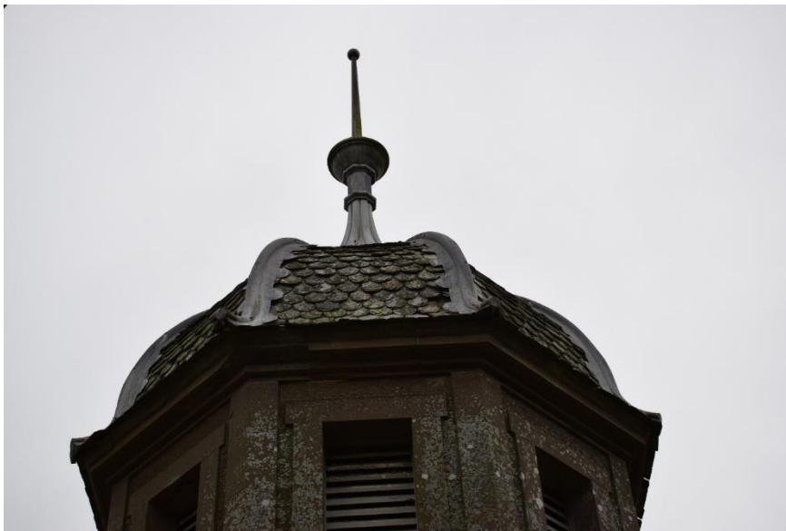
Illus 44 Detail of fish-scale slated ogee roof with ball and spike finial on roof of Room 43; facing NW
