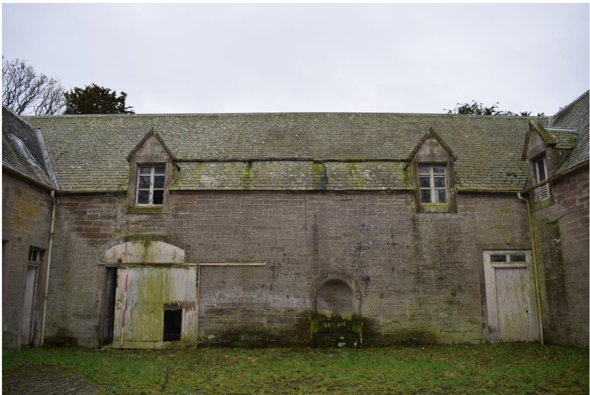
Illus 19 Stables inner courtyard SSE façade; facing SSE
