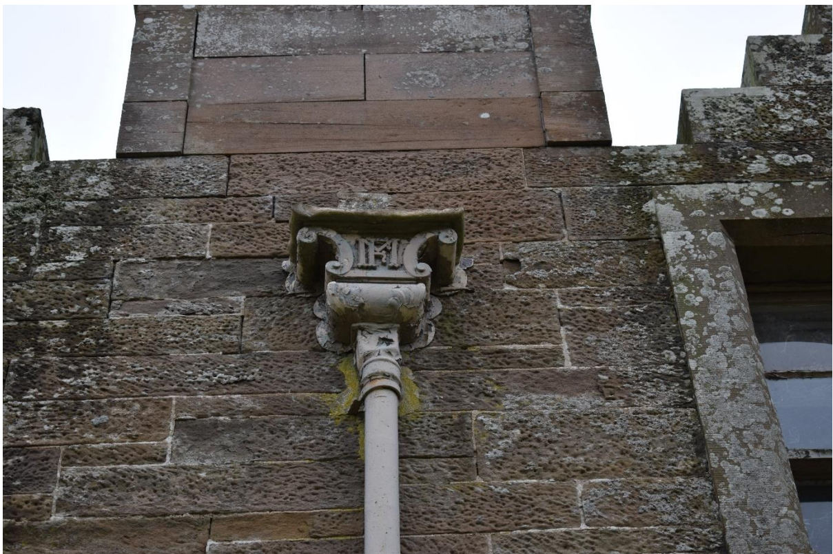
Illus 17 Stables WSW elevation Room 26 with cast iron rainwater hopper inscribed 'FM' presumably for Fox Maule Ramsay, the 2nd Baron of Panmure who revamped the buildings in the 1850s; facing ENE
