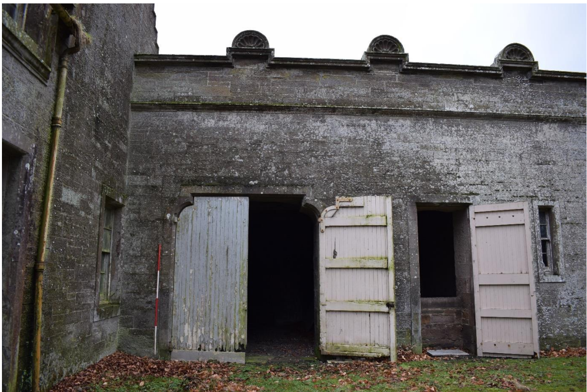
Illus 40 N building doors D5 and D6 with a string course above and a corniced crenellated parapet with segmental pediments; facing WSW
