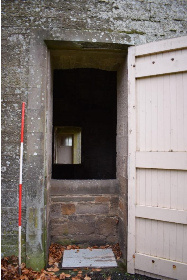
Illus 41 D6 with low wall inserted across opening to form window; facing WSW
