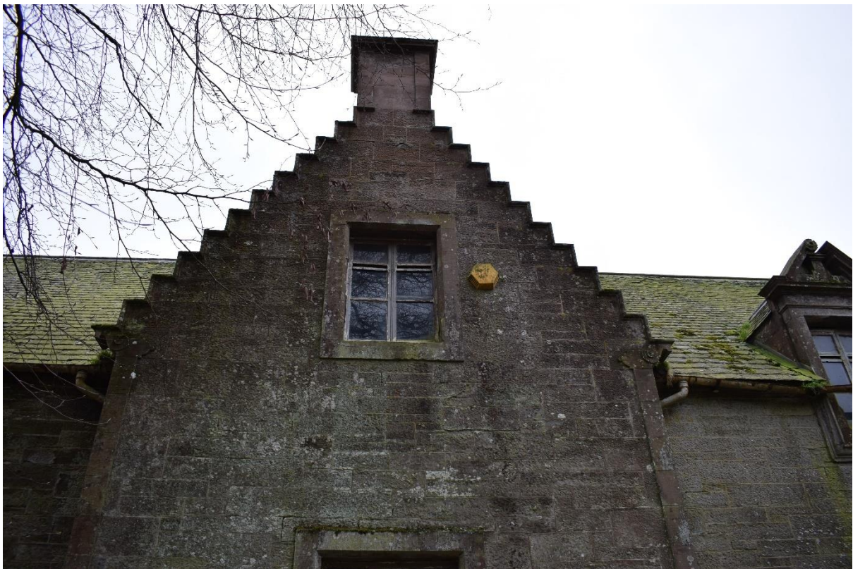
Illus 9 Stable block NNW elevation crow-step gable above W10; facing SSE
