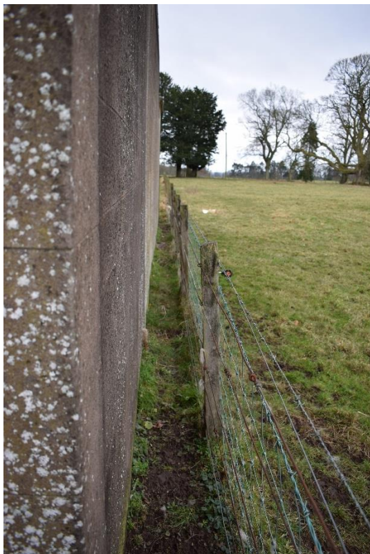
Illus 52 WSW wall Room 1 rendered after the demolition of Panmure House in 1955 (note there is no access to this side of the house); facing SSE
