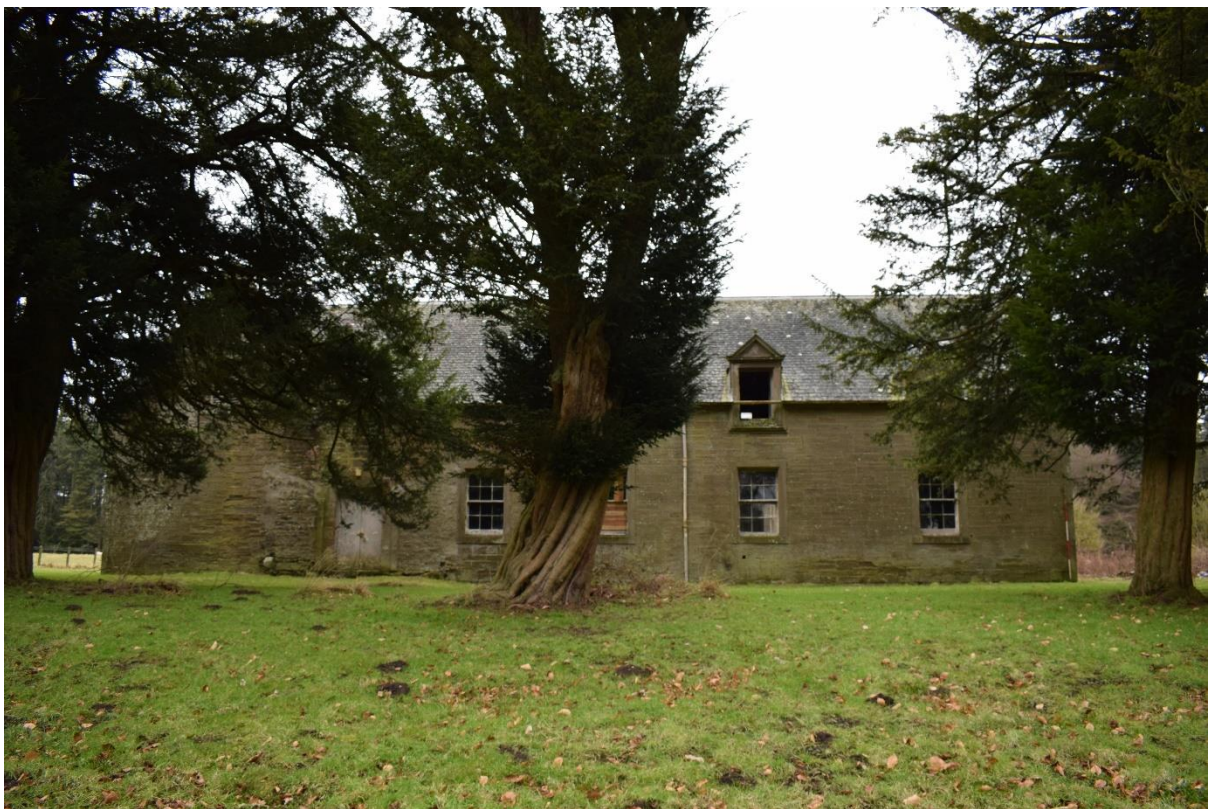
Illus 13 Stables SSE façade; facing NNW
