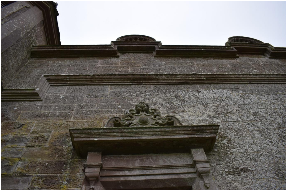
Illus 39 Room 1 NNW wall with pink sandstone portico above W18 and crenellations; facing SSE
