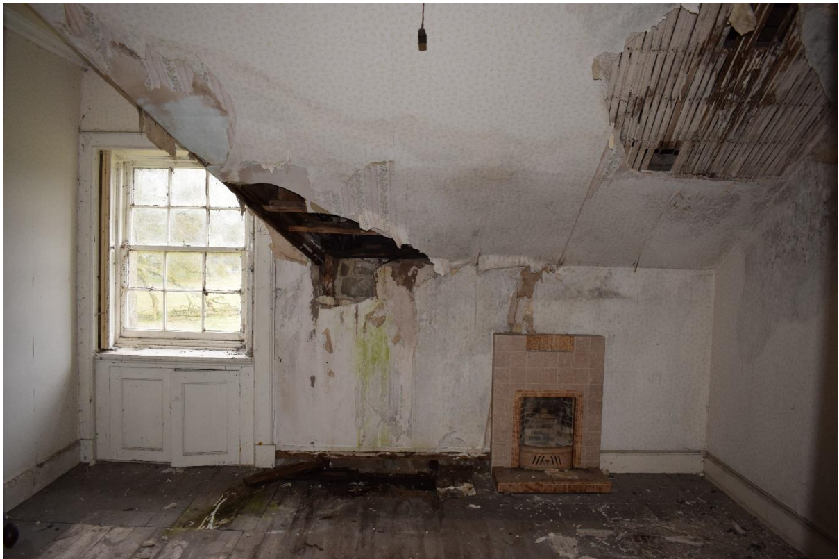
Illus 23 Room 38 WSW wall W32 (left) fireplace F26 (right); facing WSW
