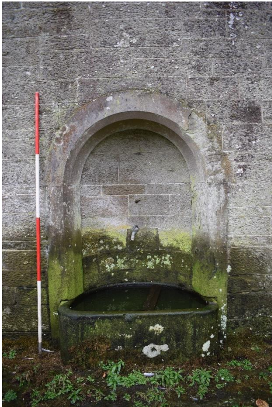
Illus 20 Sandstone and cast iron water trough F1; facing SSE
