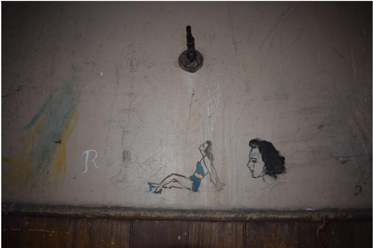
Illus 28 Room 16 NNW wall 1940s graffiti; facing NNW
