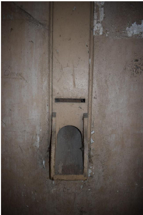
Illus 27 Room 15 cast iron chute F18; facing SSE
