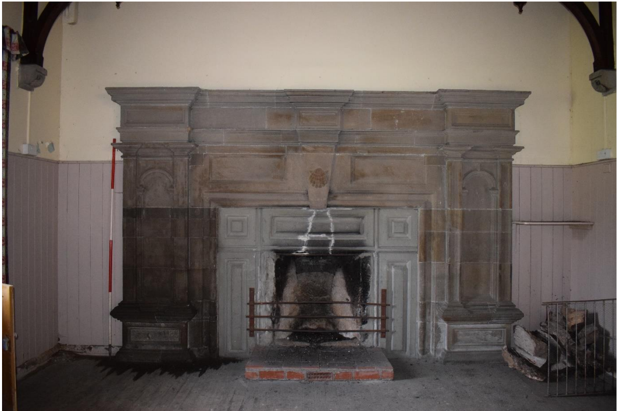
Illus 47 Room 1 fireplace F30 with central scallop motif showing timber hammerbeam roof and stone corbels; facing E
