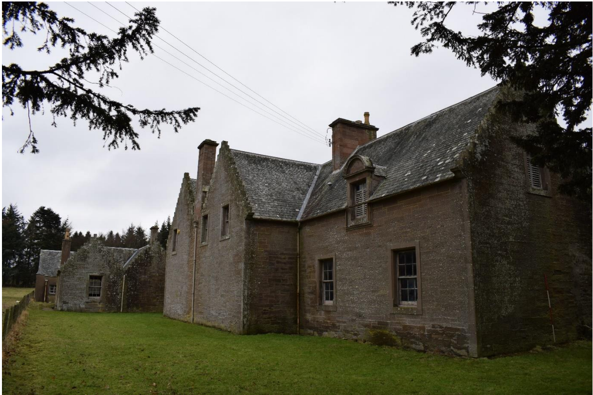
Illus 16 Stables WSW elevations with wider Room 26; facing NE
