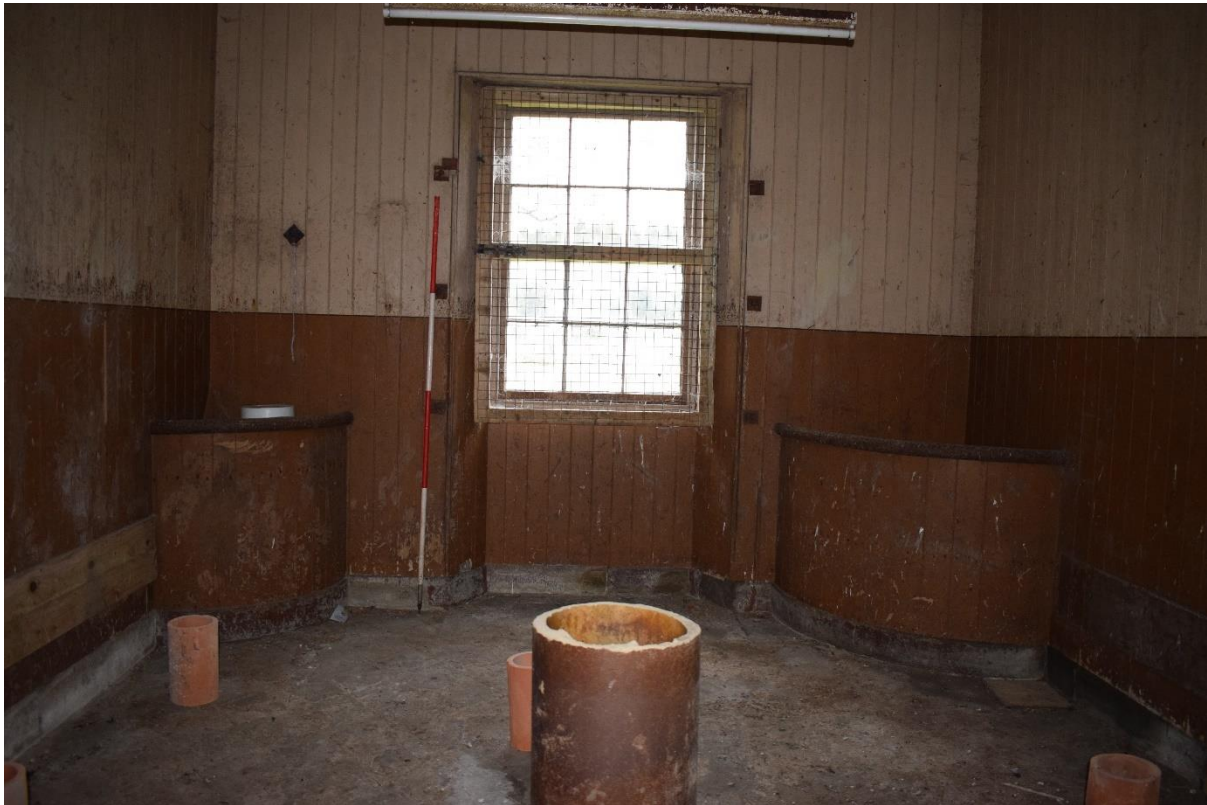
Illus 34 Room 24 stables WSW wall with W36 (centre) and wood and cast iron feed tubs F2 (left) and F3 (right); facing WSW
