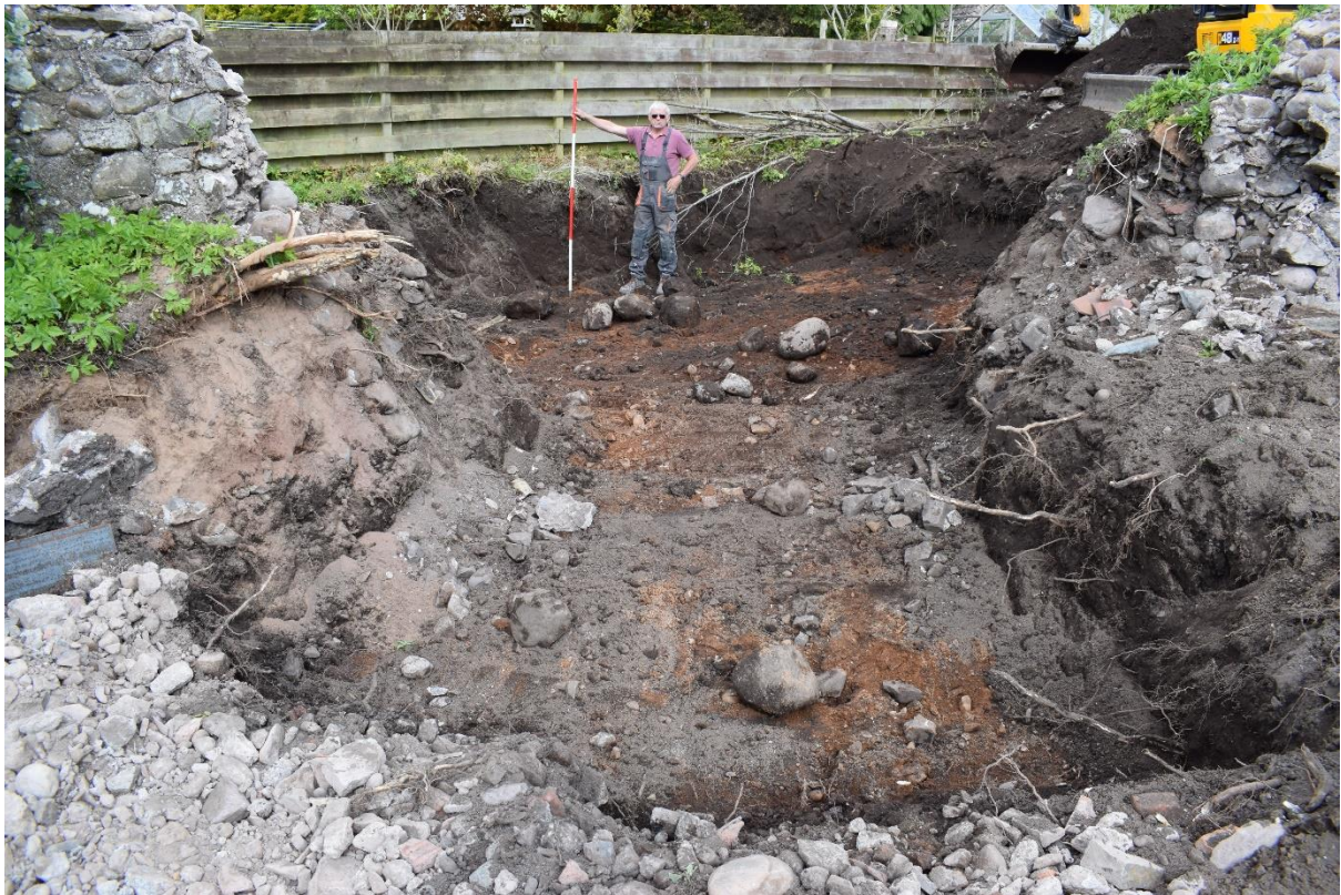
Illus 6 Up to 1.2m topsoil at the W edge of the site; facing W
