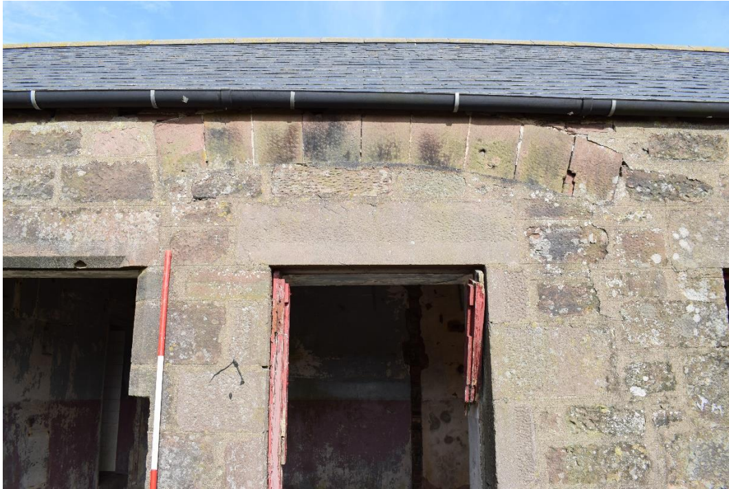
Illus 10 Room 7 SE wall D14 arched lintel detail; facing NW
