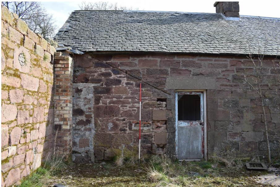
Illus 8 Room 6 SW wall D8 showing roof raggle F9; facing NE
