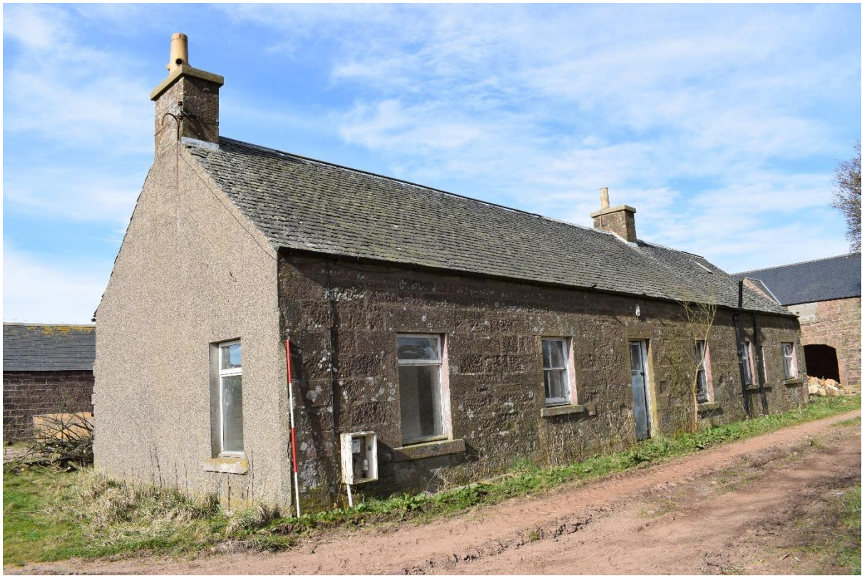
Illus 5 Farmhouse NE façade Rooms 1-6; facing W
