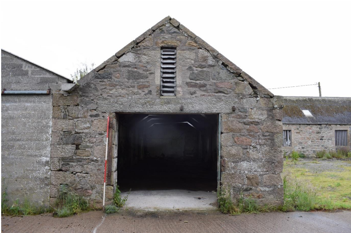
Illus 11 Building 4 W wing SSW wall D18; facing NNE
