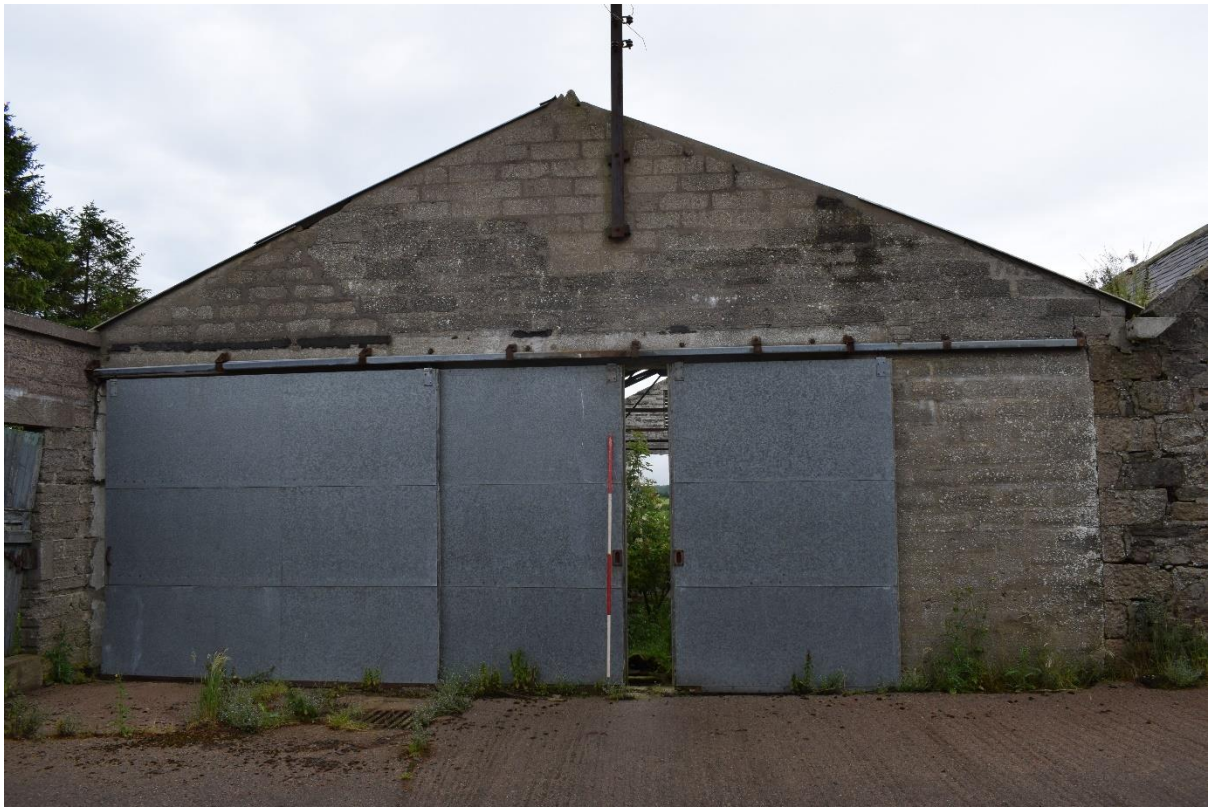
Illus 21 Building 5 SSW wall; facing NNE
