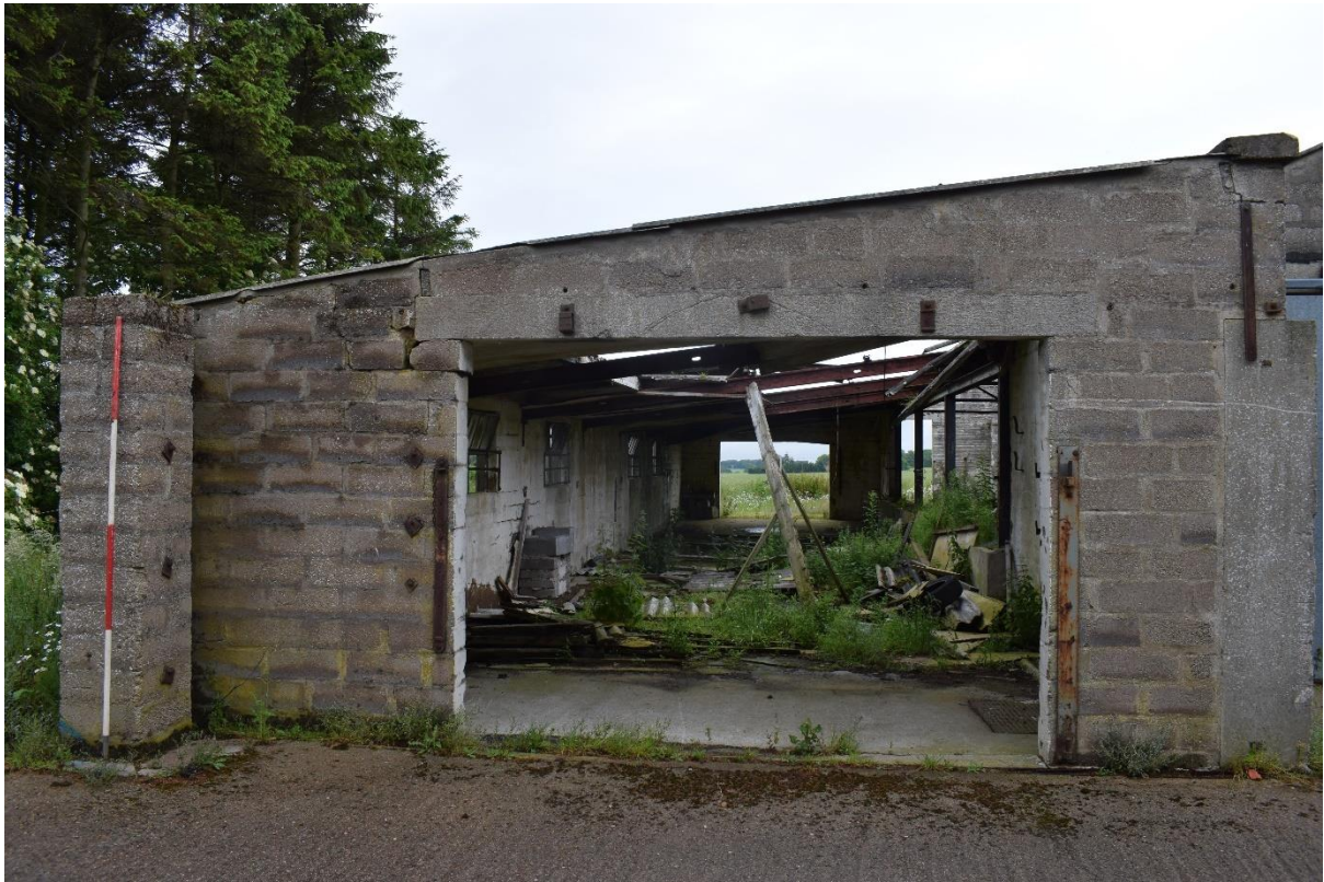
Illus 23 Building 6 SSW wall; facing NNE
