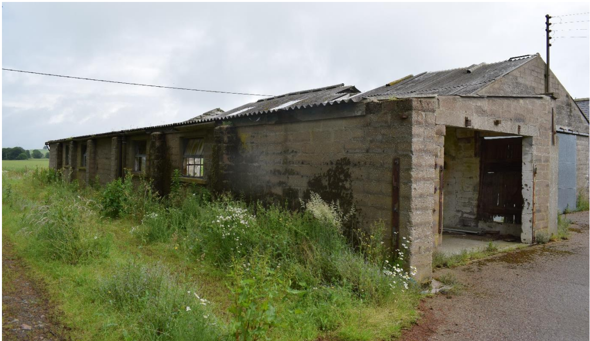
Illus 24 Building 6 WNW wall; facing NE
