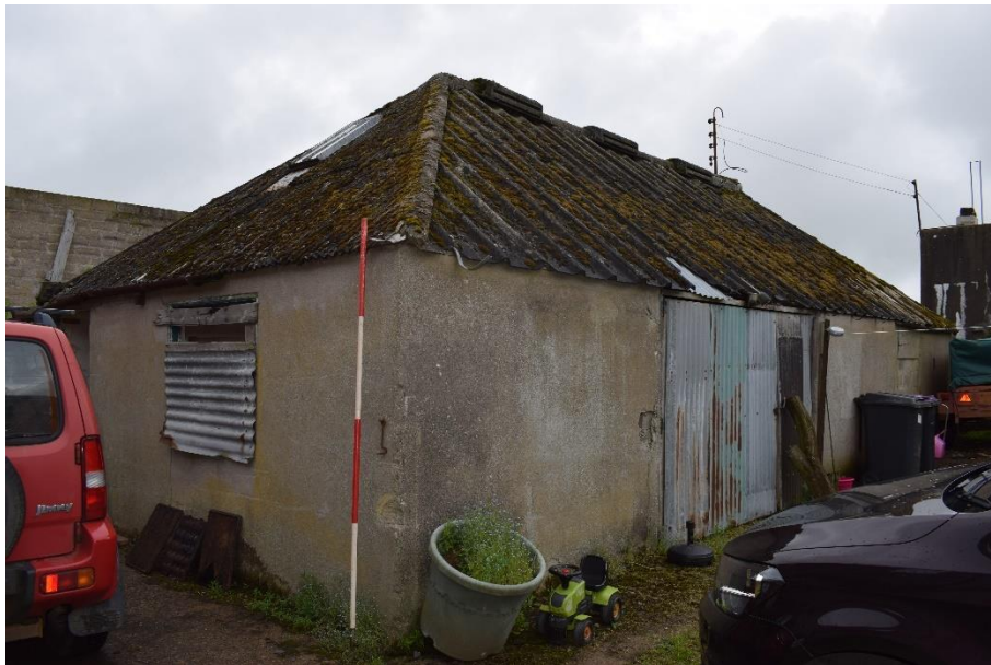
Illus 8 Building 3; facing NE
