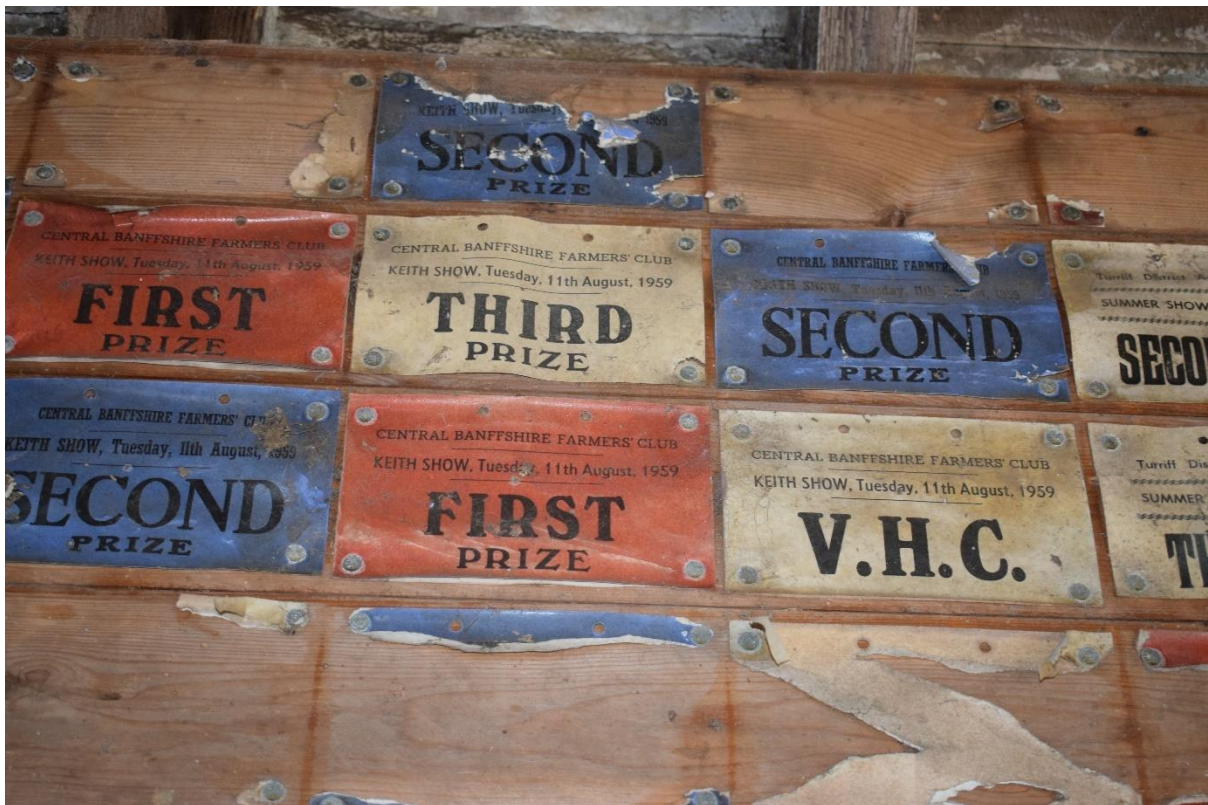
Illus 19 Building 4 E wing interior ESE wall detail of wooden board with show certificates F2
