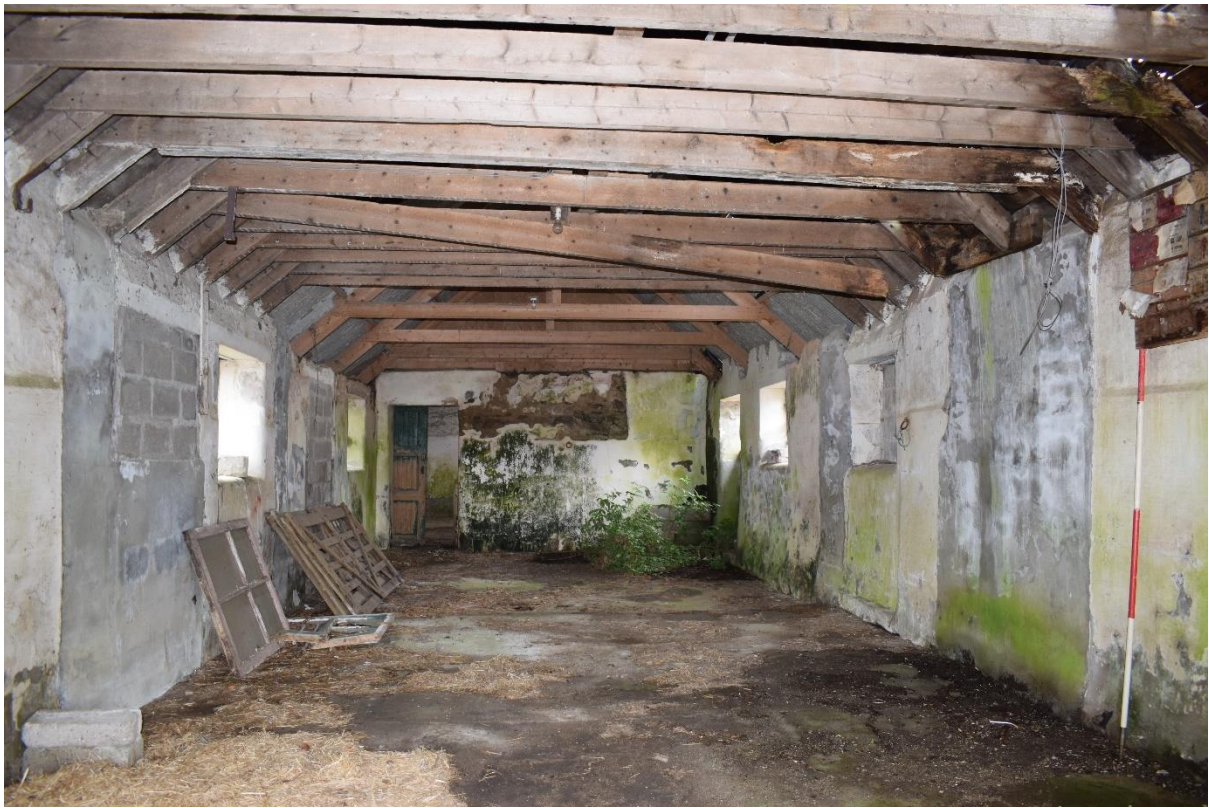
Illus 17 Building 4 E wing interior towards gable with D10; facing NNE
