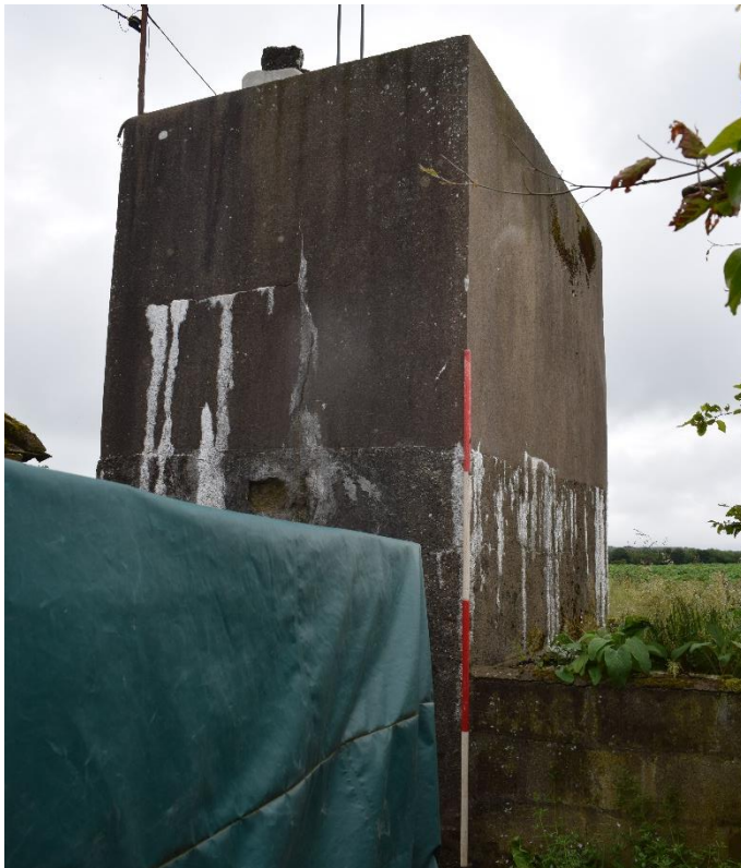
Illus 26 Building 7; facing NE
