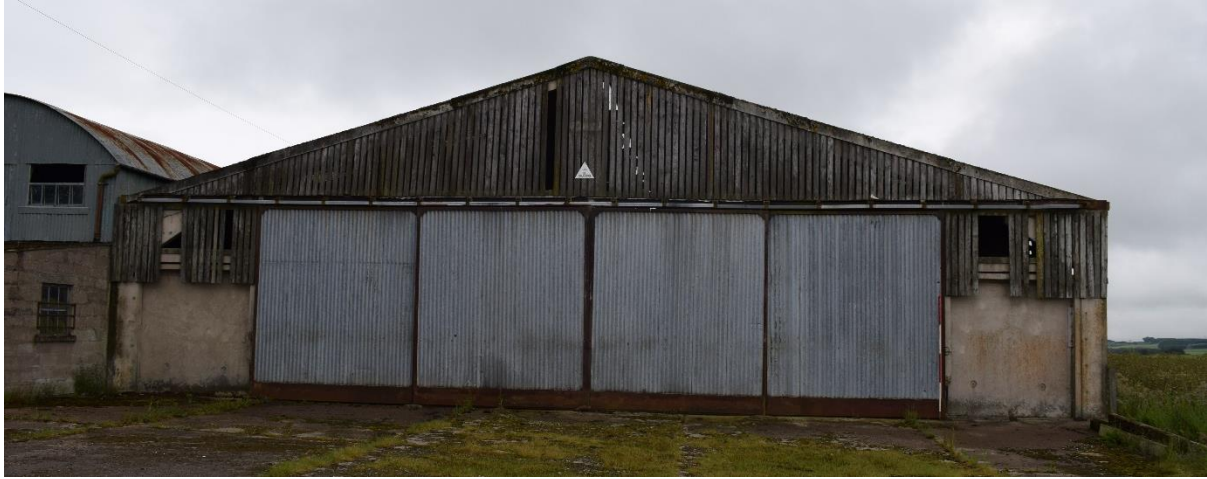
Illus 7 Building 2 WNW wall D24; facing ESE
