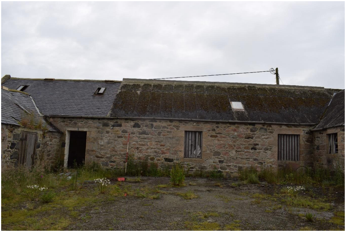
Illus 13 Building 4 N wing SSW wall D12, W5, D11; facing NNE
