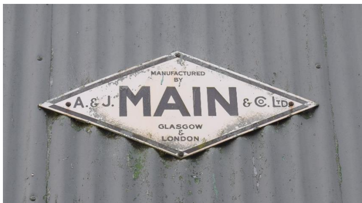
Illus 6 Building 1 constructed by A&J Main & Co Ltd, Glasgow and London; facing SSW
