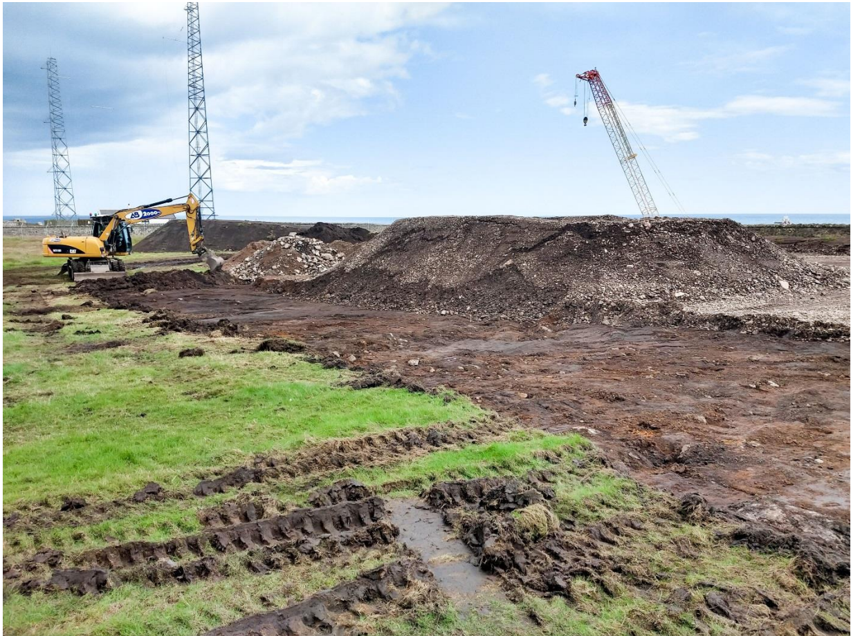
Illus 3 Soil strip along N side of watching brief area with DGPS radio tower aerials in background.
