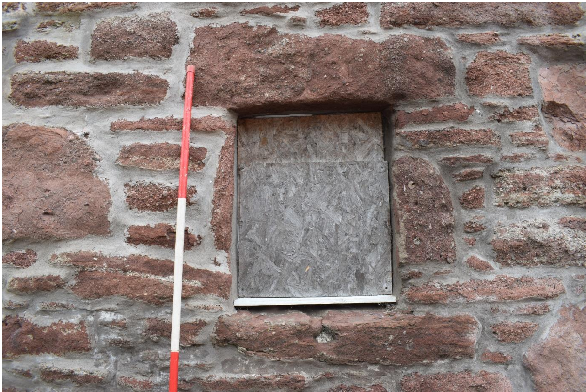
Illus 4 Window W3 showing red sandstone lintel, sill and jambs; facing SE
