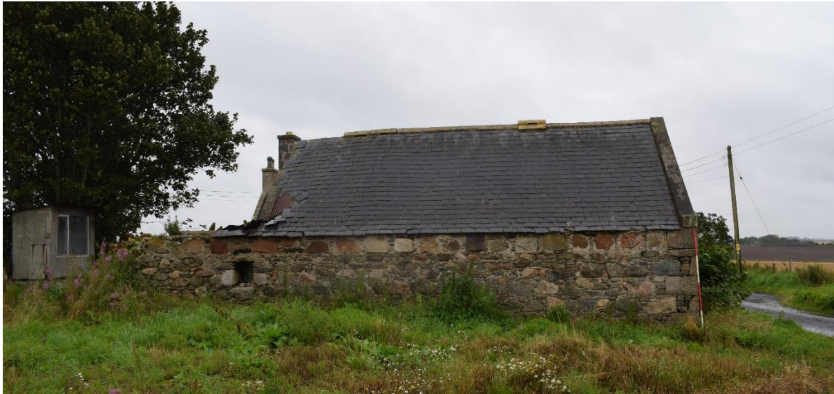
Illus 3 Building 1 NW wall; facing SE
