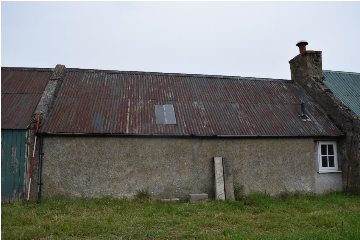
Illus 8 Building 2 ENE façade with D2 (right); facing WSW
