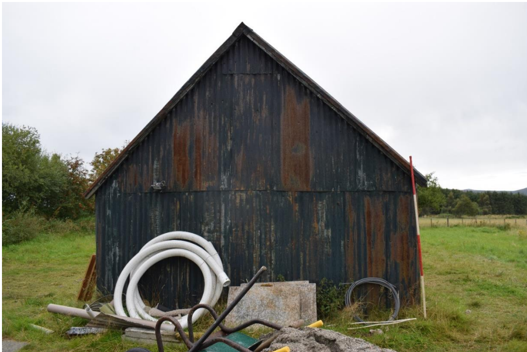
Illus 9 Building 3 SE gable, facing NNW
