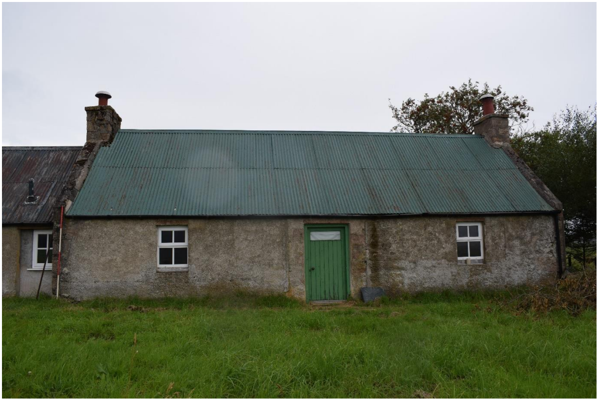
Illus 4 ENE front façade with W1, D3 and W2; facing WSW
