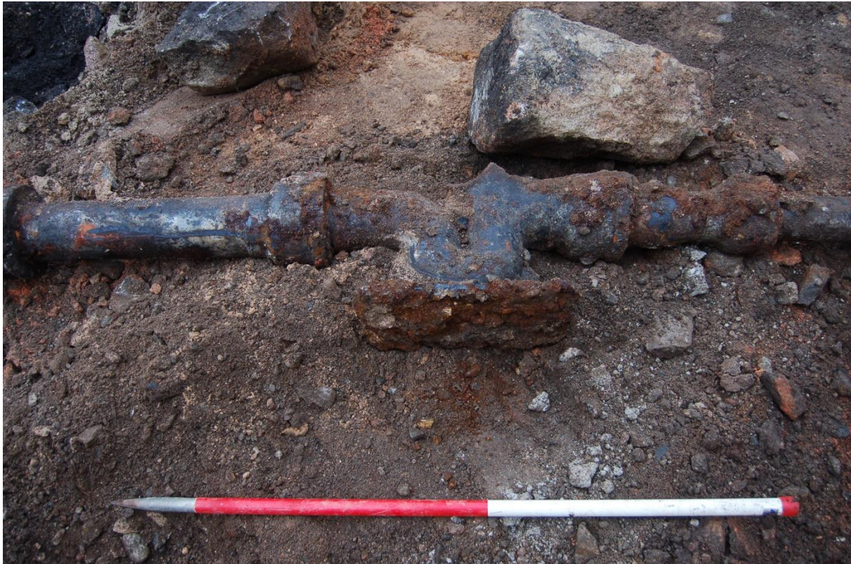
Illus 14 Section of cast iron sewer pipe with u-bend silt trap
