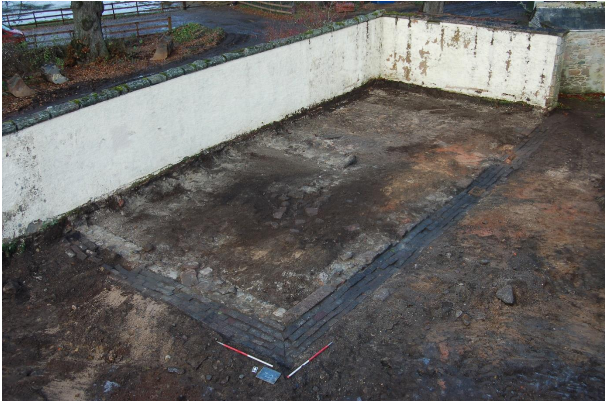
Illus 8 Outline of the building from above with the space between the NE perimeter wall and 1 visible (top right) as a darker band beyond the lighter yellow / grey of 1. The red/ orange patch of 9 can be seen middle right: facing N
