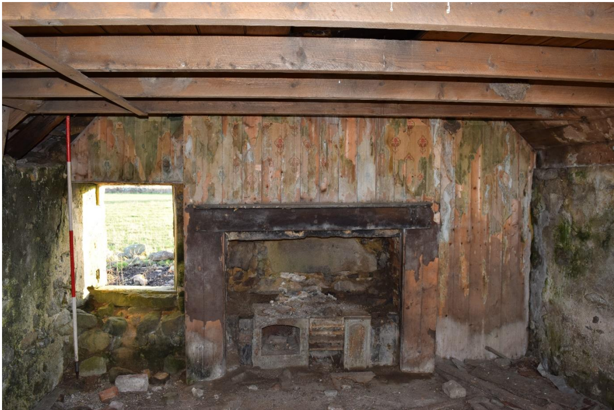
Illus 6 Building 1 Room 2 E wall range F2 on E wall with window W7 (left) showing wood paneling and wallpaper; facing E
