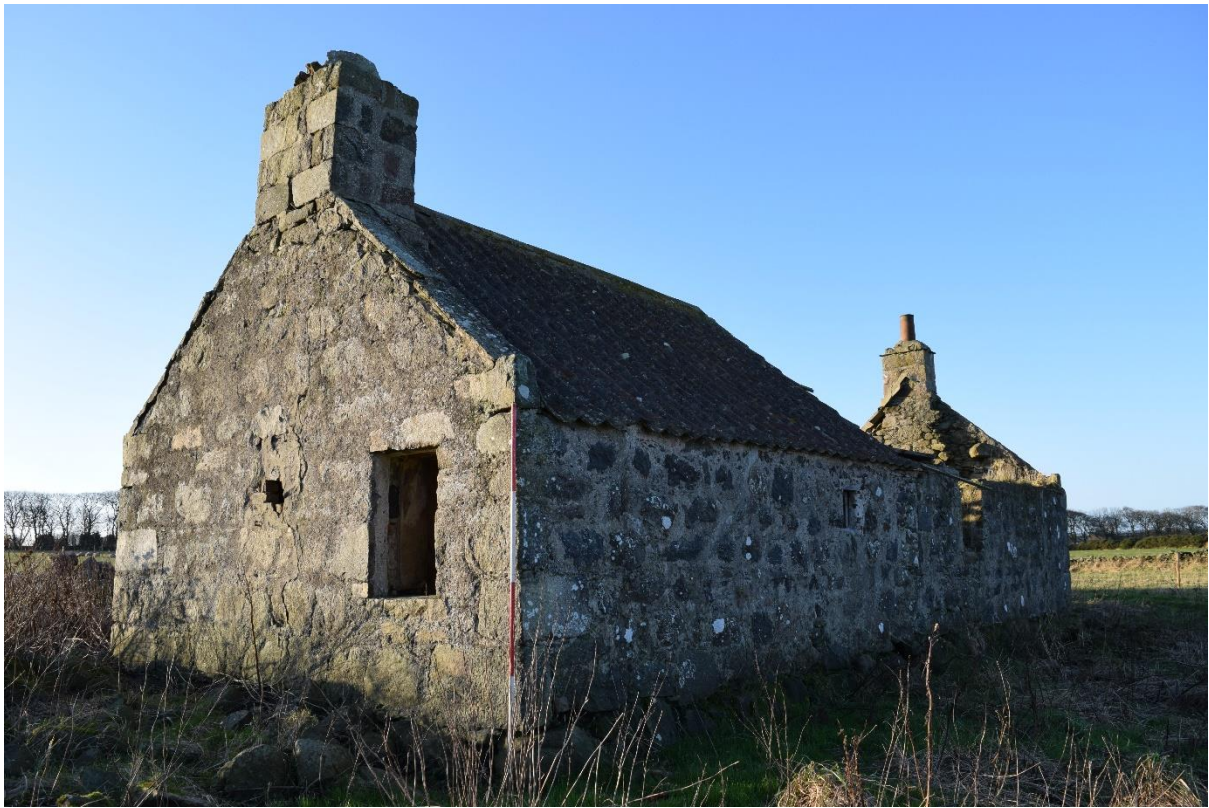
Illus 4 Building 1 E gable with W7 and N facade; facing SW
