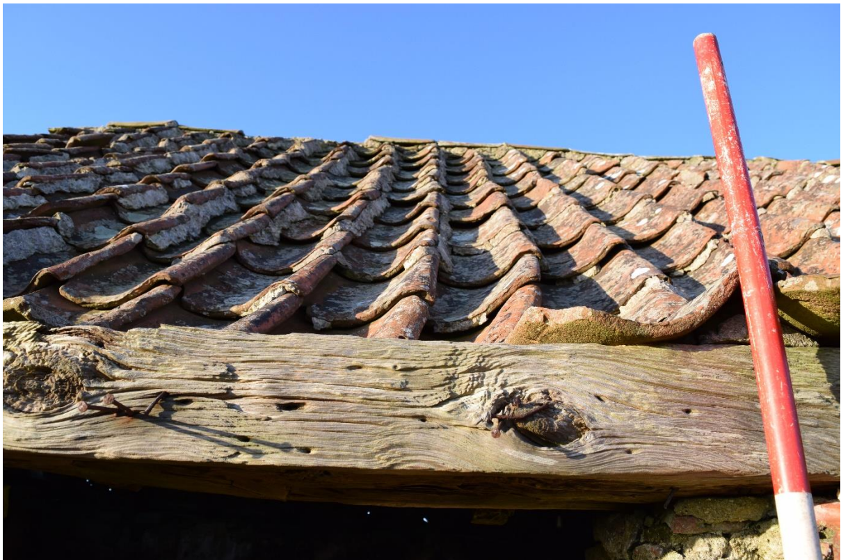
Illus 8 Pantile roof detail above D3; facing W
