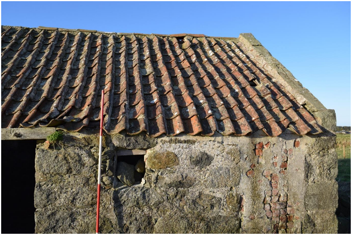
Illus 7 Pantile roof on Building 2 N end Room 1; facing W
