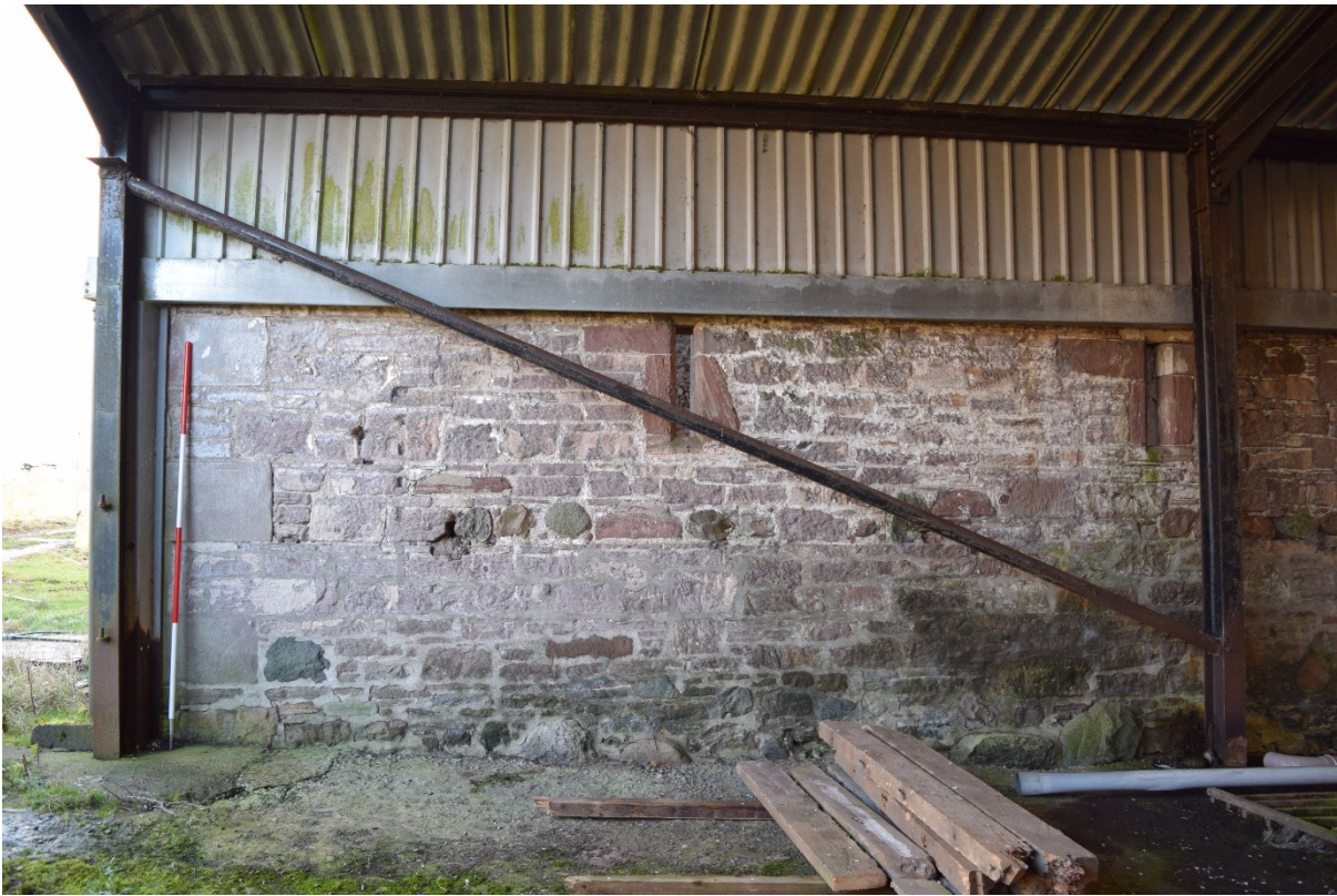
Illus 11 Room 9A SW wall exterior W35, W36; facing NE
