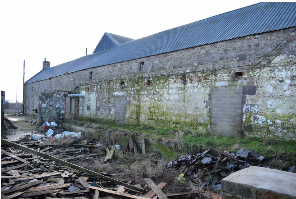
Illus 18 Room 9A NE wall with blocked doorways D5, D6 and upper windows W14, W15; wall scar F8 (right); facing S
