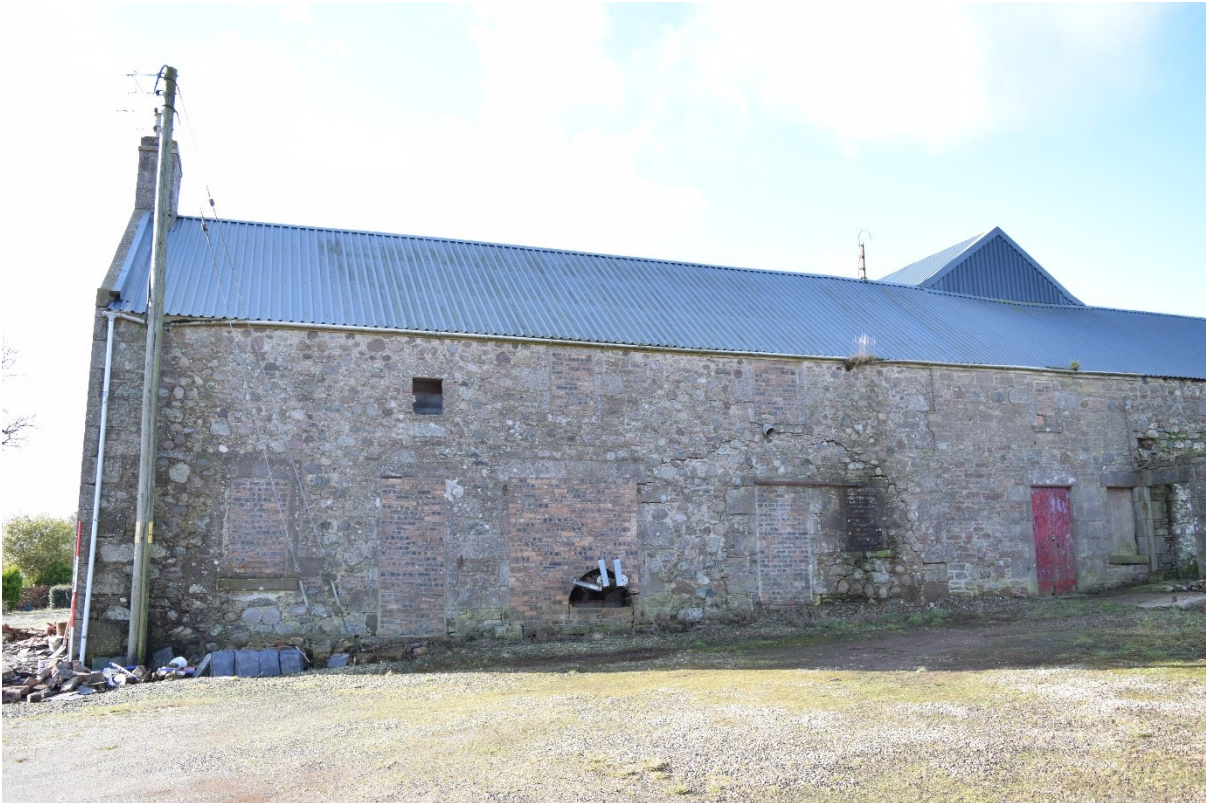
Illus 17 Rooms 10A and 10B NE wall with blocked doors and windows D1-3, W7-13
