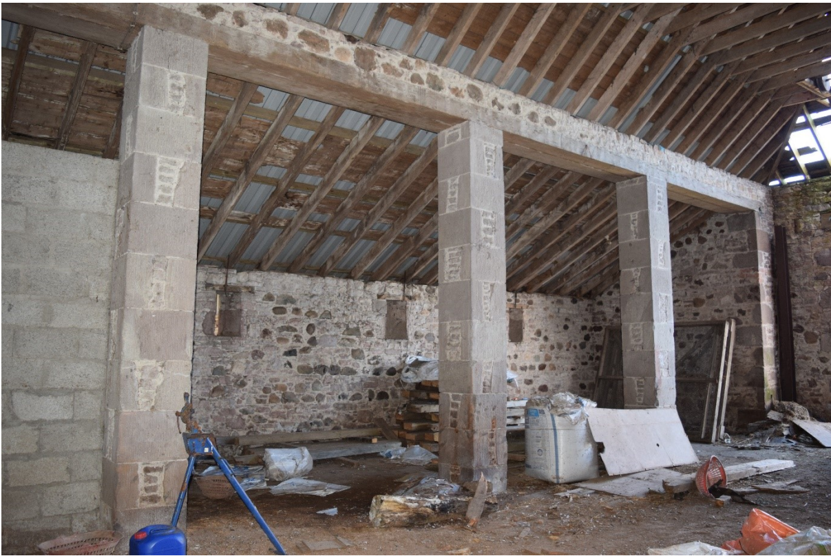
Illus 13 Sandstone piers between Room 9A (foreground) and 9B (background); facing WNW
