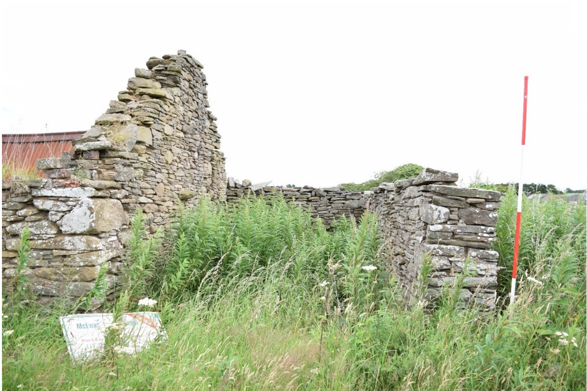
Illus 8 Room 4 SW wall; facing NE
