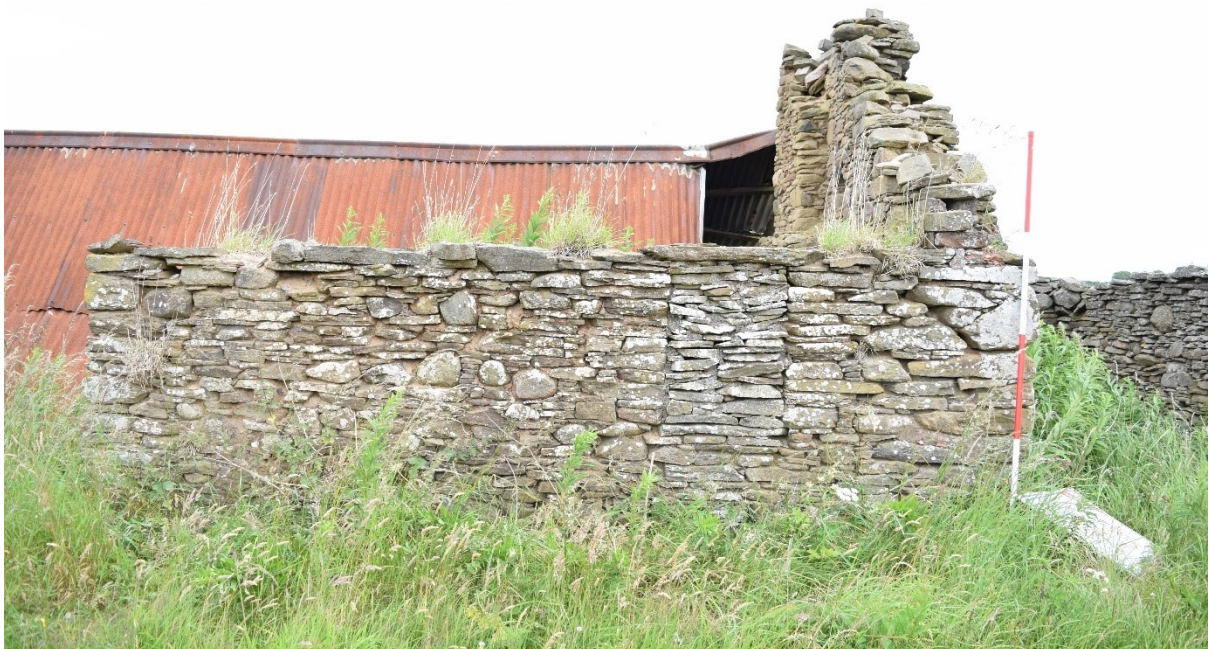
Illus 6 Room 3 SW wall blocked window W4; facing NE
