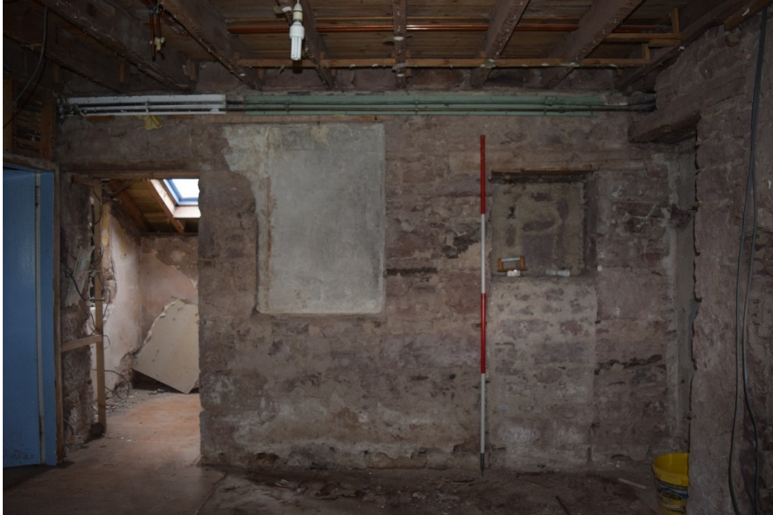
Illus 8 Phase 1 Room 1 NW wall with D3 (left), blocked window W3, door D2 later blocked to form window (right); facing NW
