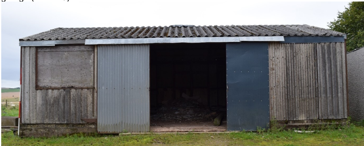
Illus 9 Building 2 NW façade; facing SE
