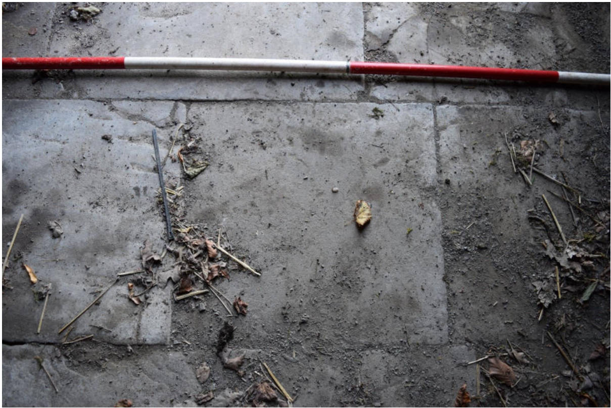
Illus 12 Stone slab floor of Room 2; facing SE
