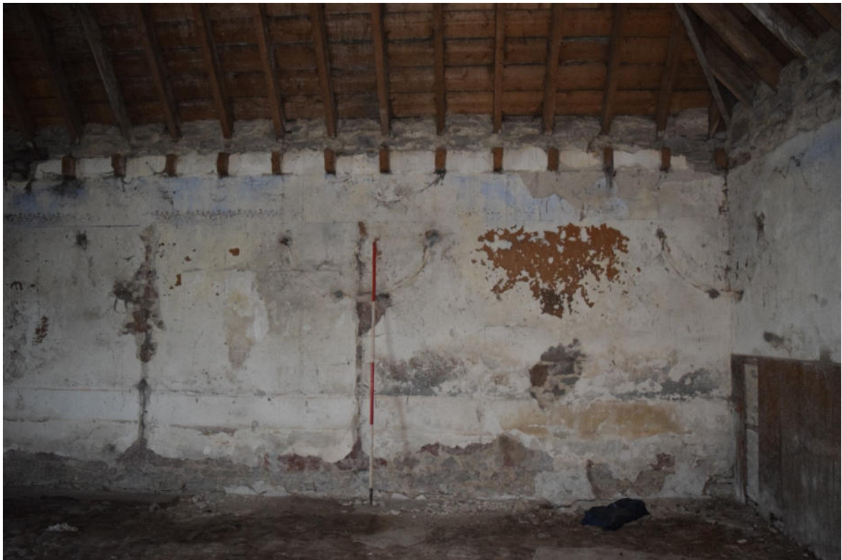
Illus 8 Room 1 SE wall scars from removal of stalls; facing SE
