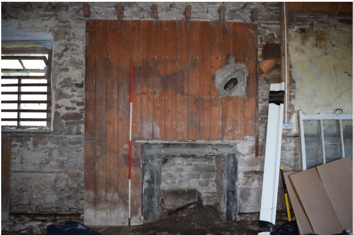
Illus 11 Room 2 SW wall W2 (left) fireplace F4 (centre) with wooden paneling
