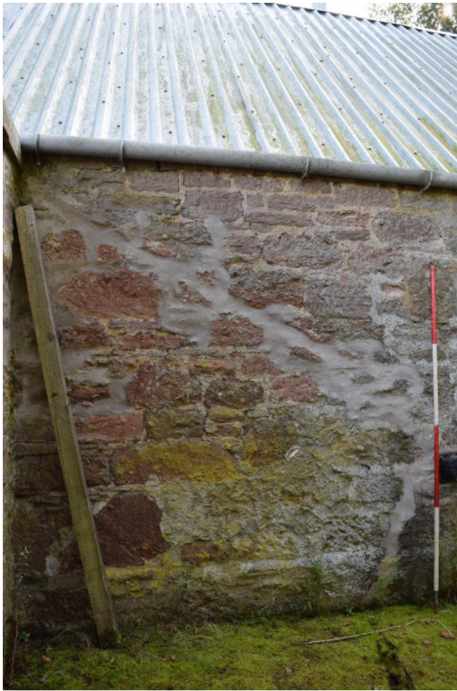
Illus 14 Elevation 3 scar after removal of Room 6 F16; facing SE
