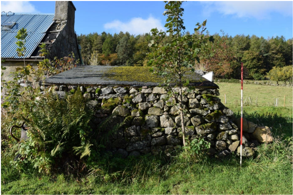
Illus 8 Room 5 E wall; facing W
