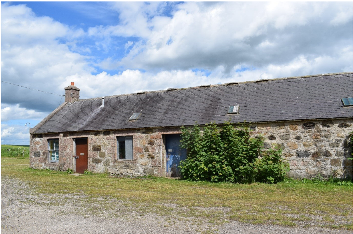
Illus 6 S façade Rooms 11 (left) and 12 (right); facing NW
