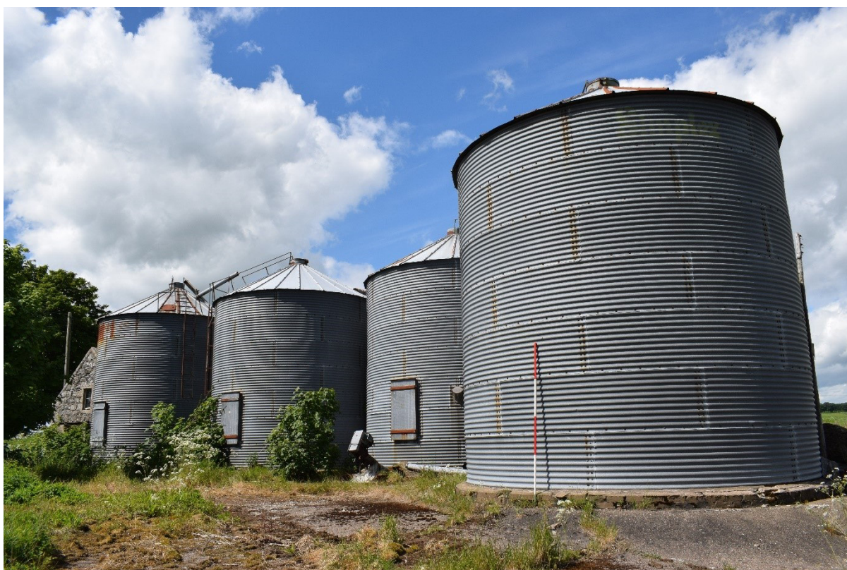
Illus 13 Tanks 2, 3, 4, 5 (l-r); facing SW
