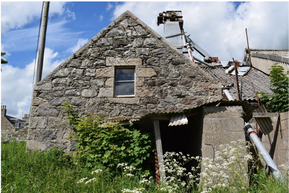
Illus 12 Room 4 E gable with W15 (top) and chute F3 (top right), overgrown and with unstable extension allowing little access; facing W
