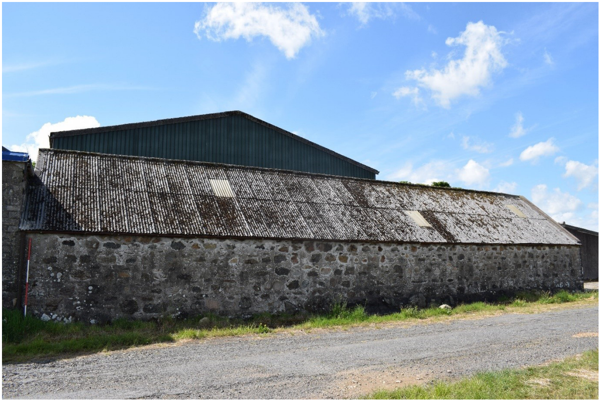
Illus 9 N wall Room 1; facing S
