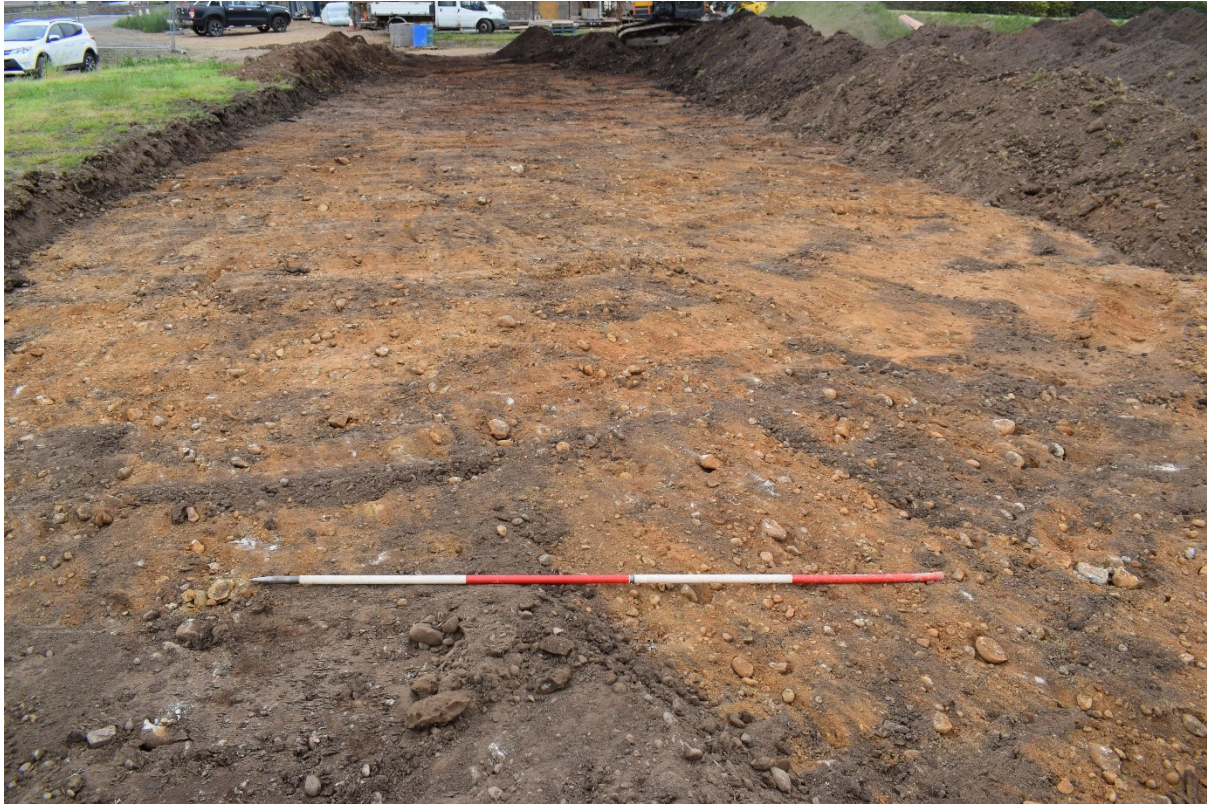
Illus 3 Monitored soil strip progressing; facing SE
