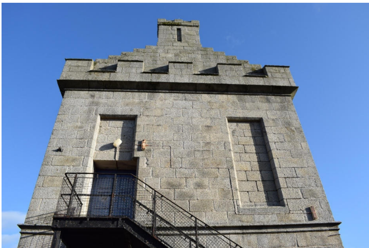
Illus 31 SW elevation showing W17 and W26 blocked with stone in Phase 2 and D5 opened in Phase 3 with iron stair F29; facing NE
