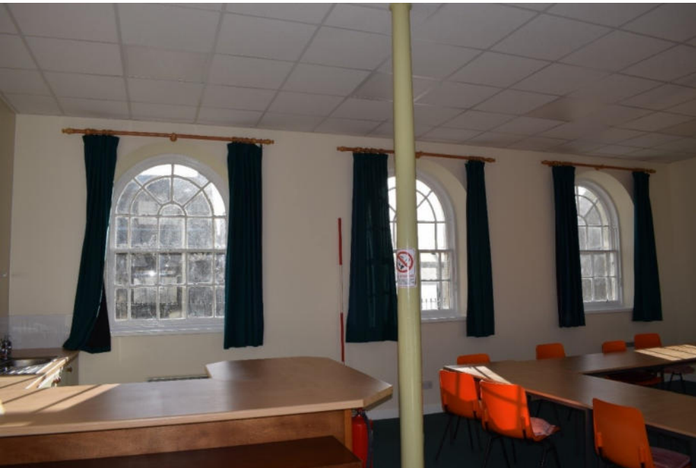
Illus 21 Room 1 SE wall W7, W6, W5; facing SE
