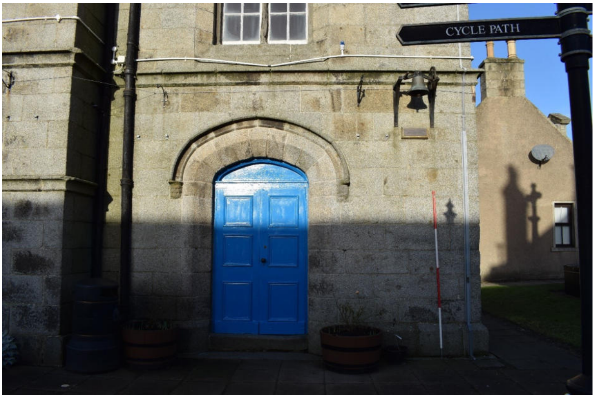
Illus 13 SE façade D3, hood moulding with sandstone heads F3 and F4 with W4 above and bell F23 (centre right); facing NW
