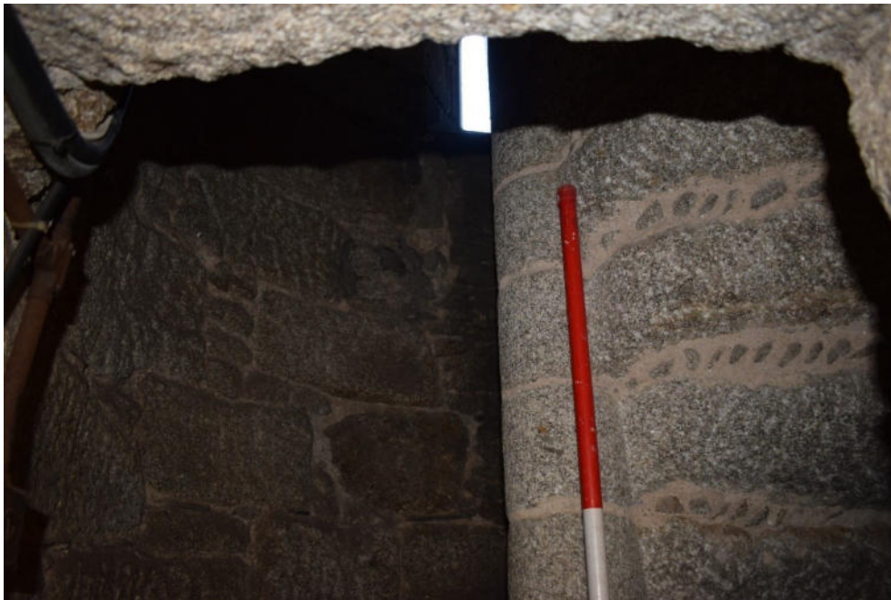
Illus 22 Stair F11; facing NW
