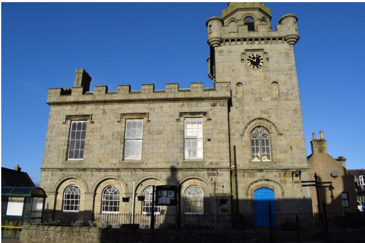
Illus 6 SE elevation; facing NW
