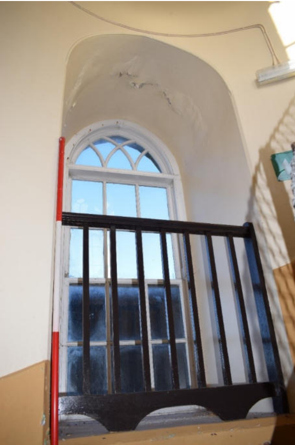
Illus 19 W9 on stair F10; facing NW
