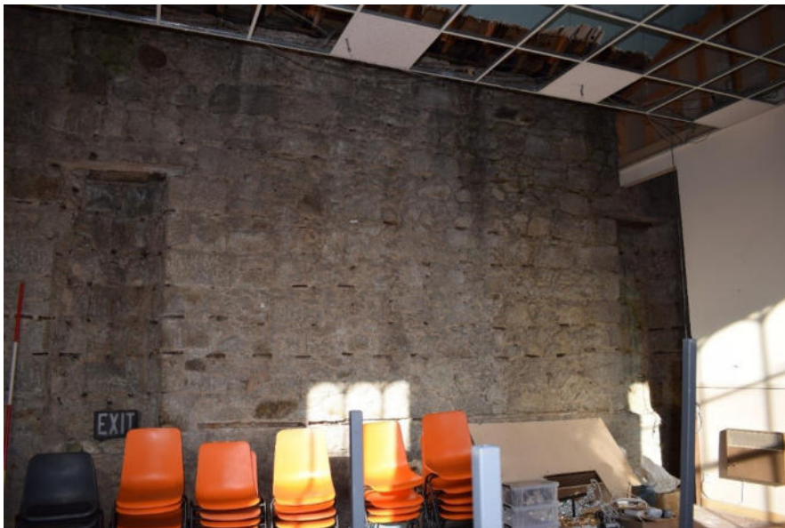
Illus 24 Room 5 NW wall F5 (left) F6 (right); facing NNW
