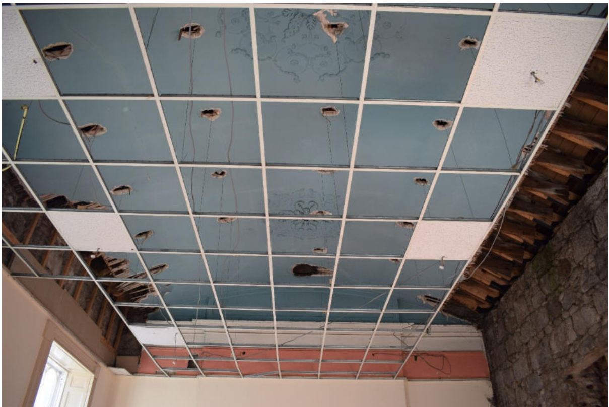
Illus 17 Room 5 plaster ceiling; facing SW
