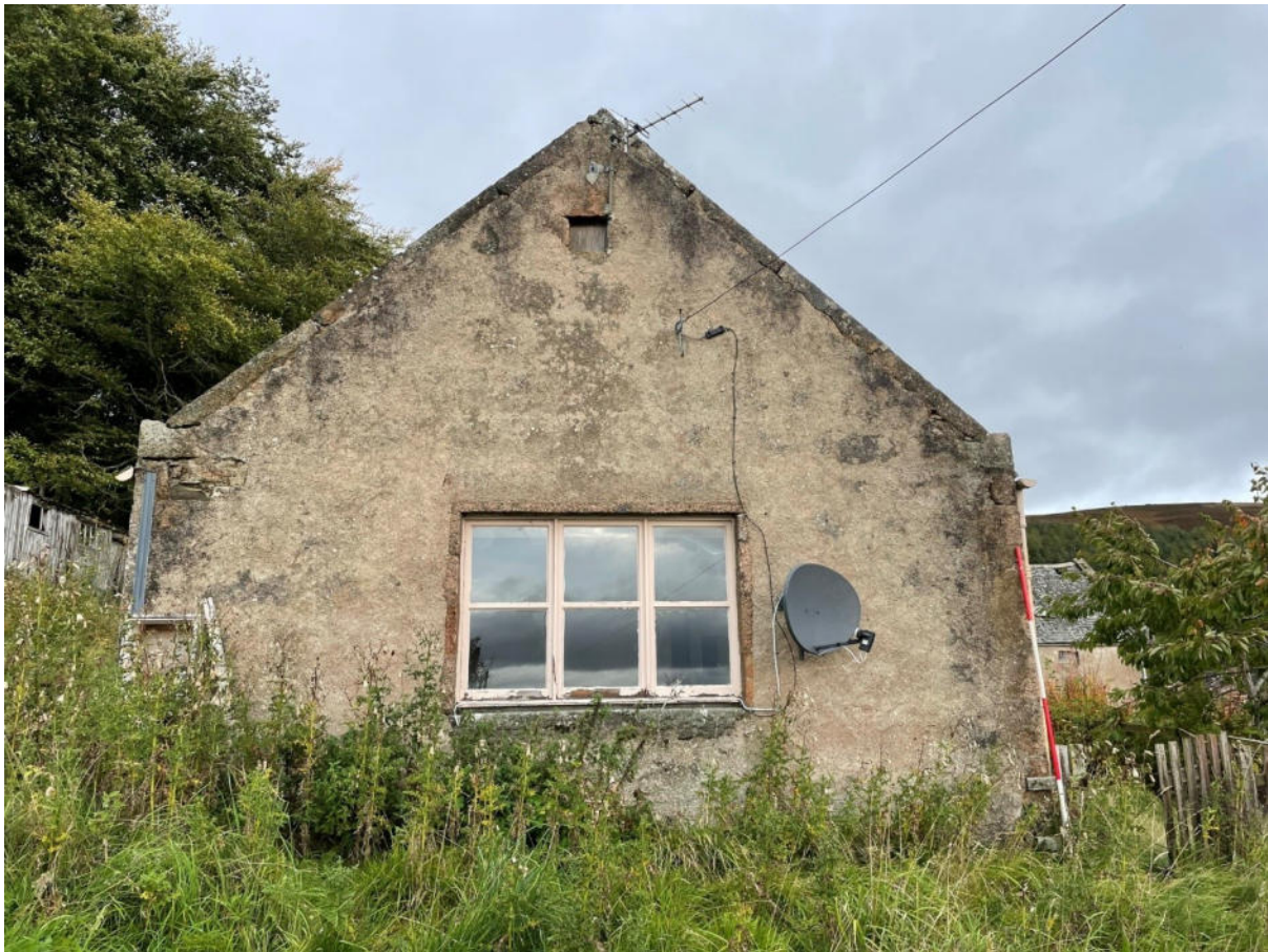
Illus 11 Room 6 S wall W14 (below) W15 (above); facing N
