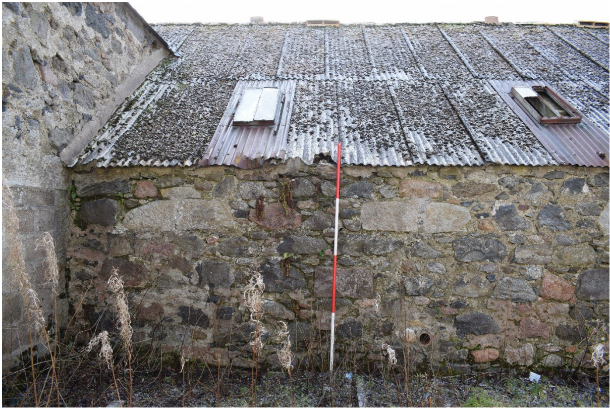
Illus 14 Room 4 blocked windows W13 (left) and W14 (right); facing SSE
