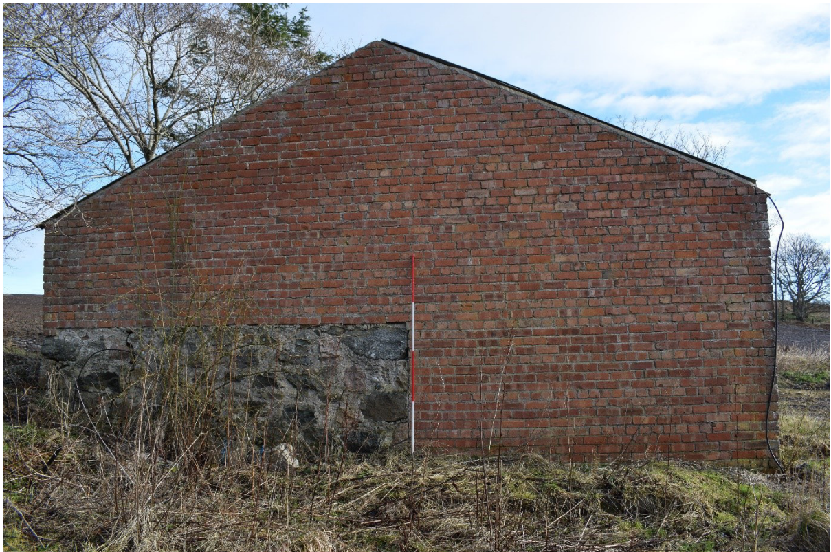
Illus 31 Building 2 WSW wall with Phase 1 stone wall; facing ENE
