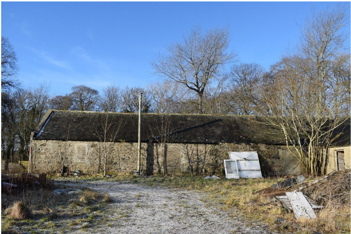
Illus 7 Courtyard WSW wing ENE elevation showing stone rubble construction and breeze block filled apertures; facing ENE
