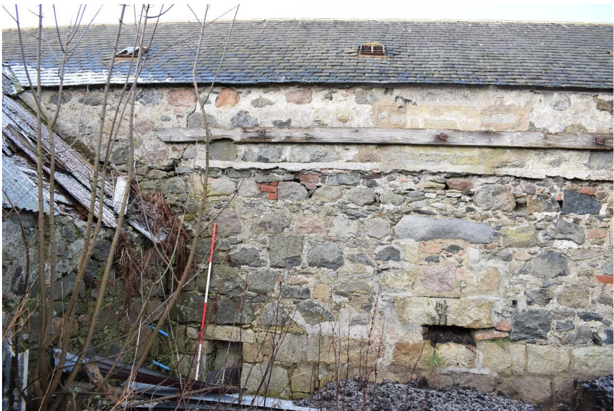
Illus 11 Room 5 ENE wall aperture F9 (bottom left), F11 (centre) with concrete roof scar F15 (centre); facing WSW
