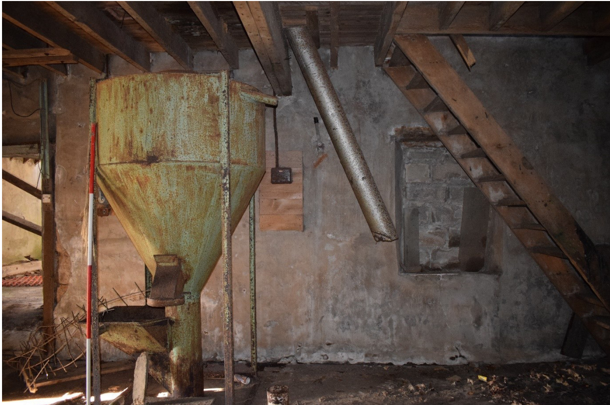
Illus 25 Room 5 metal hopper F5 with wooden stair F6; facing WSW
