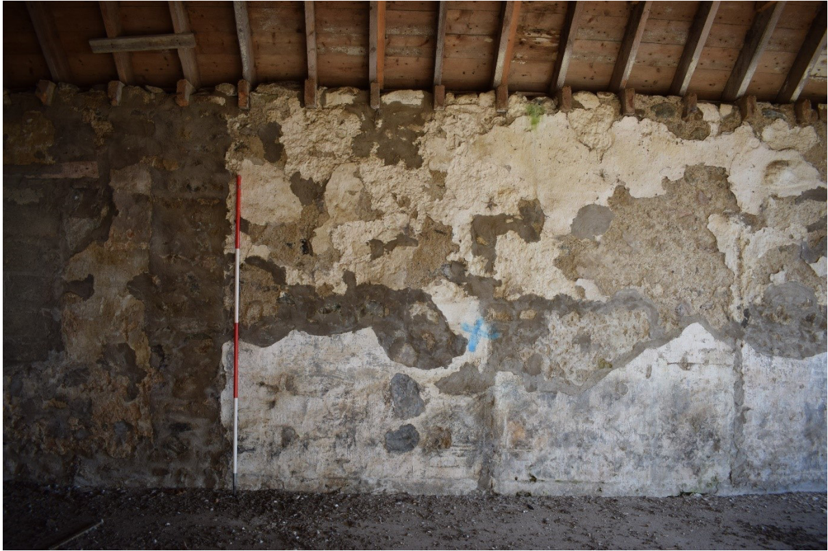
Illus 21 Room 7 ENE wall with scars of stalls (F8); facing ENE
