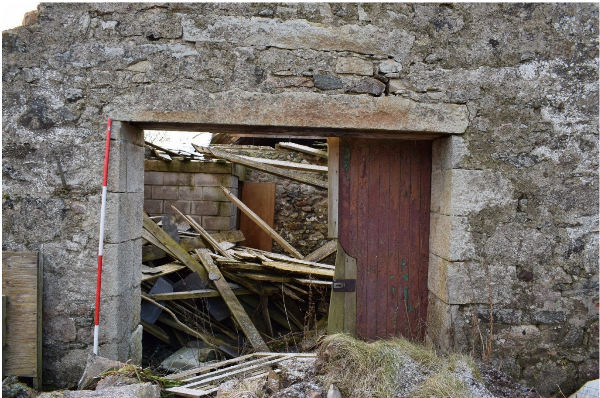
Illus 9 Room 6 NNW wall D12 with W35 sill above; facing SSE
